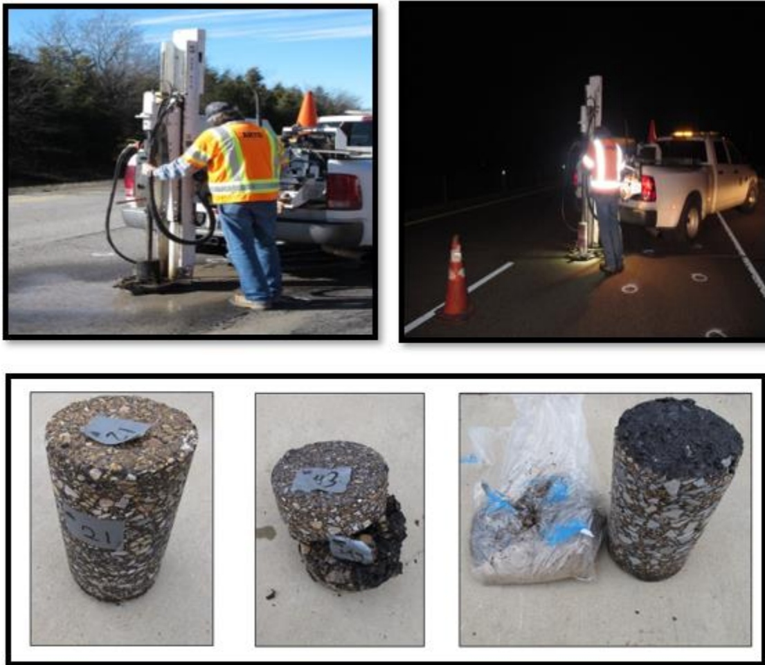
Figure 12. Collection of RAP coarse from the existing pavement
