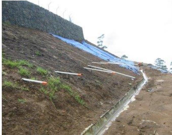
Figure 6. Horizontal Drains Protruding from Slope (www.geonusa.com)
