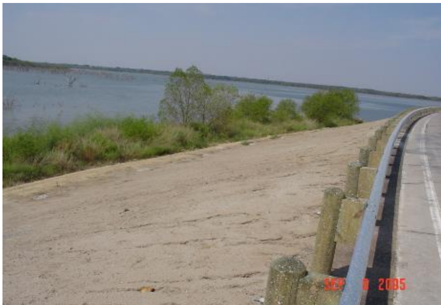
Figure 29. Down-Slope View of Completed FRS Embankment Prior to Grass Establishment - Lake Ridge Parkway (Gregory 2006)
