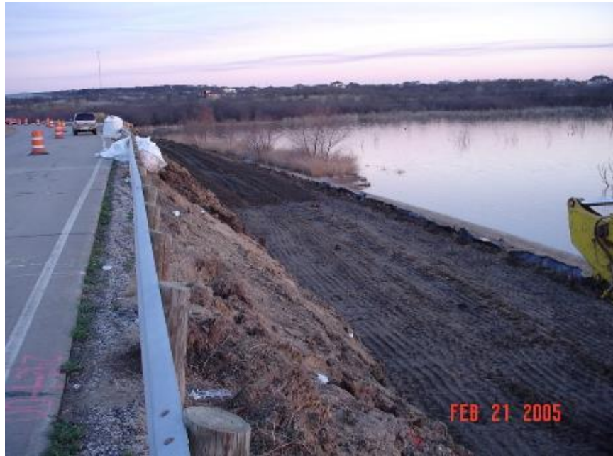
Figure 28. View of FRS Being Installed In Lifts - Lake Ridge Parkway (Gregory 2006)
