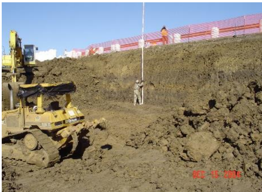
Figure 27. Initial Excavation for FRS Slope Repair - Lake Ridge Parkway (Gregory 2006)
