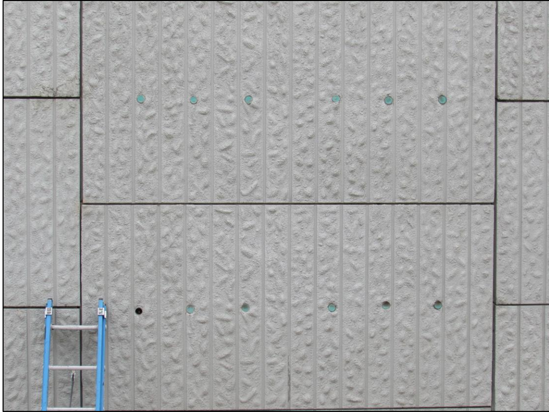
Figure 3-1: Typical MSE Wall Panels with Test Coupons
