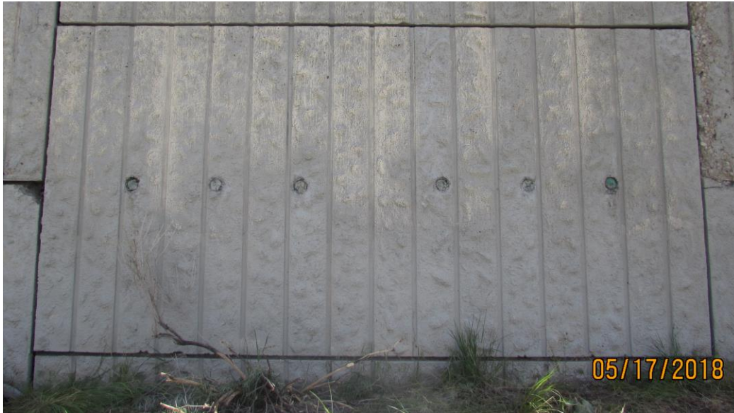
Figure 1-2: MSE Wall Panel with Coupons
