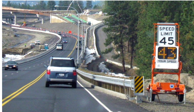
Figure 10. Photo. Rural construction zone.
