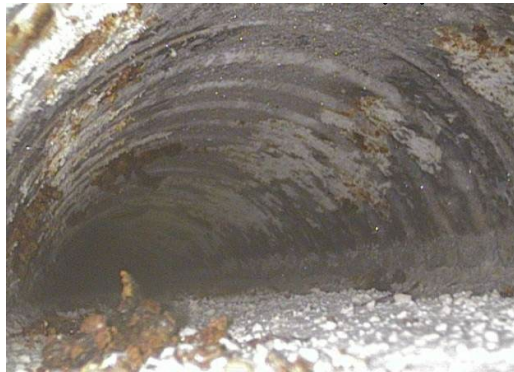
A. Corroded duct interior.
