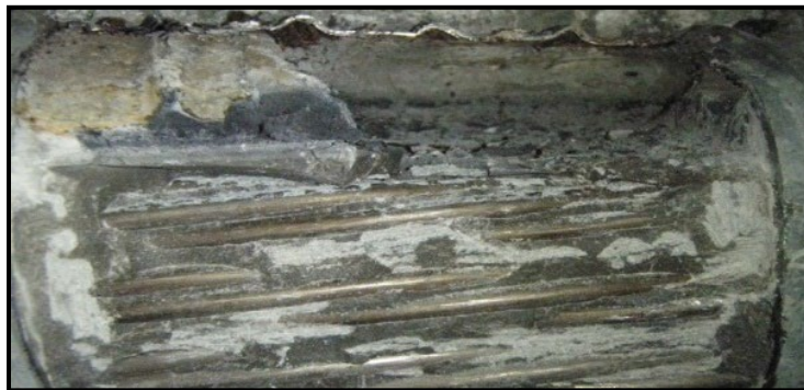
D. Exposed tendon condition 4.
