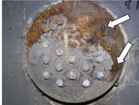
Figure 29. Photo. Exposed anchorage zone after a grout cap was removed.
