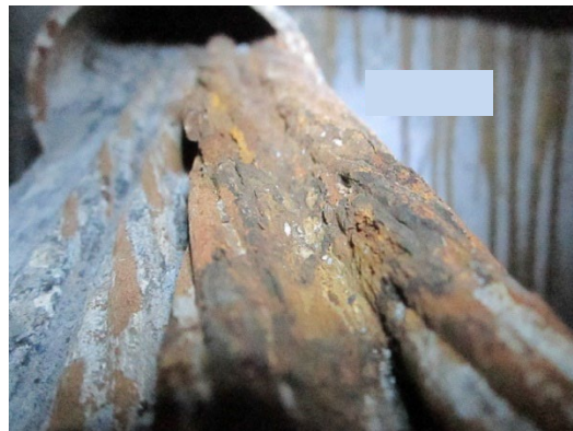
Figure 27. Photo. Closeup of severely corroded strands in a rejected tendon. (49)
