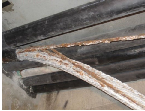
© 2017 Seoul City Facility Management.
