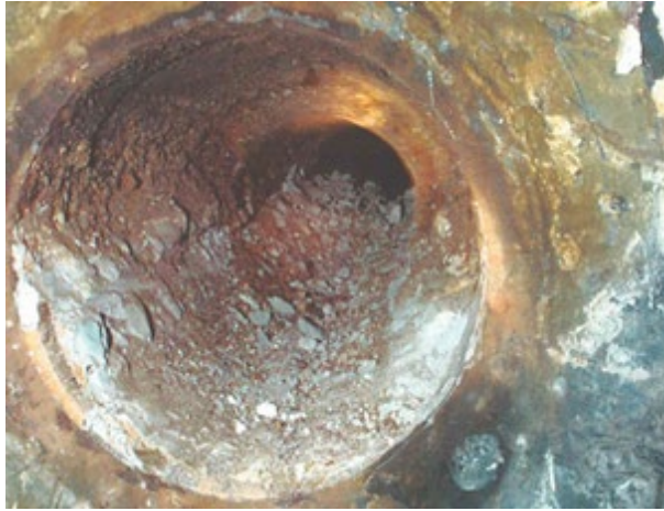
B. Interior of anchorage trumpet.
