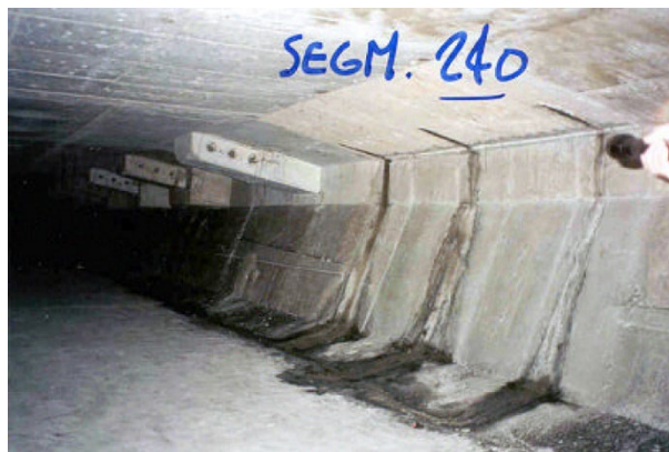
Figure 39. Photo. Interior view of water-leaking box girders at the Sawgrass Interchange. (17)
