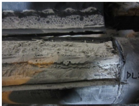
© 2017 Seoul City Facility Management.
