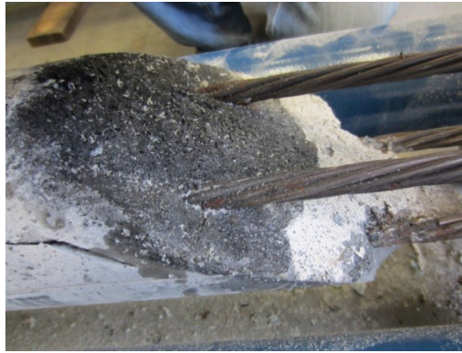
A. Strands at grout/void interface.
