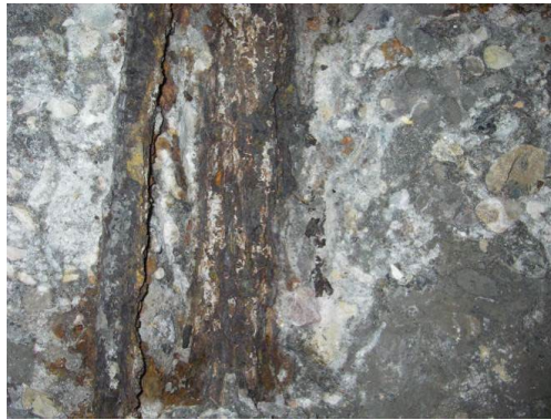
B. Closeup of a corroded tendon.
