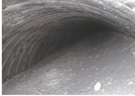
B. Corrosion-free duct interior.
