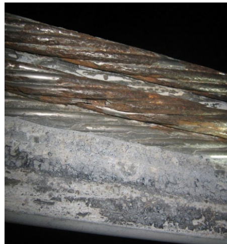
Figure 25. Photo. Closeup of segregated grout in a half-filled tendon.
