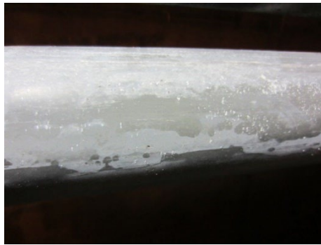
© 2017 Seoul City Facility Management.
