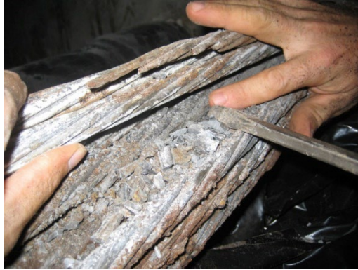
Figure 24. Photo. Interior condition of strands filled with chalky grout.
