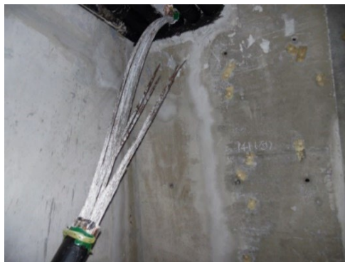
© 2017 Seoul City Facility Management.
