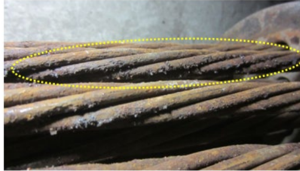
© 2017 Seoul City Facility Management.
