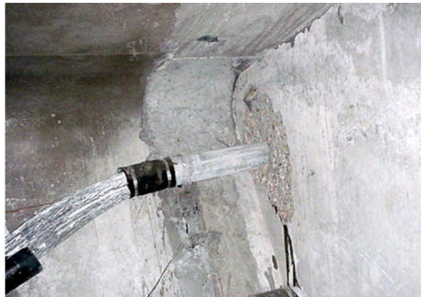
Figure 2. Photo. Failed tendon in the Mid-Bay Bridge. (17)
