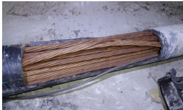
© 2017 Seoul City Facility Management.
