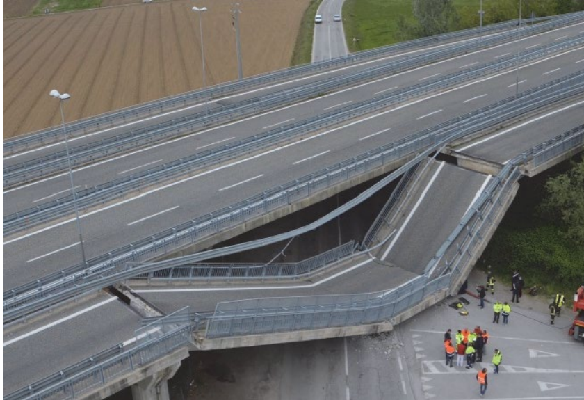
Figure 52. Photo. Collapsed La Reale Viaduct ramp. (81)
