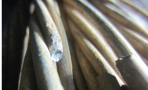
© 2017 Seoul City Facility Management.
