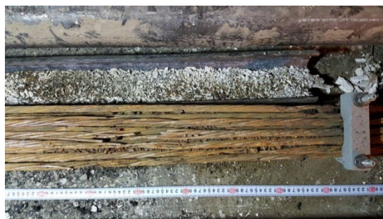
© 2017 Seoul City Facility Management.
