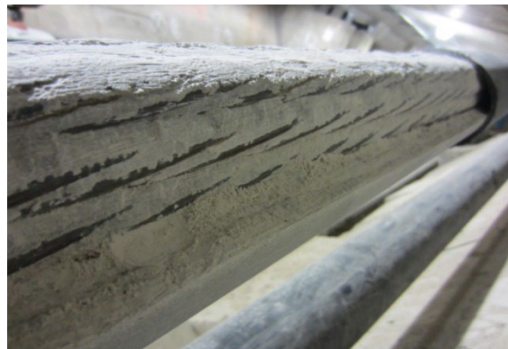
Figure 13. Photo. Typical condition of the segregated grout.
