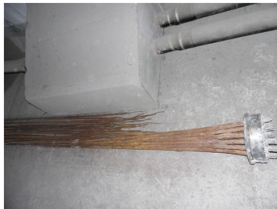
© 2017 Seoul City Facility Management.
