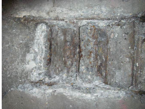
A. Corroded tendons exposed.
