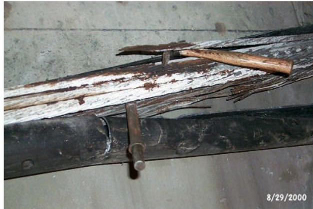
Figure 3. Photo. Severely damaged tendon. (17)
