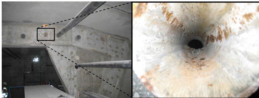
A. Closeup of the other end of the ruptured tendon.
