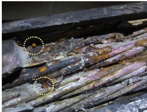
© 2017 Seoul City Facility Management.
