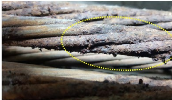
© 2017 Seoul City Facility Management.
