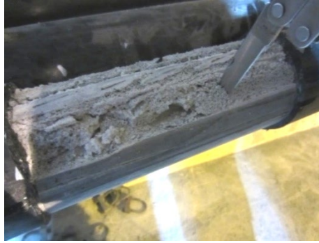
© 2017 Seoul City Facility Management.
