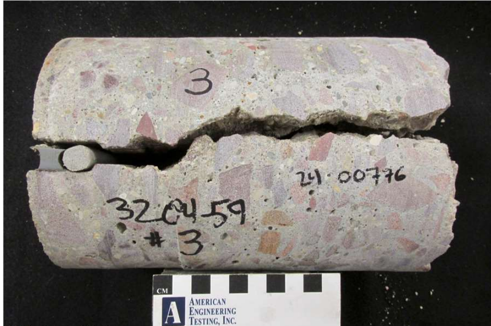
DESCRIPTION – Project 3204-59, core
