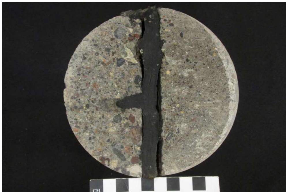
DESCRIPTION – Project 2786-116, core 1J, as-received
