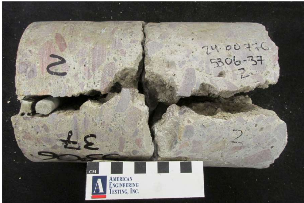
DESCRIPTION – Project 5306-37, core 2
