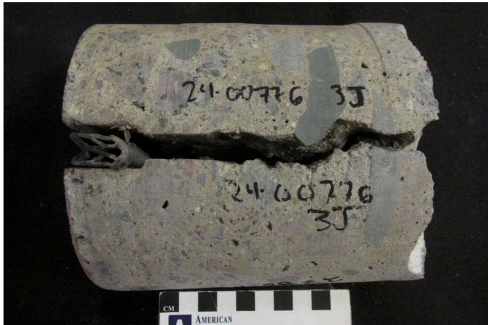
DESCRIPTION – Project 2786-115, core 3J, as-received
