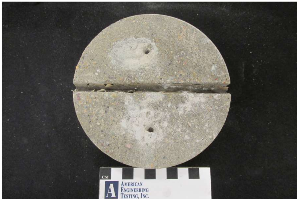
DESCRIPTION – Project 0712-32, Core 2
