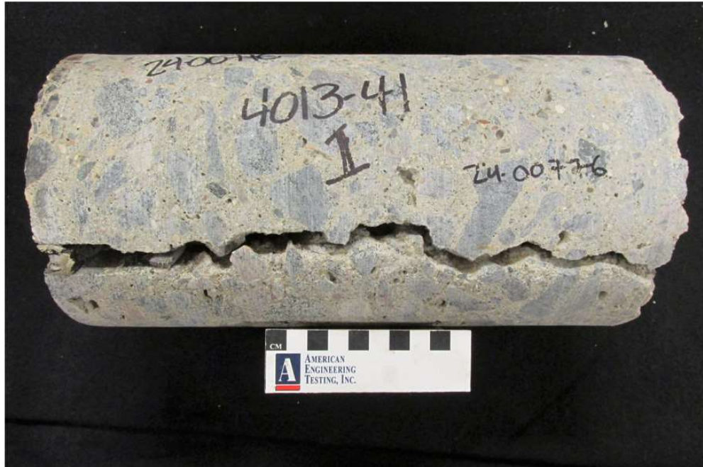
DESCRIPTION – Project 4013-41, core 1
