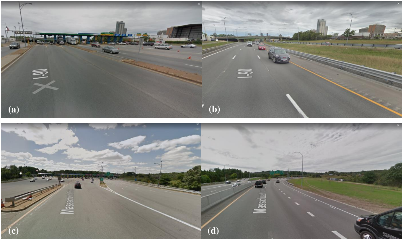
Figure 2. Images of the Massachusetts Turnpike before and after legacy toll plazas were demolished in (a) before: Allston/July 2011, (b) after: Allston/September 2018, (c) before: Weston/August 2013, and (d) after: Weston/September 2018 (Source: Google Maps)
