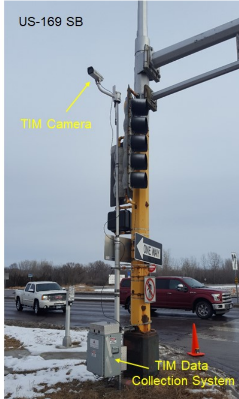
Figure 3.7 Installation of Video Data Collection System at US-169 & TH-282/Quaker Ave.
