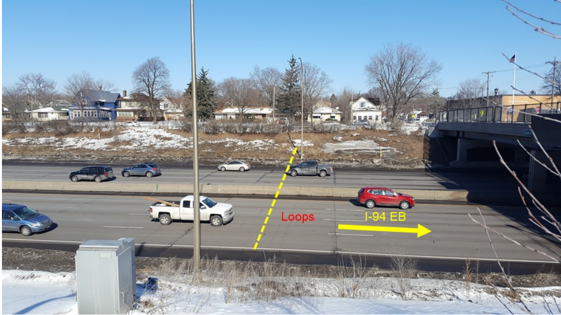
Figure 3.17 Location of Inductive Loop Sensors at Site #5 (I-94 at N Victoria St).
