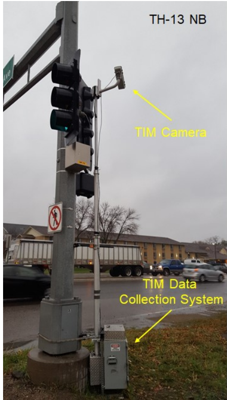
Figure 3.11 Installation of Video Data Collection System at Site #3 (TH-13 at Lynn Ave).
