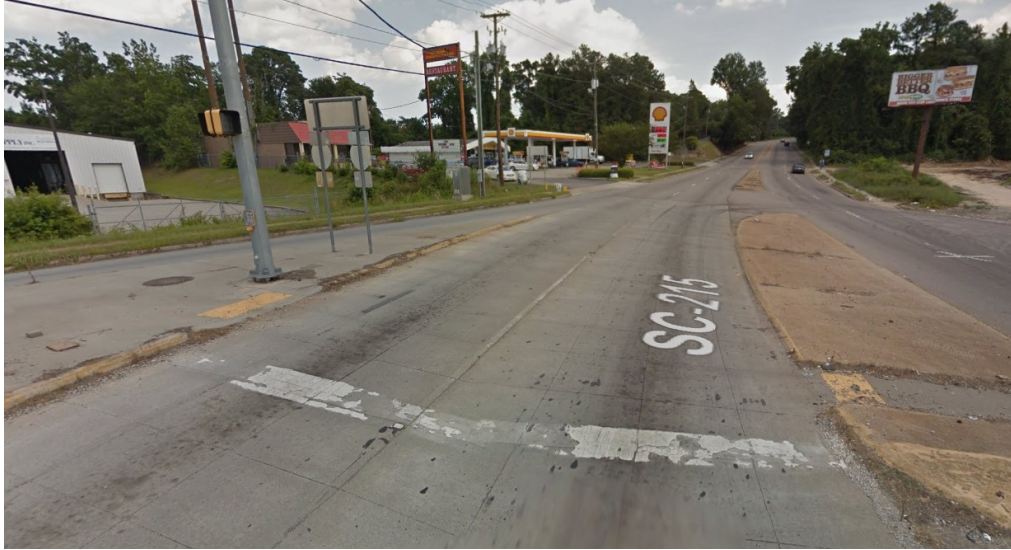
Figure 3-7. FRC overlay on SC-215 near Columbia, SC (Google Maps, 2016).
