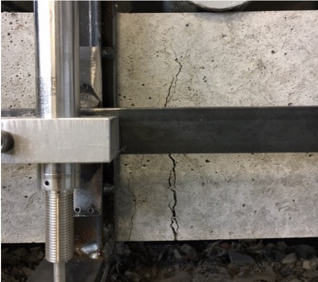
Figure 4-13. An example of a crack developed after peak load was achieved in a flexural performance test.
