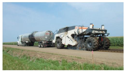
A train of equipment runs on an SFDR site: a tanker of new asphaltic material connected to a reclaimer that pulverizes the old pavement and mixes in part of the road base and possibly stabilizing agents.
