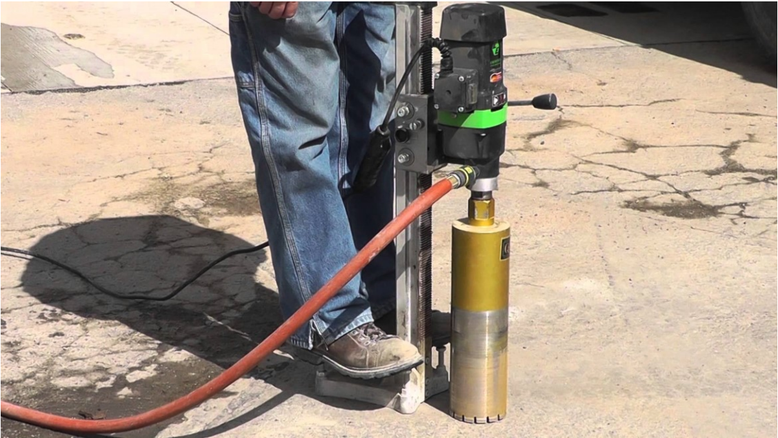
Figure 5. Pavement coring apparatus.
