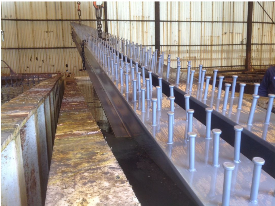
Figure 2 Steel Beams Progressively Dipped in Kettle Filled with Molten Zinc
