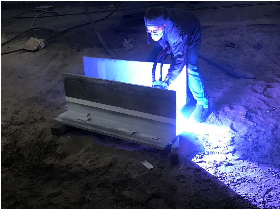
Figure 19 Metallizing T-Beams (Note Removal of Masking)
