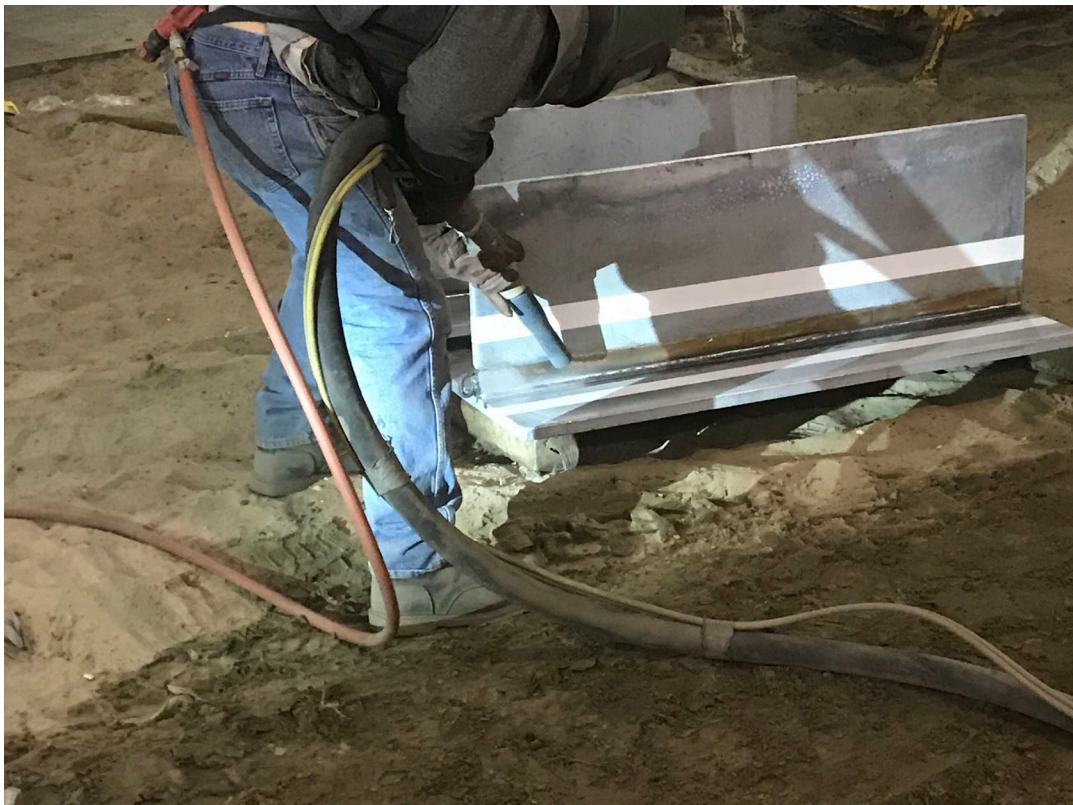
Figure 15 Abrasive Blasting Fillet Welds
