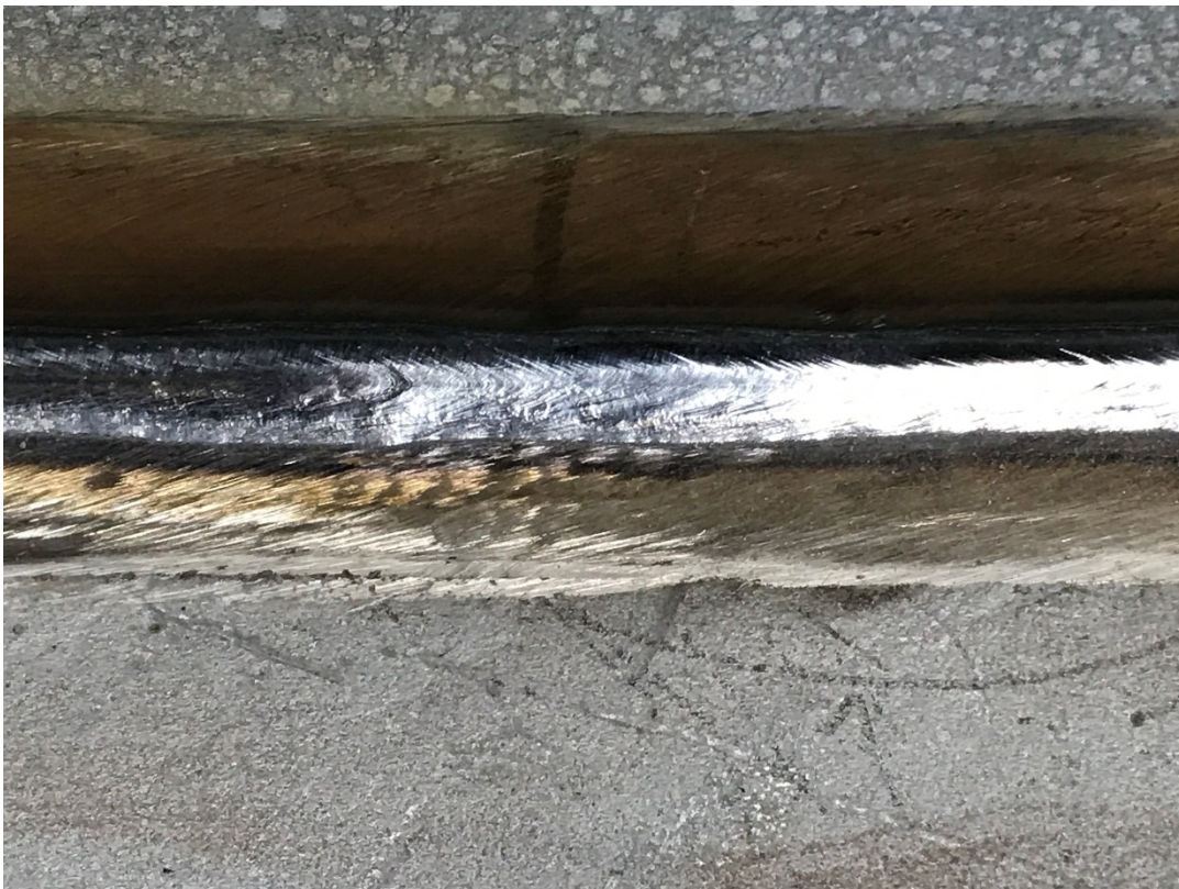
Figure 13 Completed 5/16" Fillet Weld
