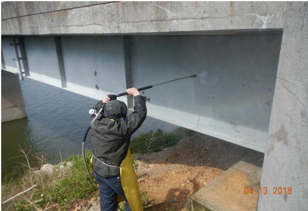
Figure 23 KTC Personnel Pressure Washing Beam Ends
