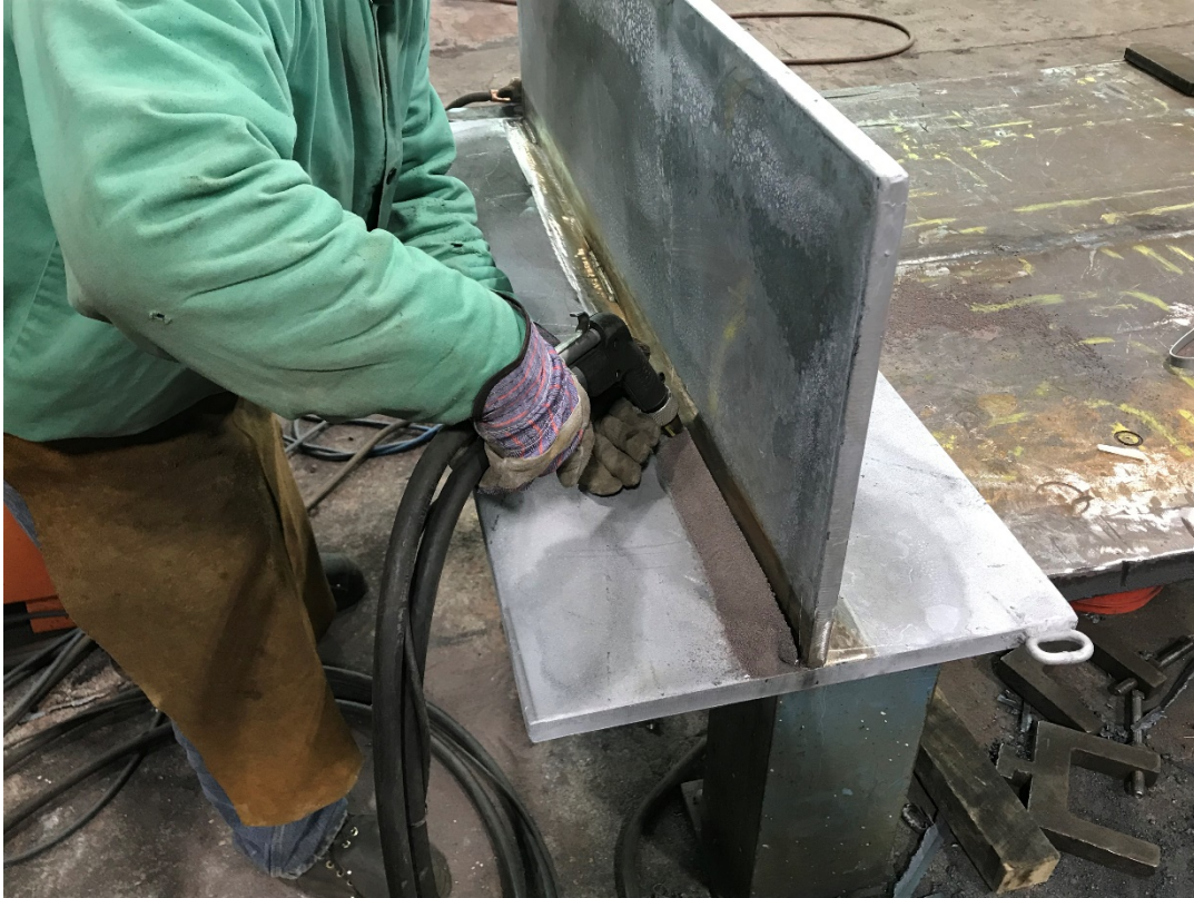
Figure 12 Manual Sub-Arc Fillet Weld
