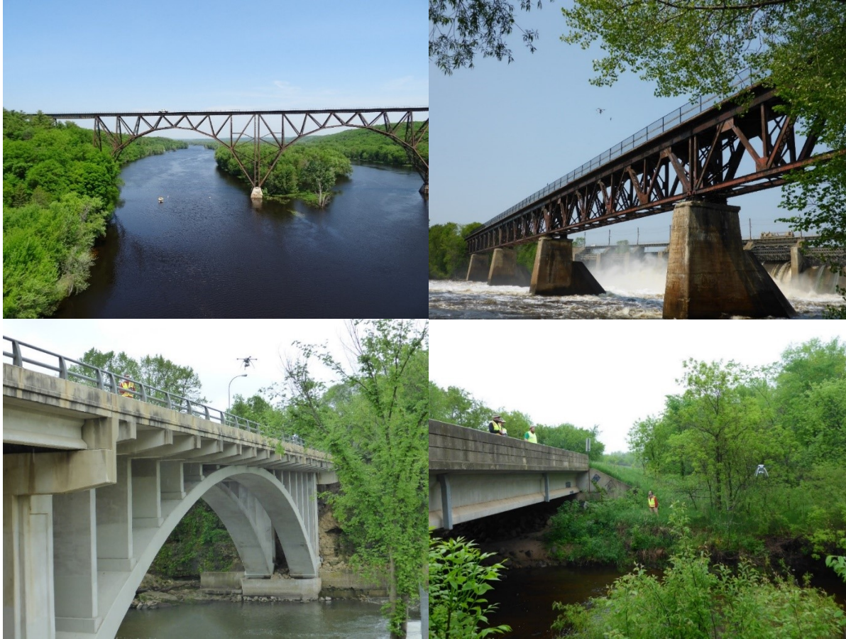
Figure 1.1 Overall Photographs of Four Bridges Selected for Phase I UAS Inspection.
