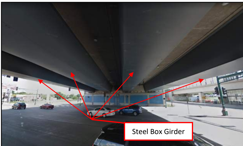
Image 3: Overall View of Bridge Underside.
