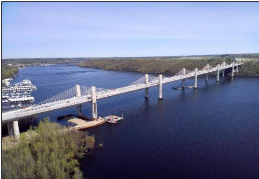
Image 2: Overall View of Bridge.
