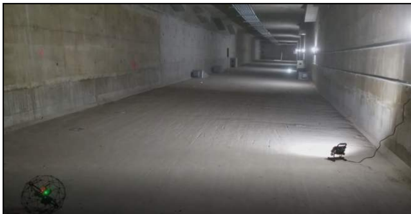
Image 3: Overall View of Inside of a Box Girder.
