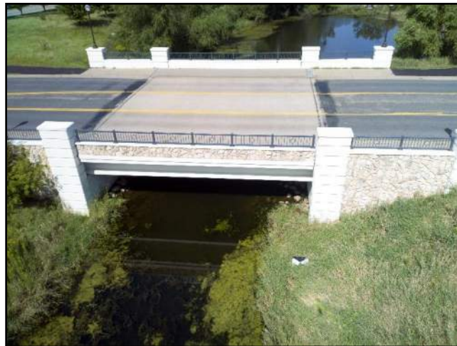
Image 2: Overall View of Bridge Topside.
