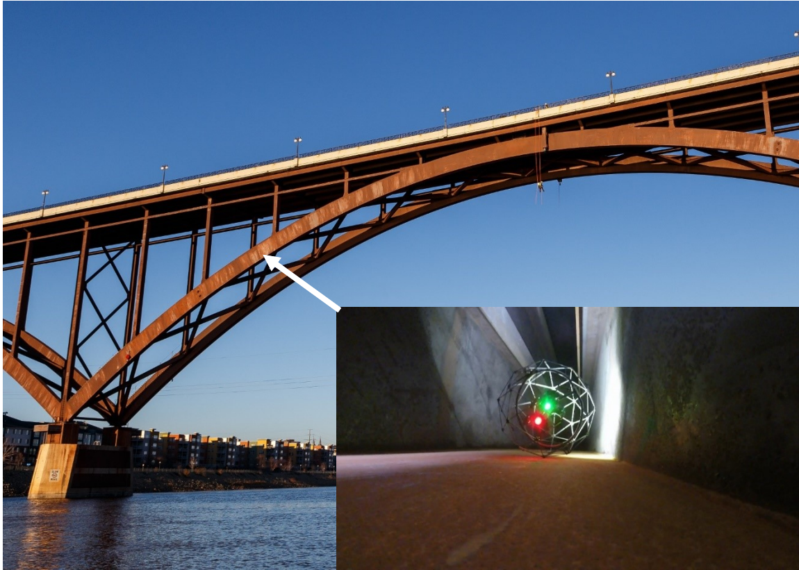
Figure 3.9 Photograph of the Elios UAS Rolling Inside a Steel Box Beam
