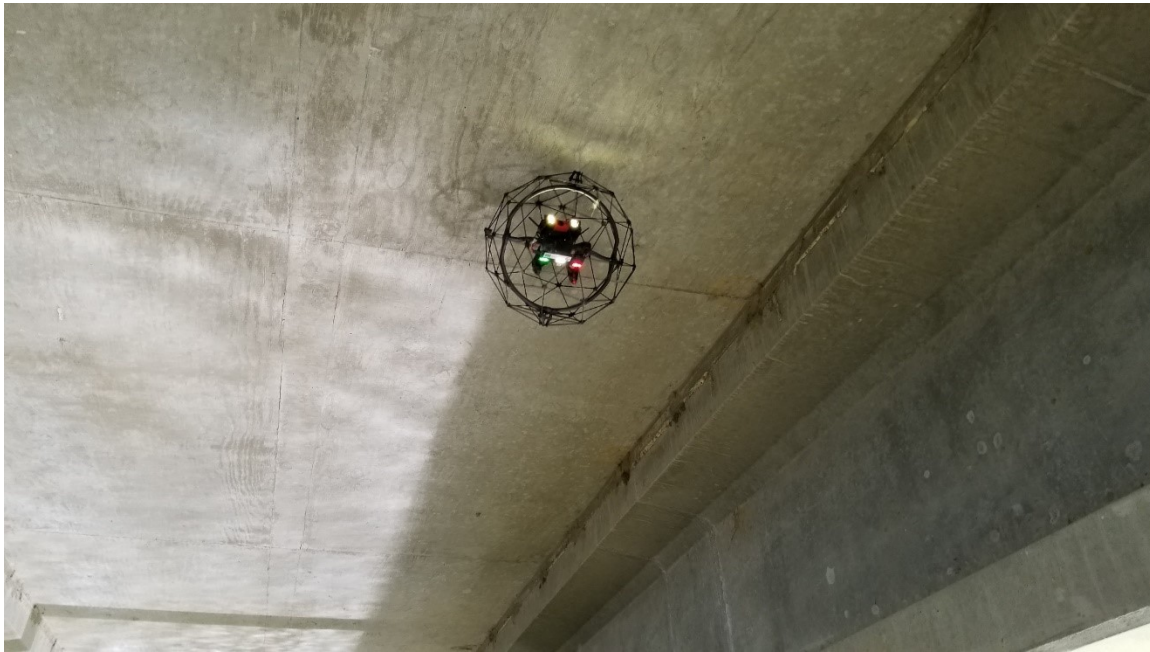
Figure 3.8 Photograph of the Elios UAS Rolling along a Concrete Deck Soffit.
