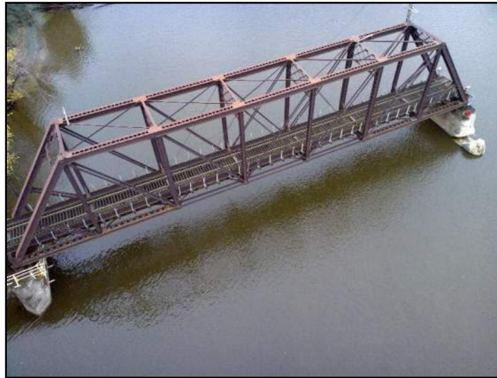
Image 2: Overall View of Bridge Topside.
