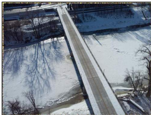
Image 3: Overall View of Bridge Topside.
