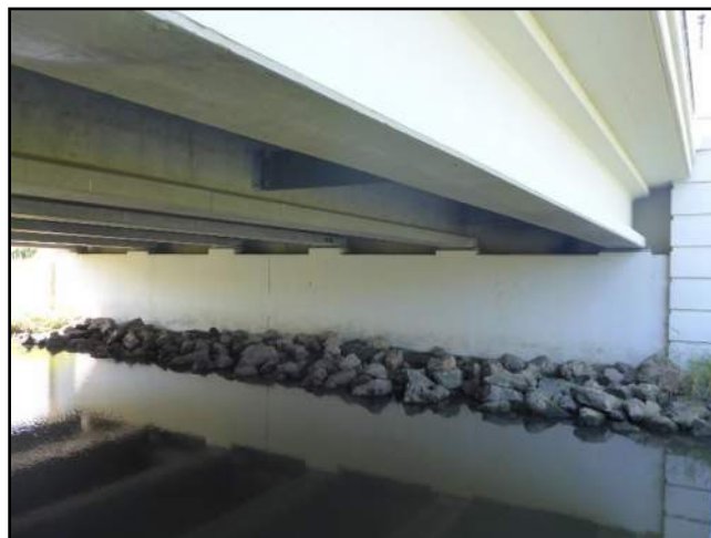
Image 3: Overall View of Bridge Underside.
