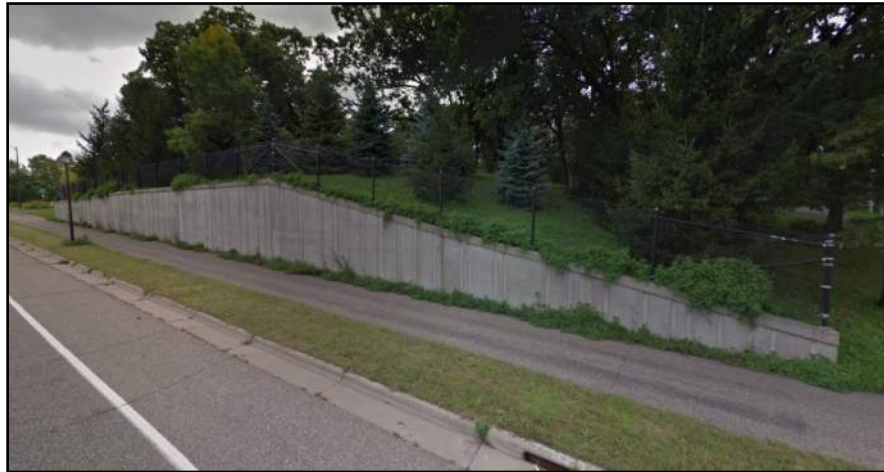
Image 3: Overall View of Lakeville Retaining Wall.
