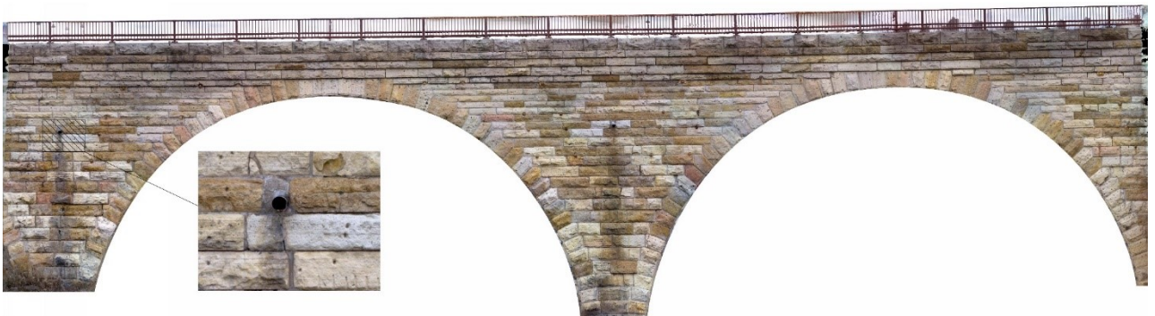
Figure 4.7 Pix4D Bridge Facade Orthoplane
