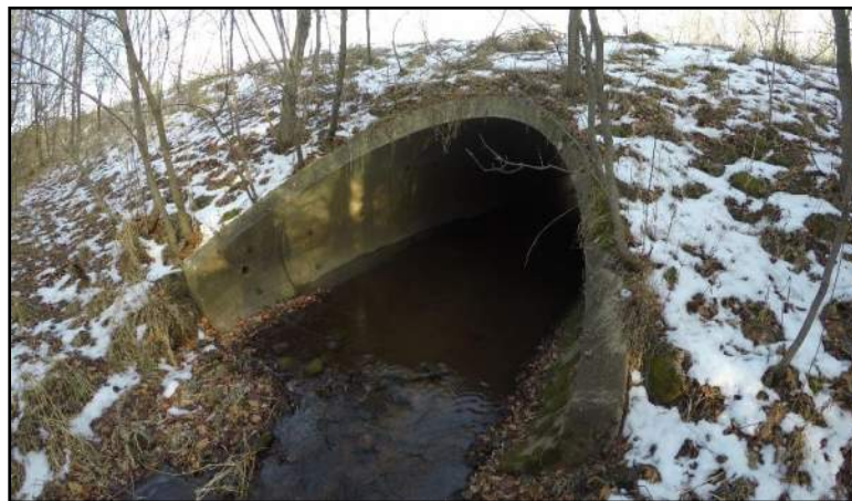
Image 3: View of Culverts East Entrance.
