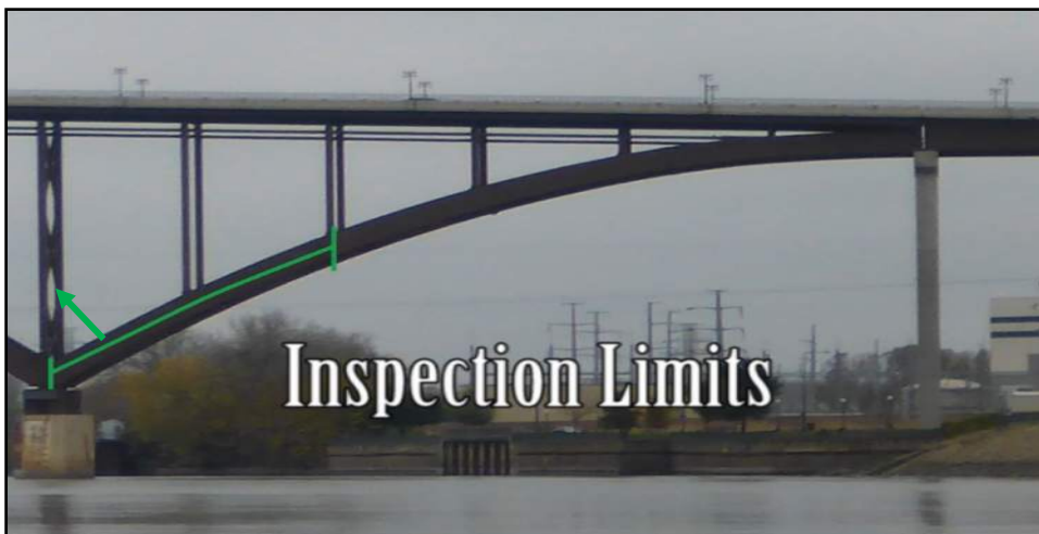
Image 3: Overall View of Bridge Underside & Inspection Limits for Steel Arch.
