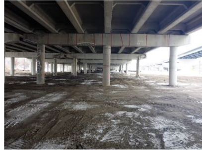
P1300082 – Pier 37WB, looking west
