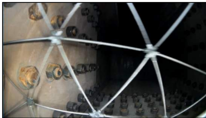
Image 6: View of Elios Inspecting a Splice in the Arch.
