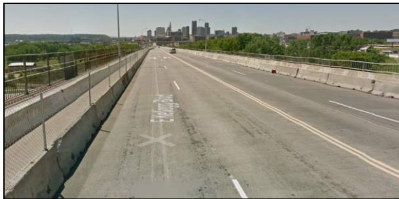
Image 2: Overall View of Bridge Topside.
