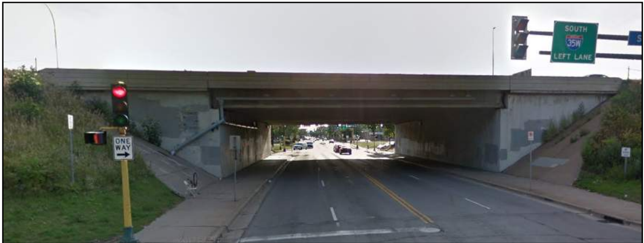
Image 2: Overall View of Bridge.
