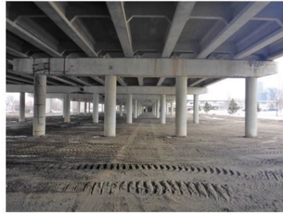
P1300096 – Pier 37EB, looking east
