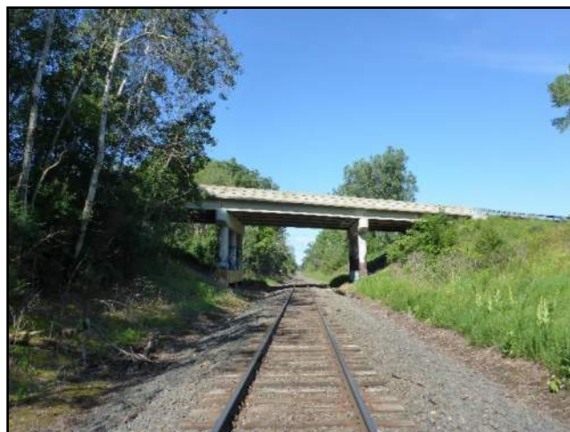
Image 3: Overall Elevation View of Bridge.
