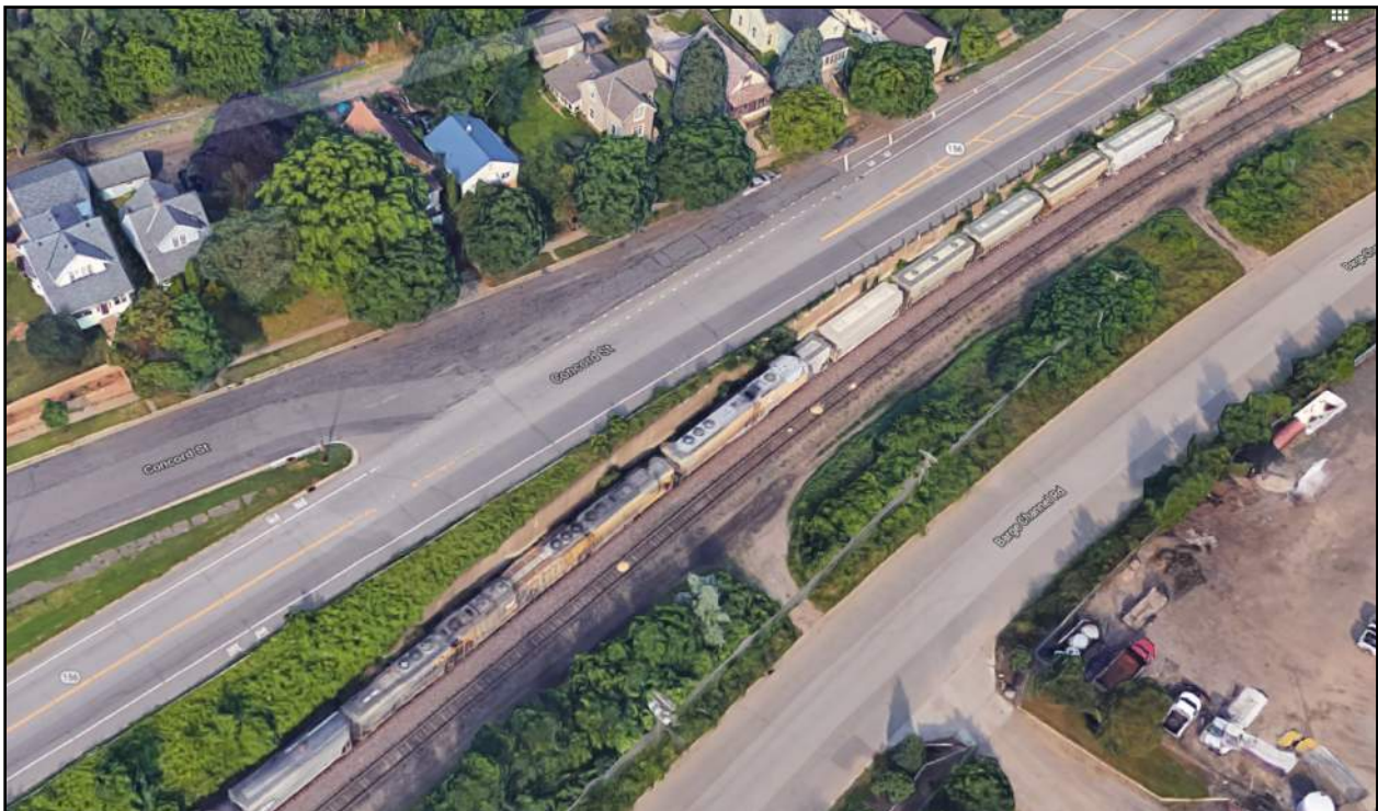
Image 4: Overall View of South St. Paul Retaining Wall.
