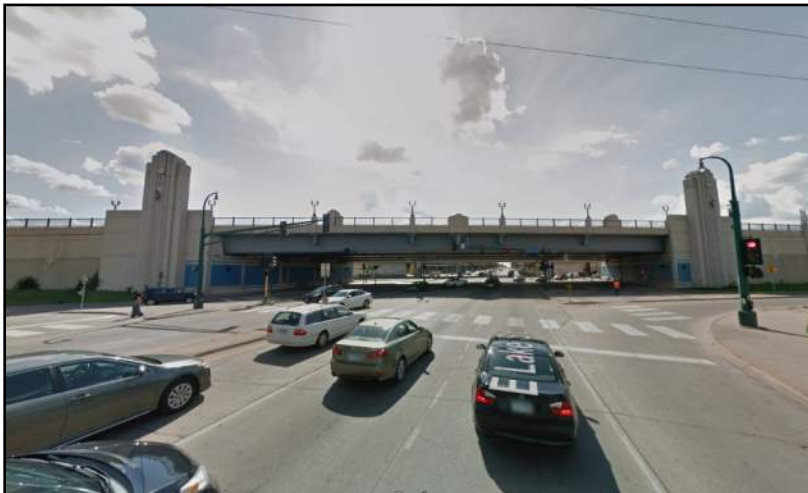
Image 2: Overall View of Bridge.
