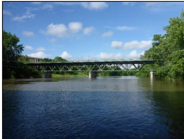
Image 2: Overall View of the Bridge fascia.
