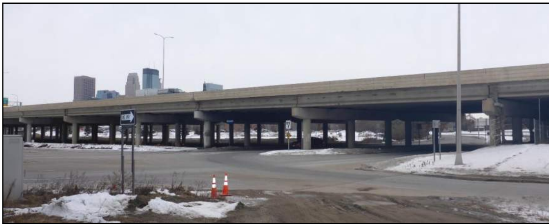
Image 2: Overall View of Bridge North Elevation.
