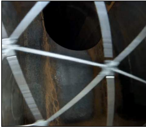
Image 9: View of Elios Inspecting an Arch Rib Section.
