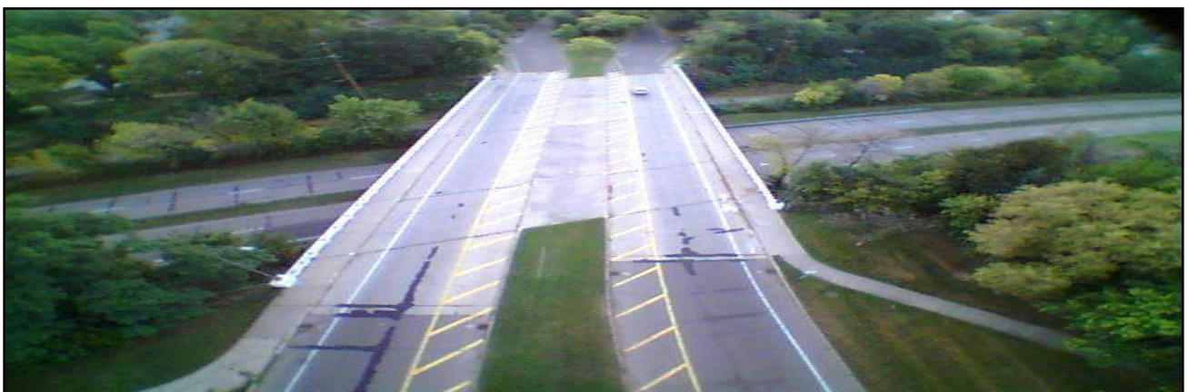
Image 3: Overall View of Bridge Deck.
