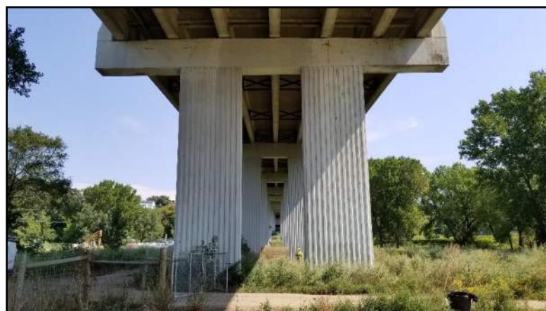
Image 3: Overall View of Bridge Underside.
