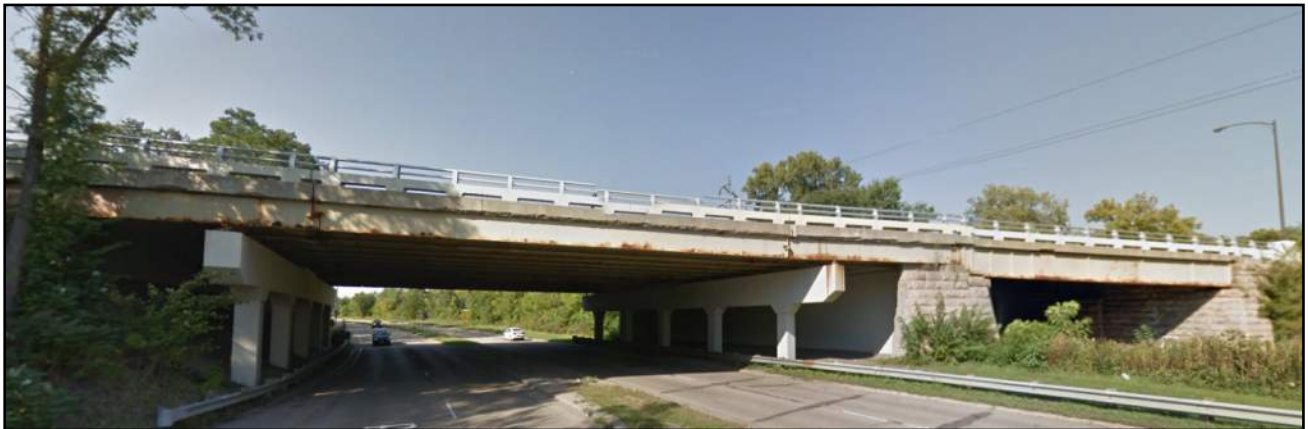
Image 2: Overall View of Bridge.
