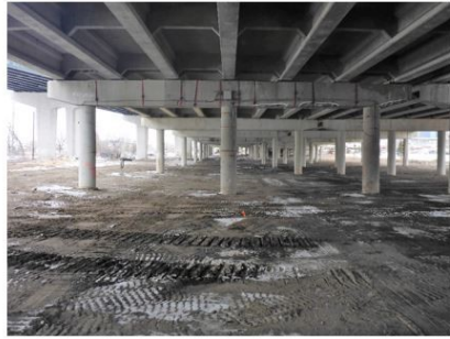
P1300083 – Pier 37WB, looking east
