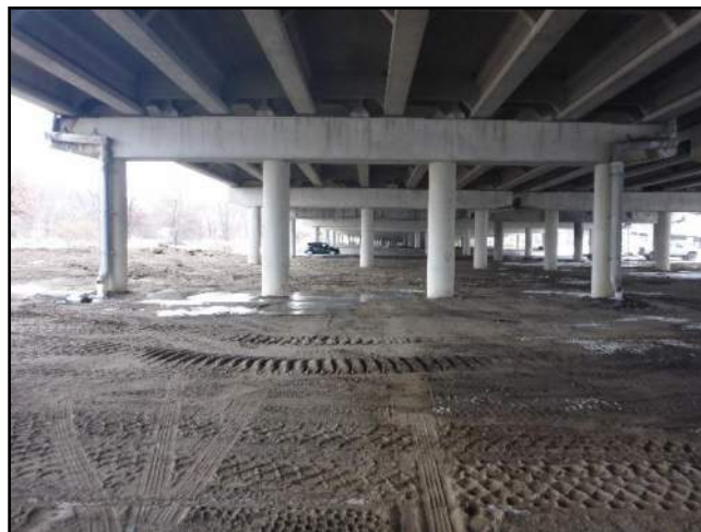
Image 3: Overall Elevation View of Typical Concrete Pile Bent.
