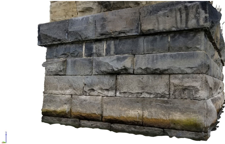
Figure 4.9 3D Model of Bridge Pier Created from Terrestrial Photos
