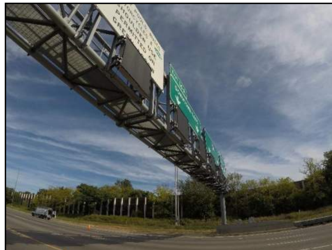
Image 3: Overall View of Gantry Underside.
