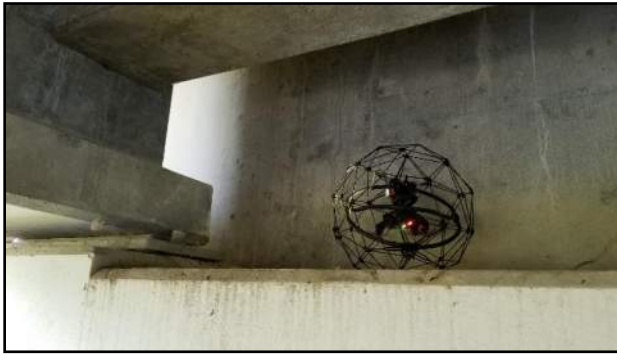
Image 8: View of Elios Inspecting a Hard to Reach Bearing.
