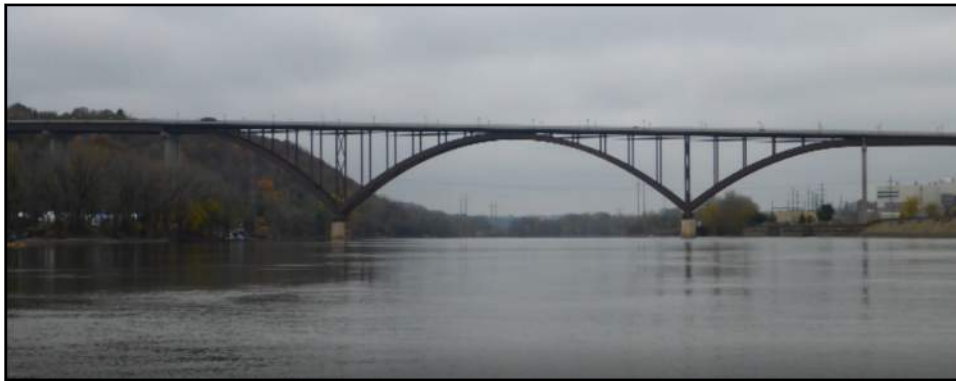
Image 2: Overall View of Bridge.
