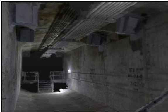
Image 13: 3D model of the Inside of the Box Girder. (Click Image to access 3D Model)
