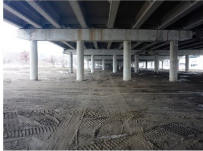
P1300097 – Pier 37EB, looking west
