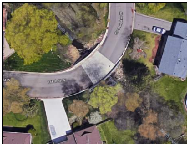
Image 2: Overall View of Bridge.
