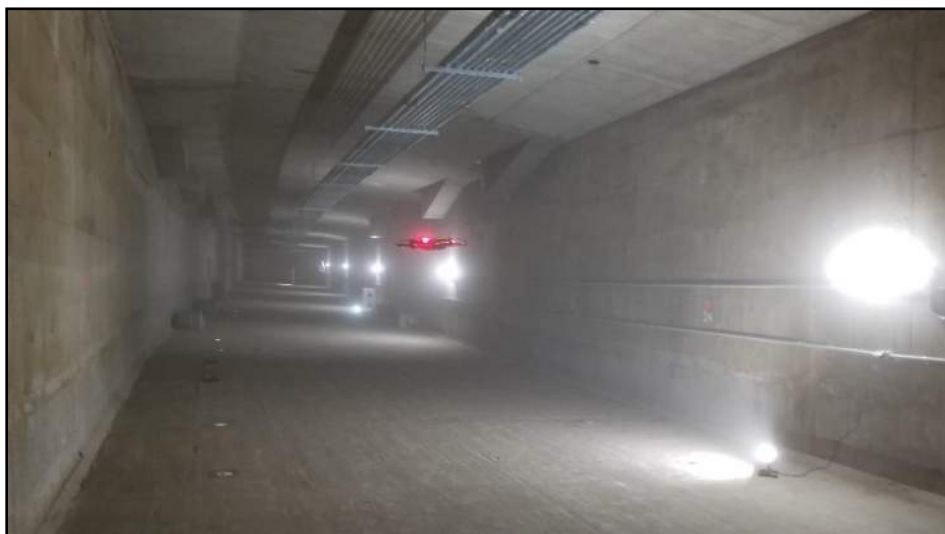
Image 8: View of Albris Gathering Detailed Photographs of Girder.
