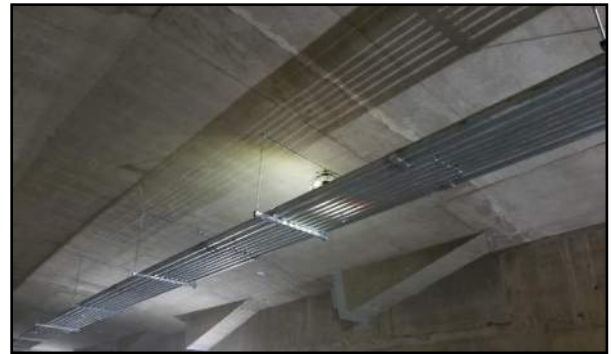
Image 10: View of Elios Inspecting a Hard to Reach Face of Girder.
