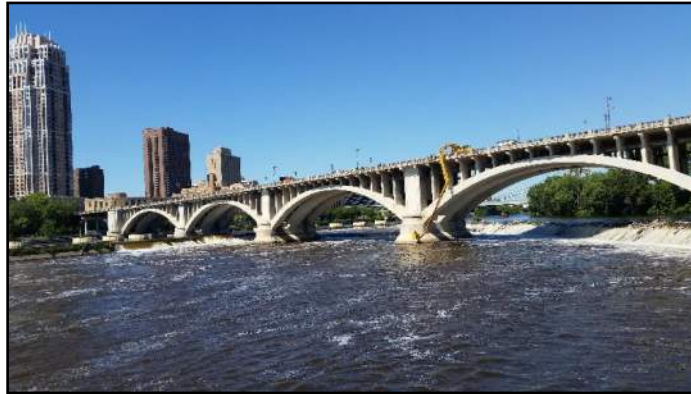
Image 2: Overall View of Bridge Topside.
