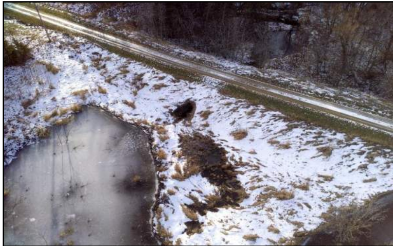
Image 2: Overall View of Culverts Topside.
