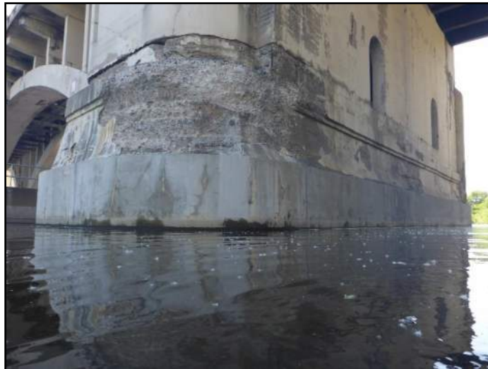
Image 3: Overall View of Bridge Pier.
