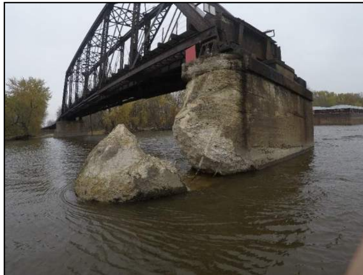
Image 3: Overall View of Bridge Underside.
