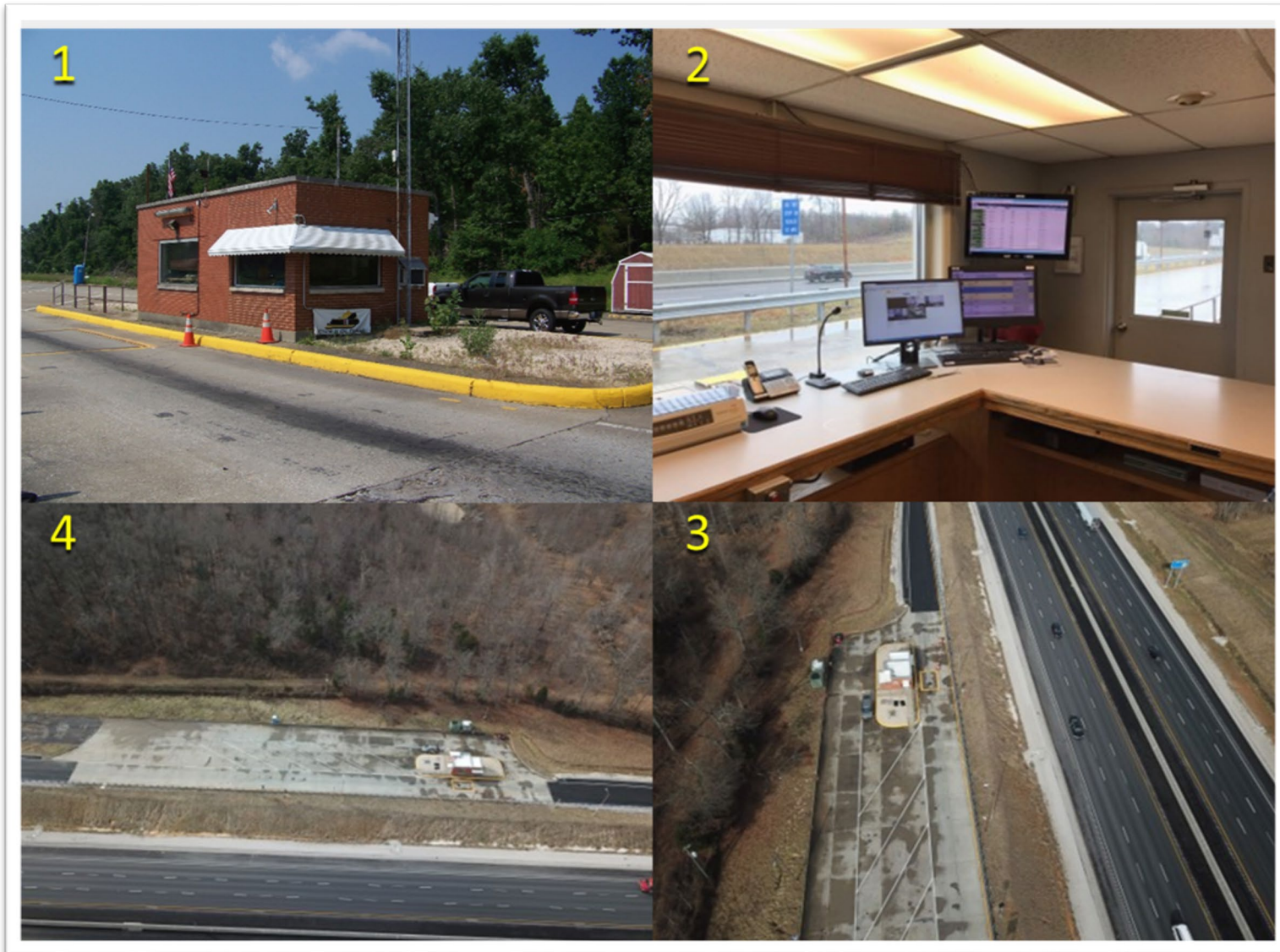
Figure E.6 Hardin Weigh Station Photos
