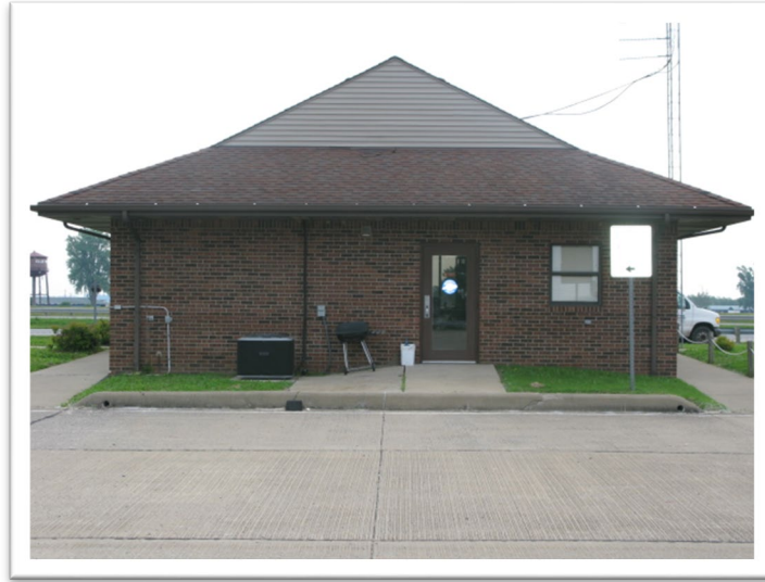
Figure 4.7 Henderson Scale House
