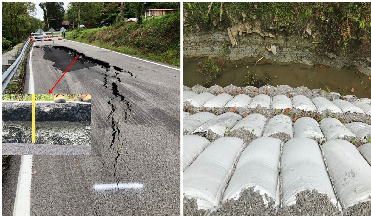
Figure 3.8 Roadway Failure (Left) Earthbag Barrier Wall (Right)
