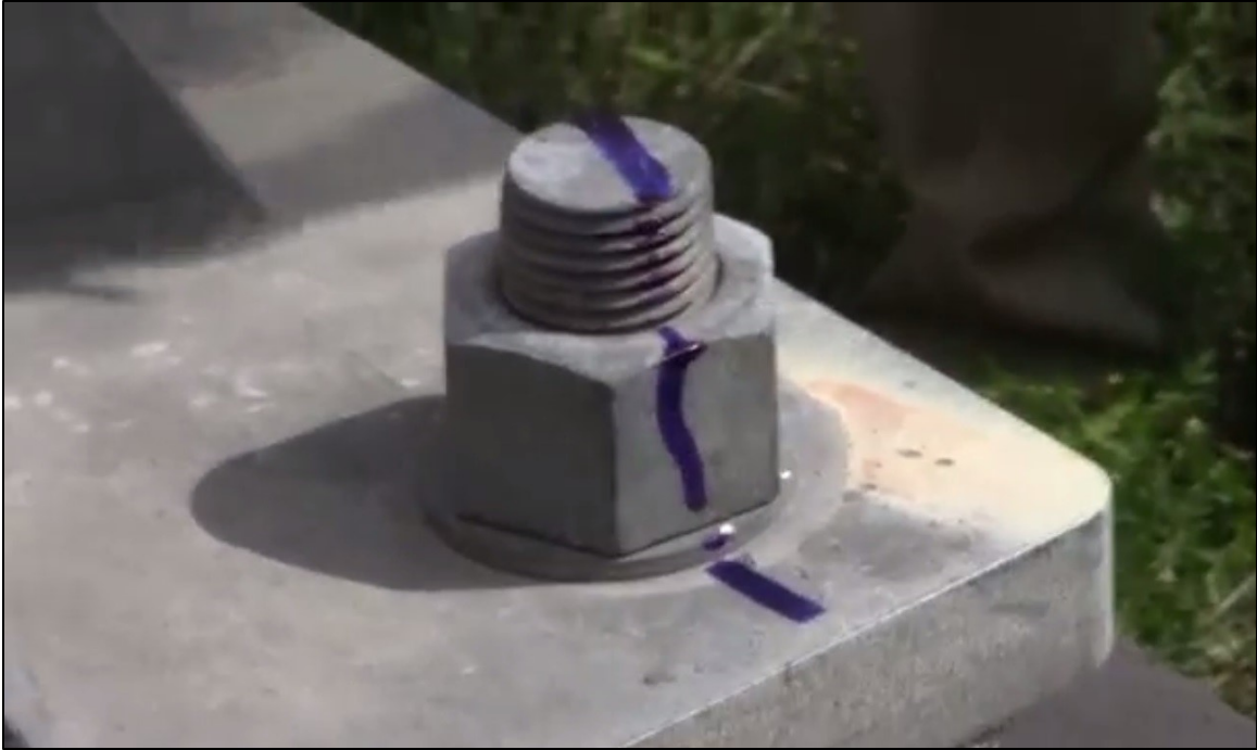
Figure 3-16 - Reference Marks Used During Maintenance
