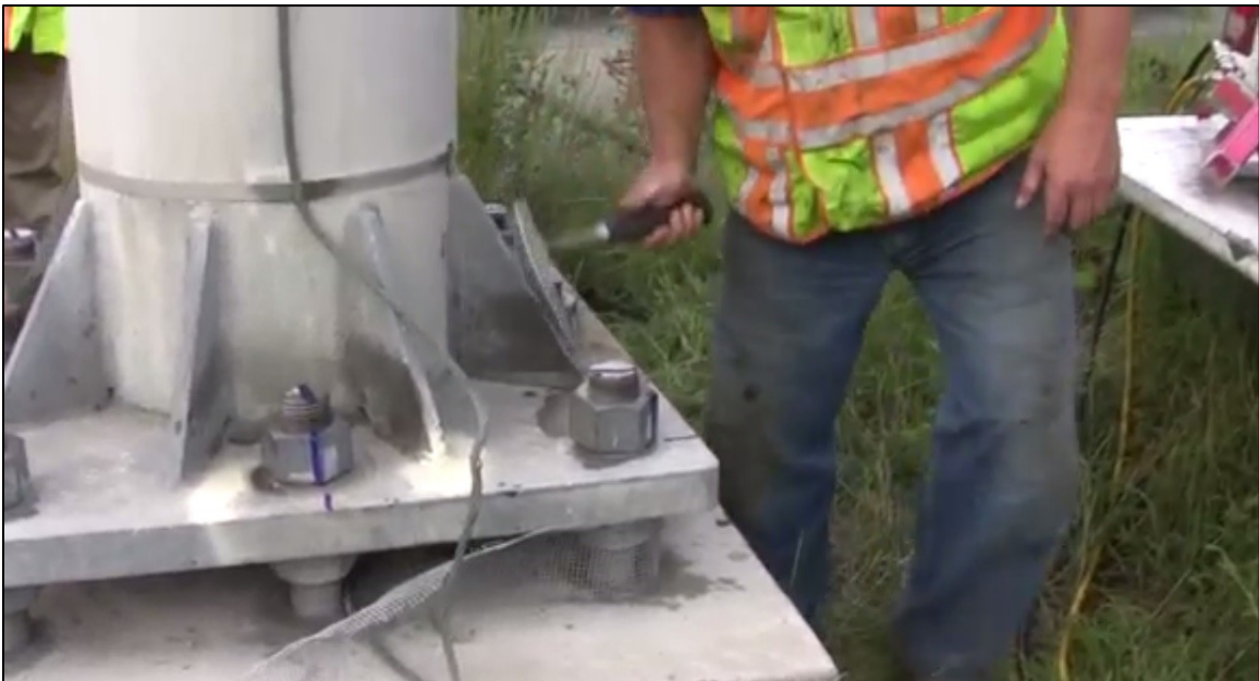
Figure 3-15 - Washers Struck to Inspect Nut Tightness
