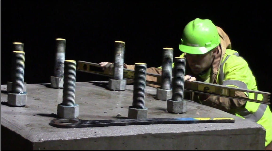
Figure 3-20 - Leveling During Iowa Site Visit
