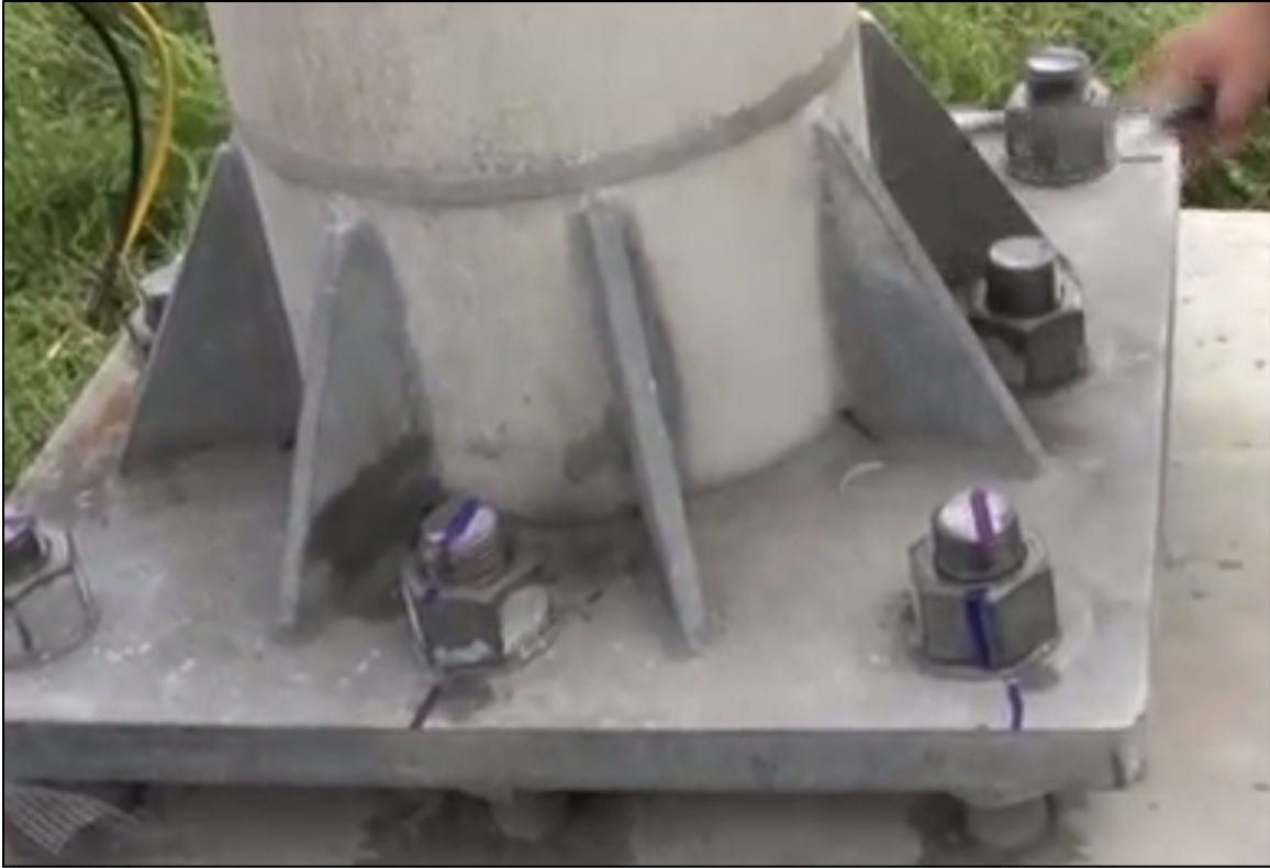
Figure 3-18 - After Maintenance Retightening
