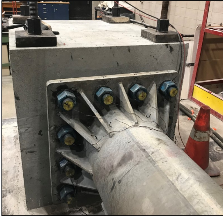
Figure 5-36 - Concrete Block Following Post-tensioning
