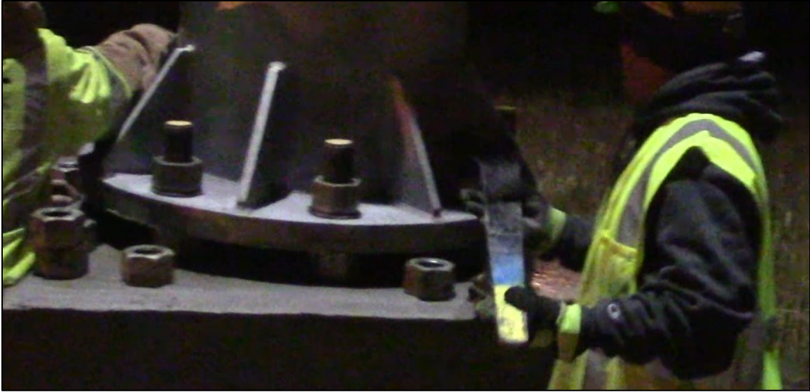
Figure 3-24 – Snug-tightening of Bolts
