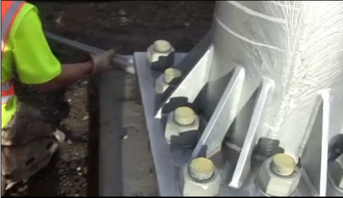
Figure 3-10 - Leveling Nut Tightening in Minnesota
