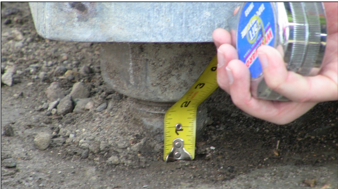
Figure 3-13 - Distance from Foundation to Bottom Leveling Nut
