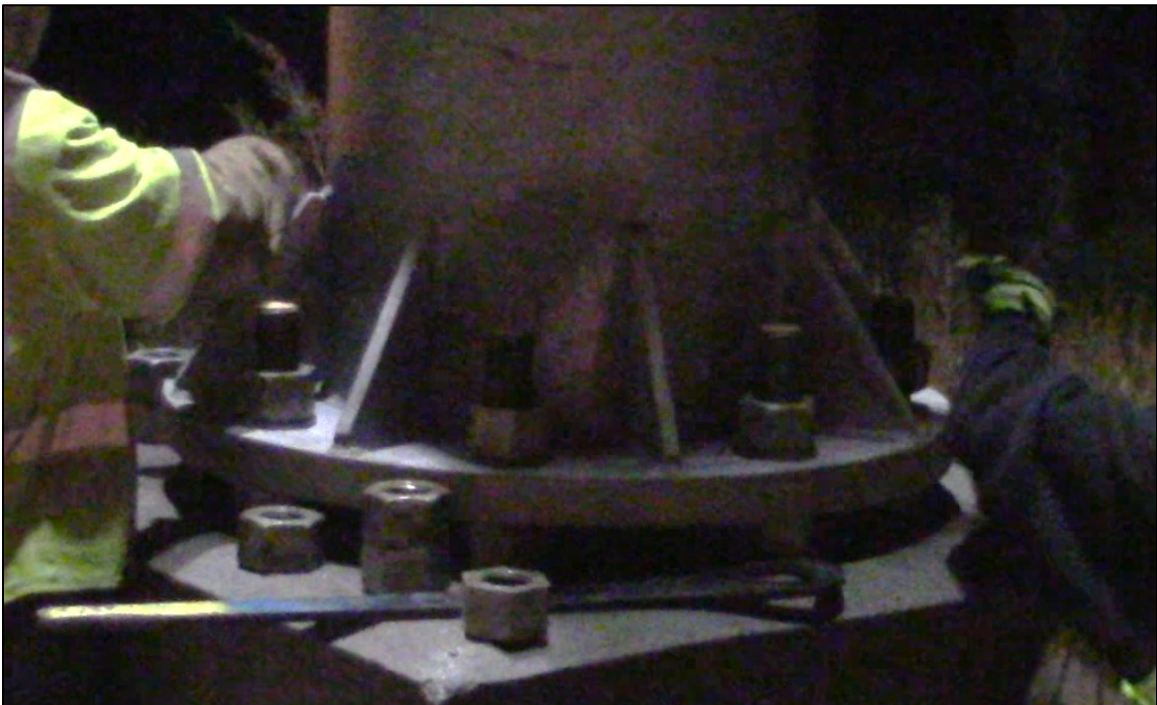
Figure 3-23 - Hand Tightening of Bolts
