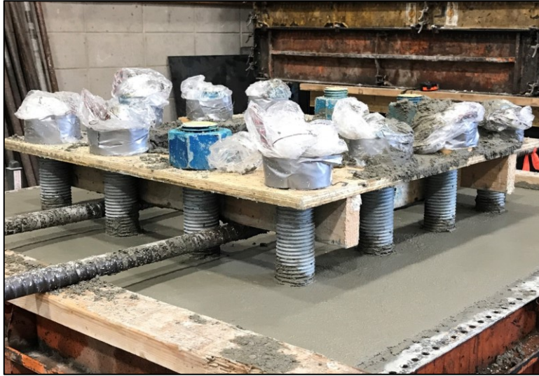
Figure 5-30 - Anchor Bolts during Concrete Curing
