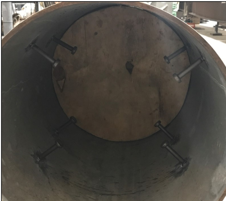
Figure 5-31 - Shear Studs and Wood Form Inside Sign Post
