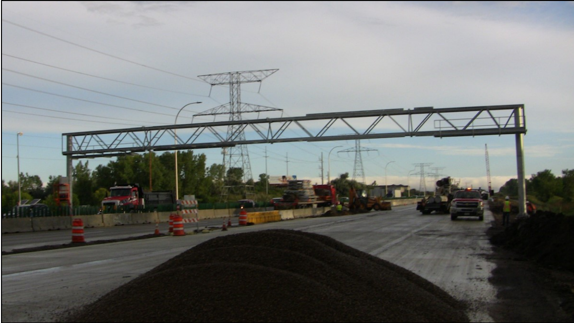
Figure 3-6 - Overhead Sign Truss on Interstate 494 Near Maple Grove
