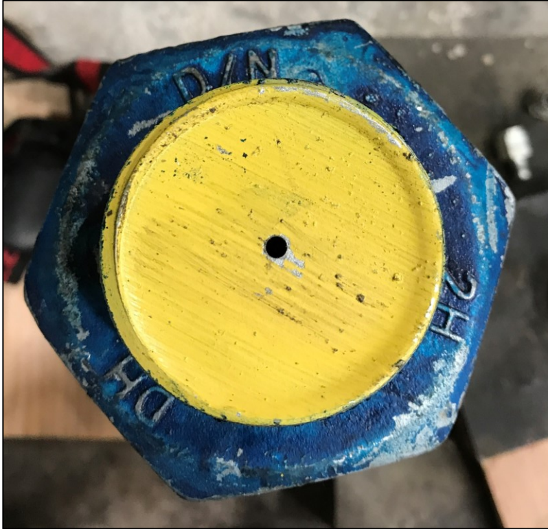
Figure 5-5 - Predrilled Hole in 2-1/4" Anchors
