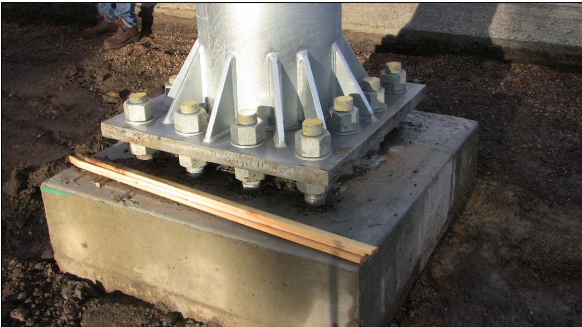
Figure 3-7 - Overhead Truss Baseplate and Anchor Bolts
