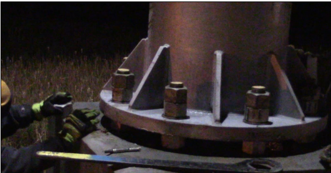
Figure 3-27 - Final Assembly with Jam Nuts
