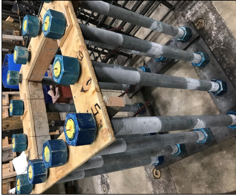
Figure 5-28 - Anchor Bolt Cage
