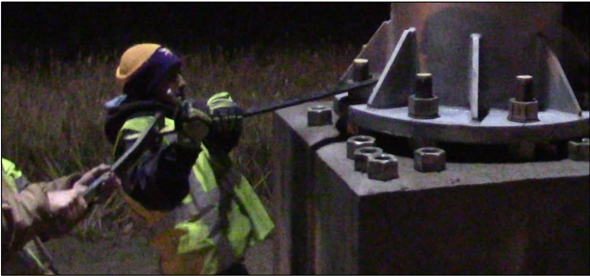
Figure 3-25 - Final Tightening After Making Reference Marks
