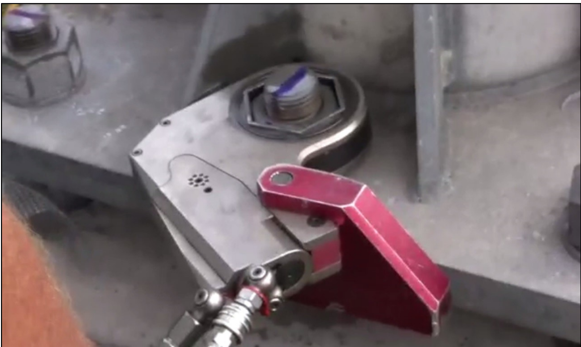
Figure 3-17 - Hydraulic Wrench Used for Maintenance Retightening
