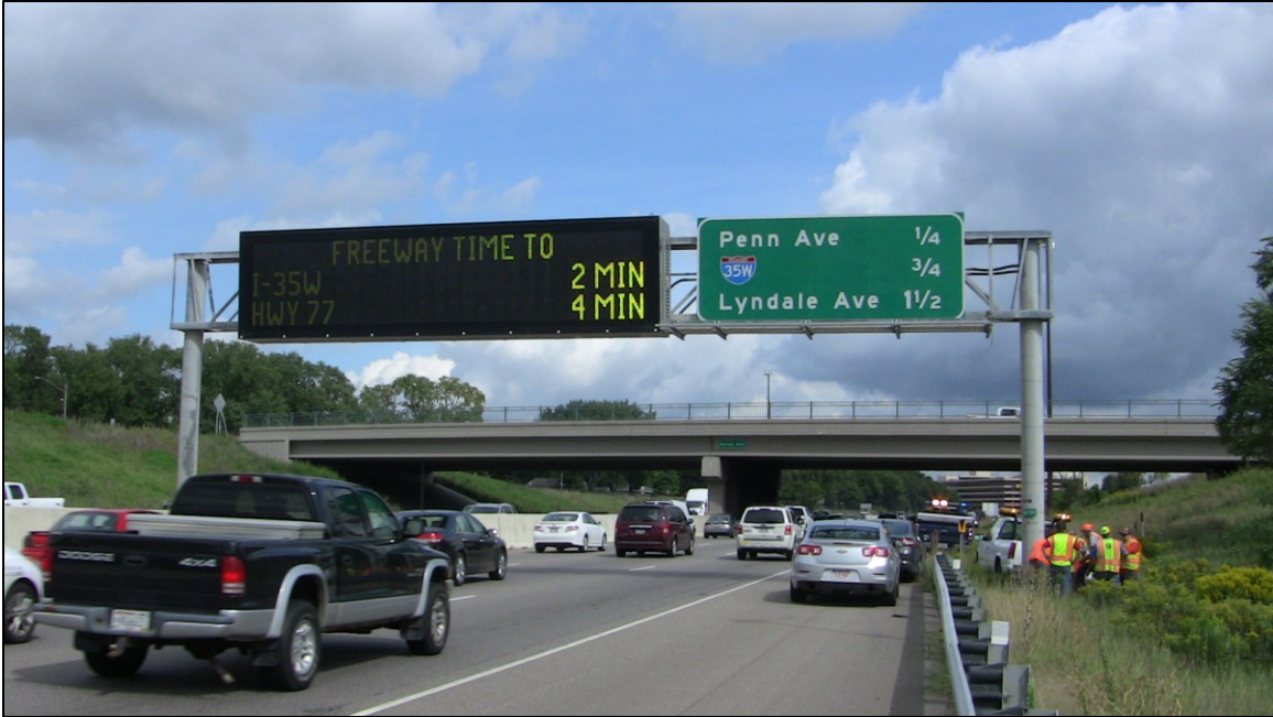
Figure 3-14 - VMS Support on I-494 Near I-35
