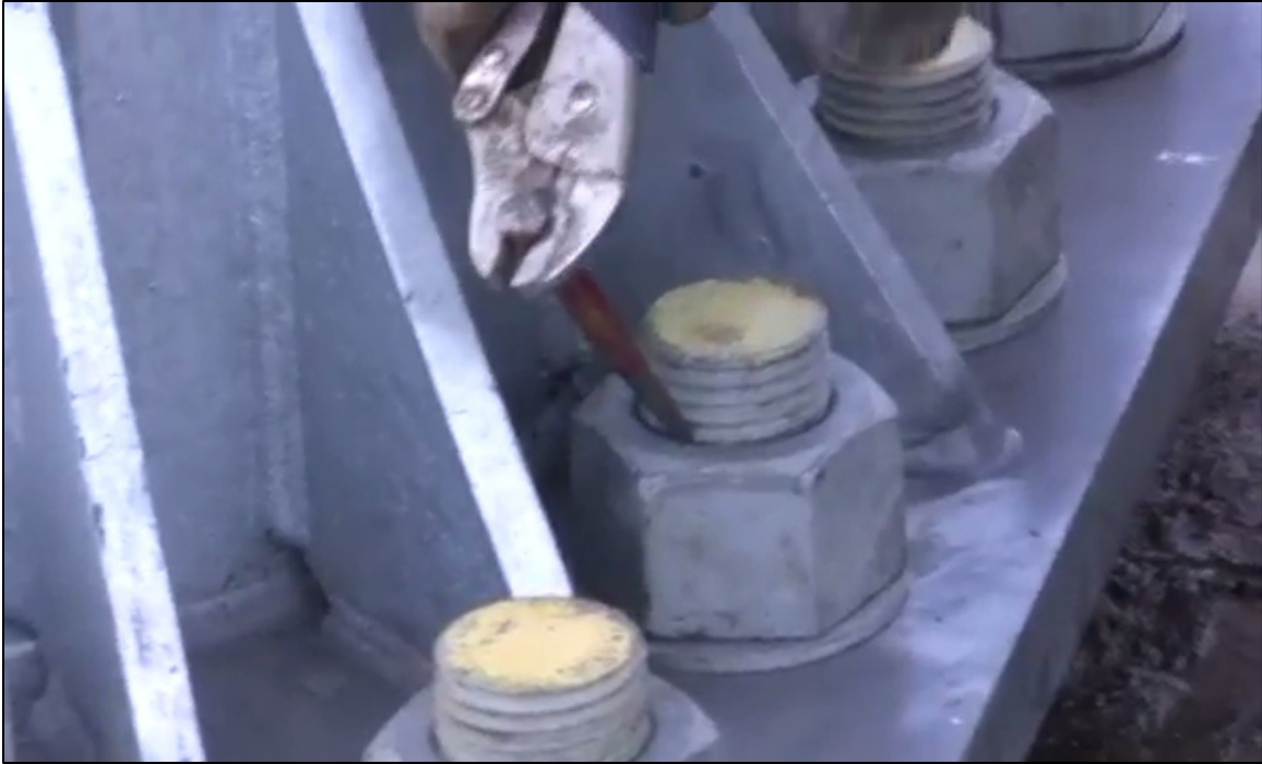
Figure 3-12 - Puncturing of Threads after Tightening
