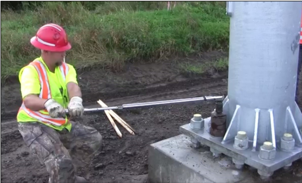
Figure 3-11 - Top Nut Tightening with Calibrated Wrench in Minnesota
