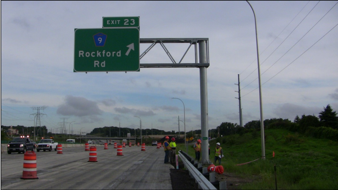
Figure 3-8 - Cantilevered Sign Support on Interstate 494 Near Maple Grove
