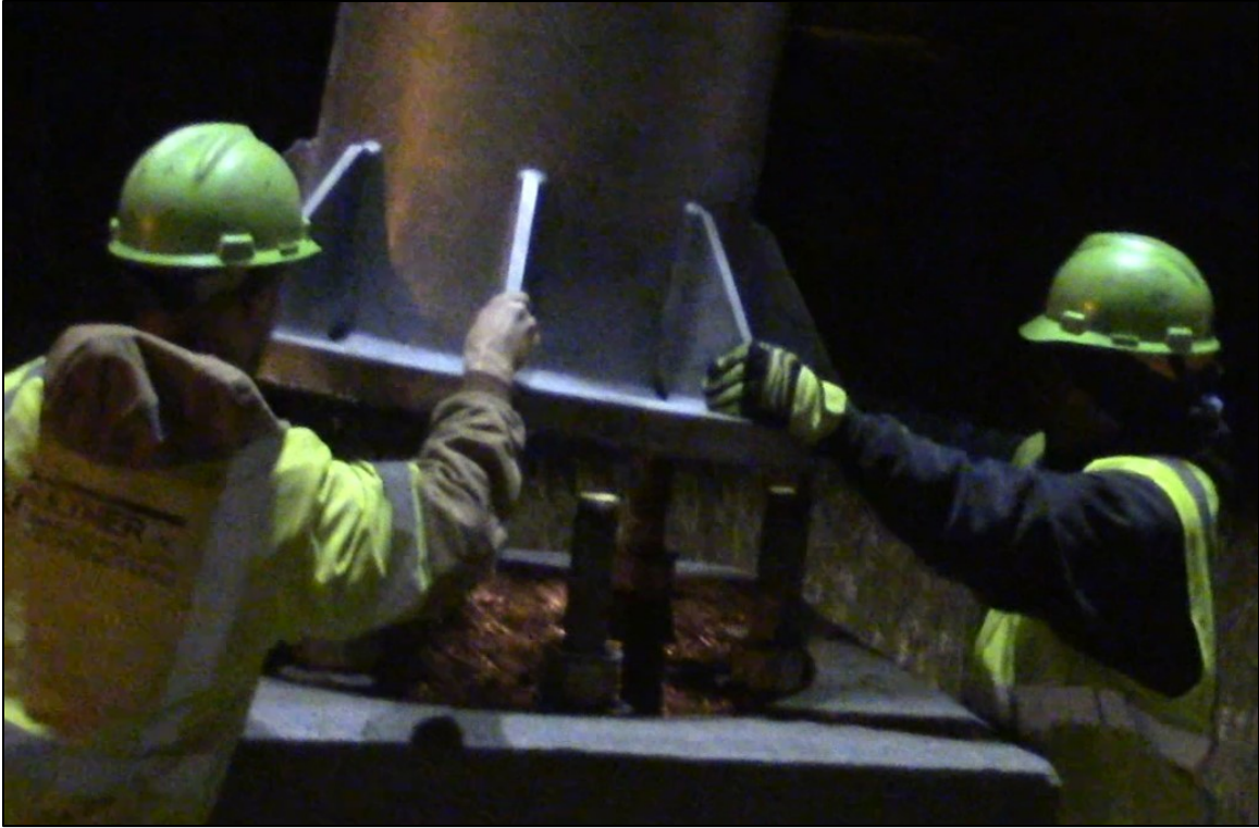
Figure 3-22 - Installation of Pole
