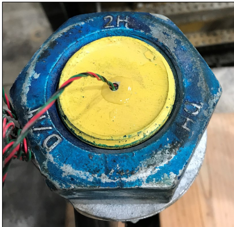
Figure 5-6 - Anchor Bolts after Strain Gage Installation
