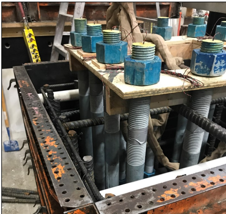
Figure 5-29 - Rebar, Anchors, and PVC Placed in Formwork
