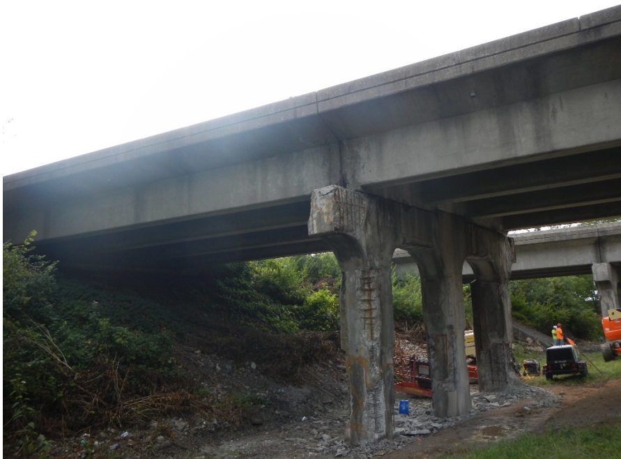
Figure 47 A pier with concrete removed for a jacketing repair
