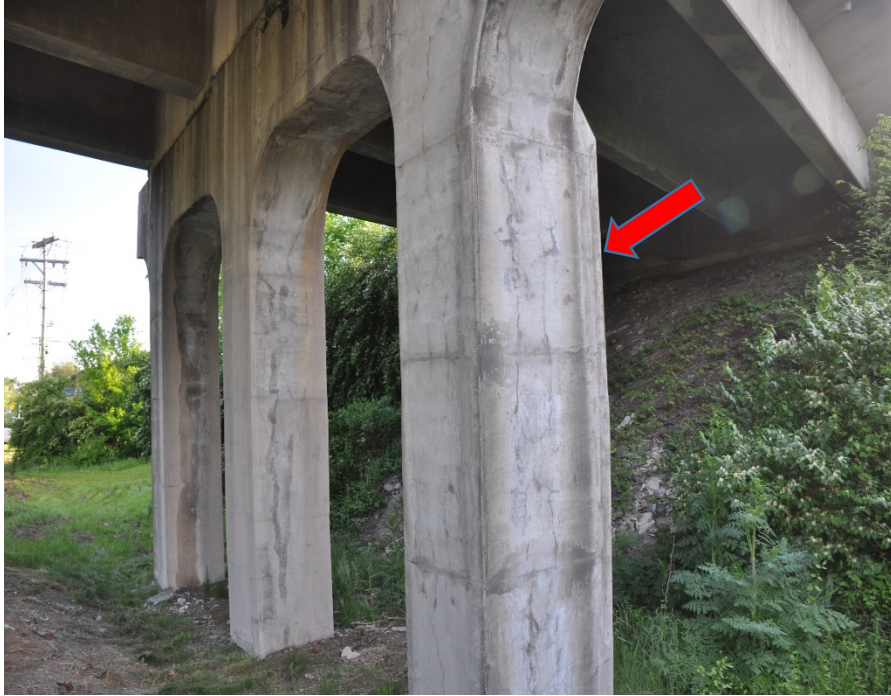
Figure 48 Repaired concrete pier with blister applied to strengthen a column (arrow)
