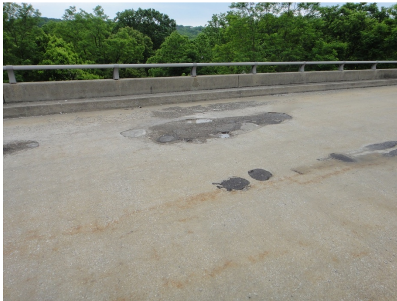
Figure 2 Spalled bridge deck concrete that has been patched
