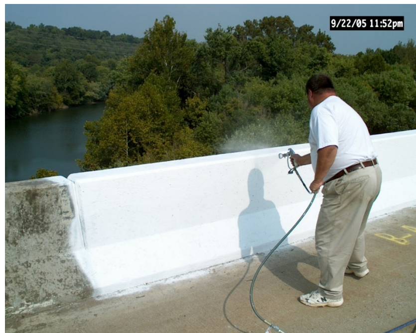
Figure 43 Spray painting of an acrylic coating on a barrier wall
