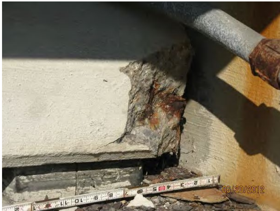
Figure 4 Spalling concrete on prestressed beam end under joint showing corroded reinforcing steel
