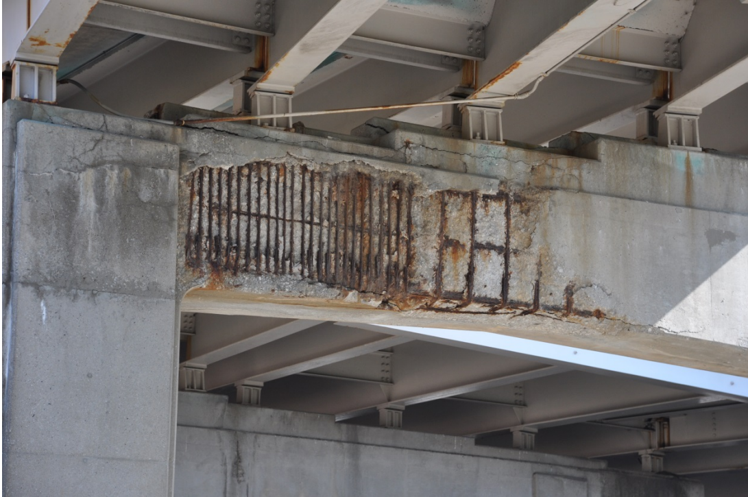
Figure 5 Spalling concrete on pier cap with corroded reinforcing steel
