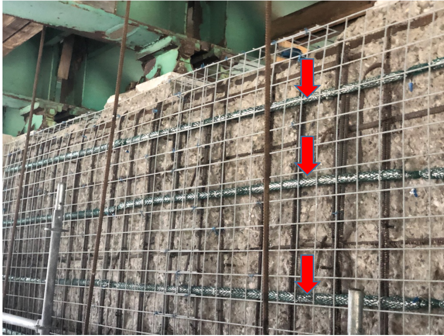
Figure 56 Distributed anodes (red arrows) employed on jacket repair (courtesy Vector Corrosion Technologies)
