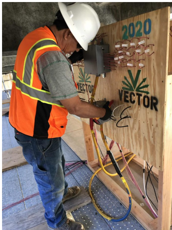
Figure 53 DC power control panel for electrochemical chloride extraction (courtesy Vector Corrosion Technologies)
