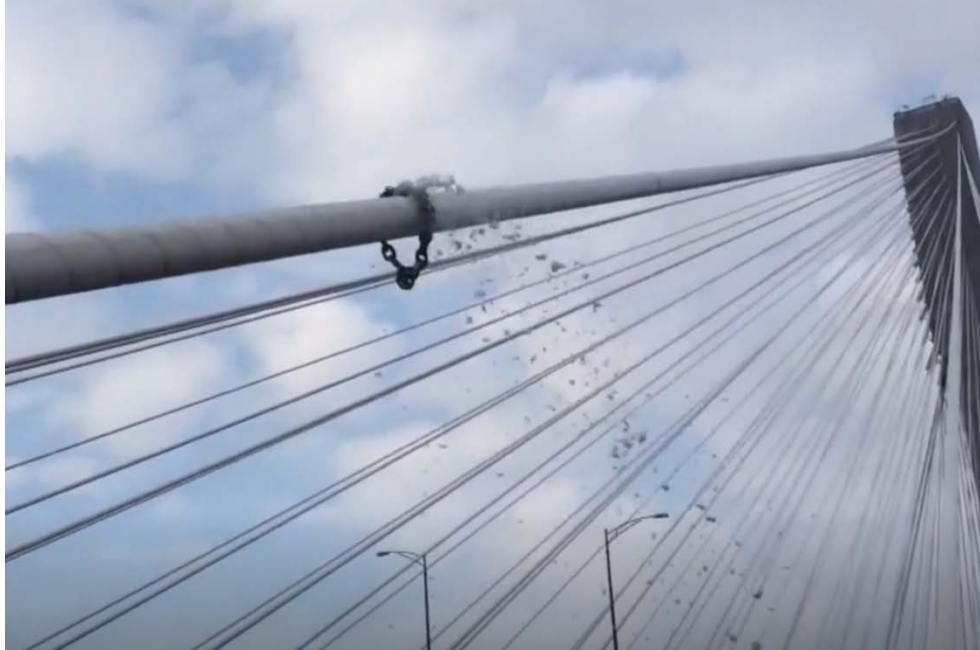
Figure 6 Deicing collar in operation
