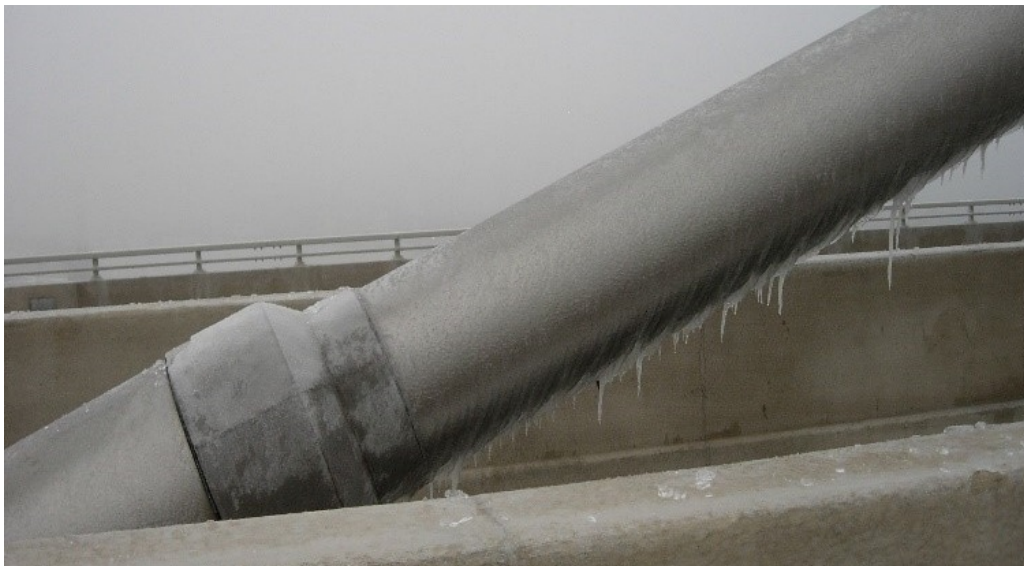
Figure 1 Ice forming on a cable stay [1]
