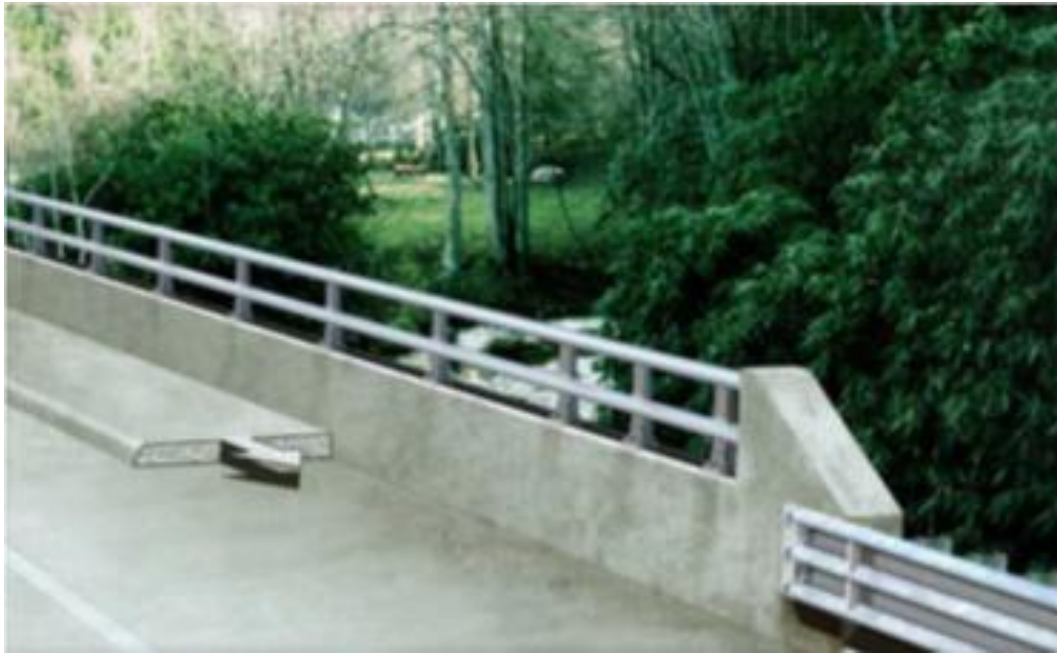
Figure 1. NCDOT Two-Bar Metal Bridge Rail Installation
