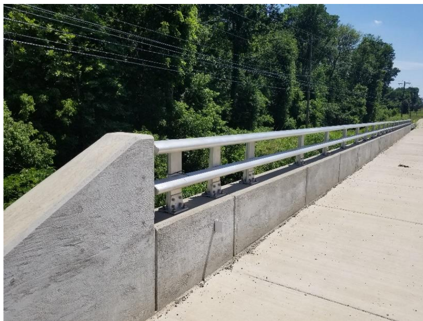
Figure 1.1: An NC two-bar metal rail.
