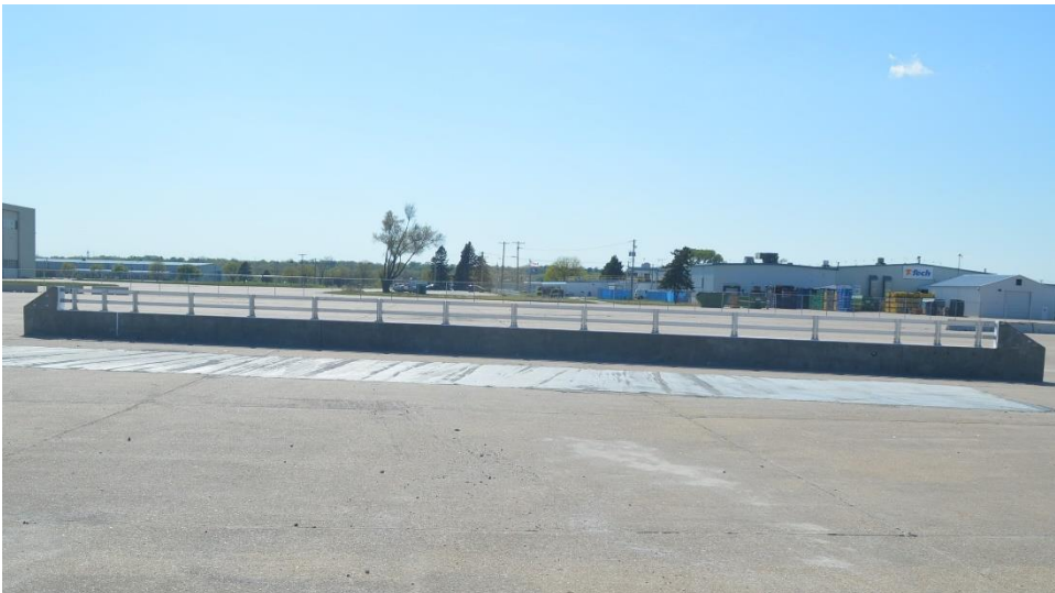
Figure 54. System Damage, Test No. NCBR-1
