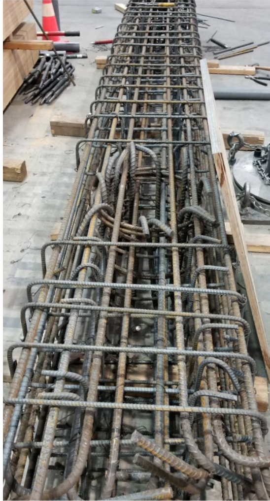
Figure 3.3 Reinforcement cage of cap beam
