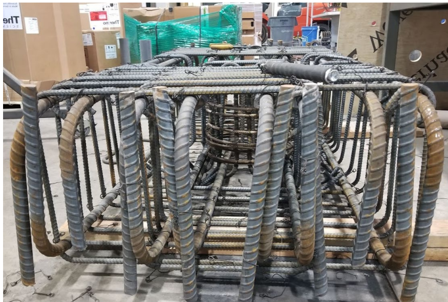
Figure 3.1 Reinforcement cage of footing
