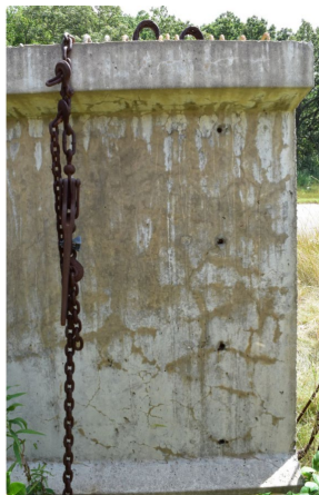
Map cracking on web
