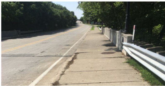
(a) General view of the bridge
