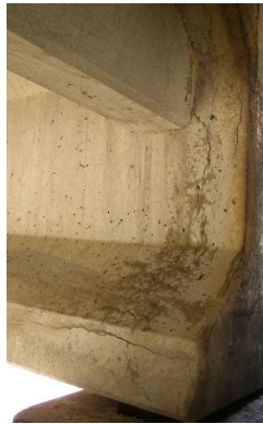
a) PC-I girder cracking
