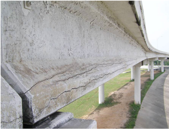
a) PC-I girder cracking
