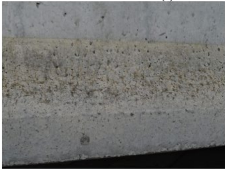
(b) Bottom flange map and longitudinal cracking
