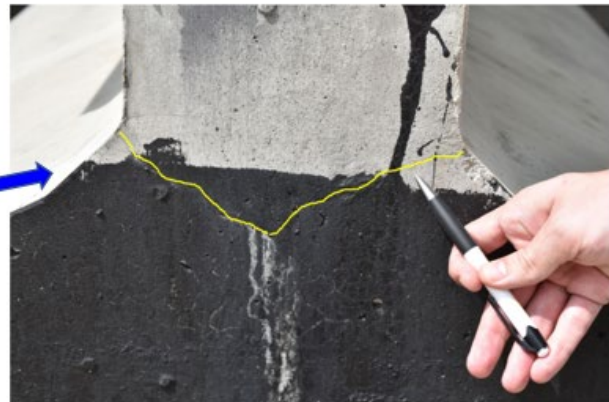
Close-up views of the crack with efflorescence at the bottom of the web
