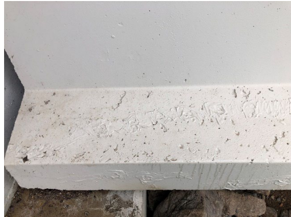
(b) Epoxy injected and repaired cracks
