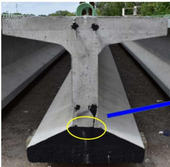
Cross-section of a bulb-tee girder
