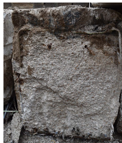
Figure D-3. Severely deteriorated beam ends (north end of the bridge)
