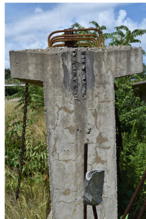
Map cracking on web
