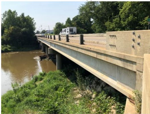
(b) Bottom flange of south fascia beam
