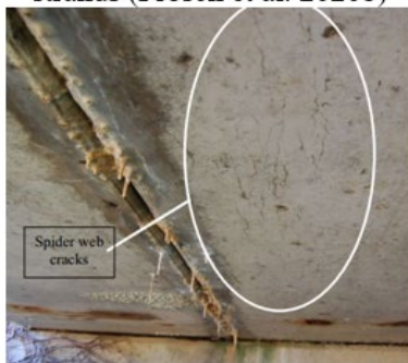
(e) Spider web cracks in box-beam bottom flange (Frosch et al. 2020b)
