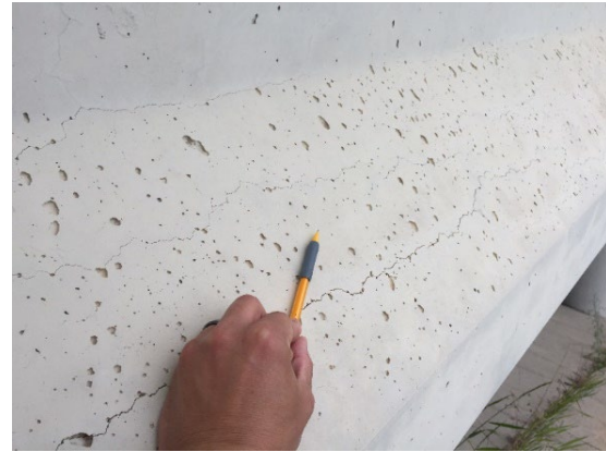
a) PC-I girder cracking
