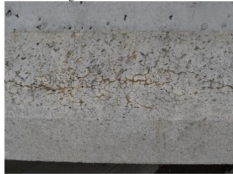
(b) Bottom flange map and longitudinal cracking
