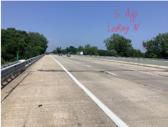
(a) General view of the bridge
