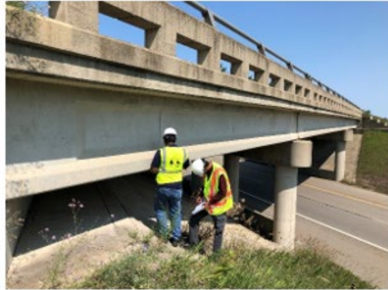
(b) East fascia beam (image taken from the south end)
