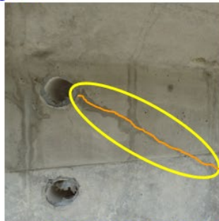
Close-up views of the diagonal crack
