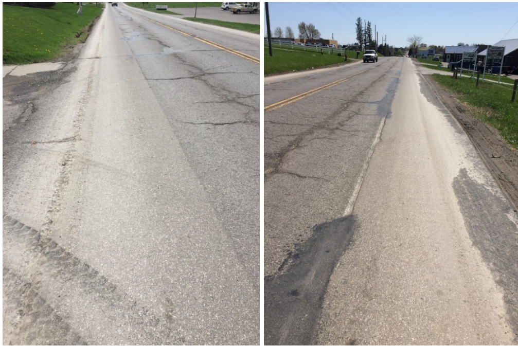
Figure A.10 Pictures of sections with AP2-76 mix after 20 months of construction
