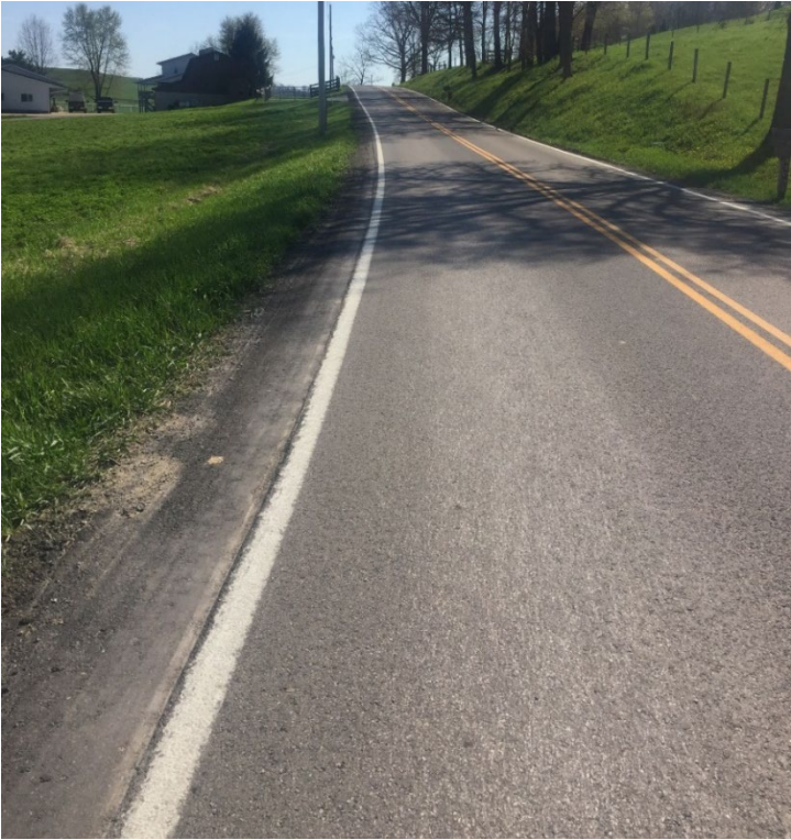
Figure A.12 Pictures of AP2-GTR test sections after 7 months of construction
