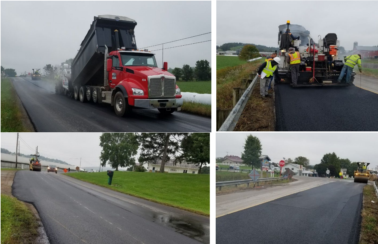
Figure A.4 Pictures taken during construction of test sections on CR 114
