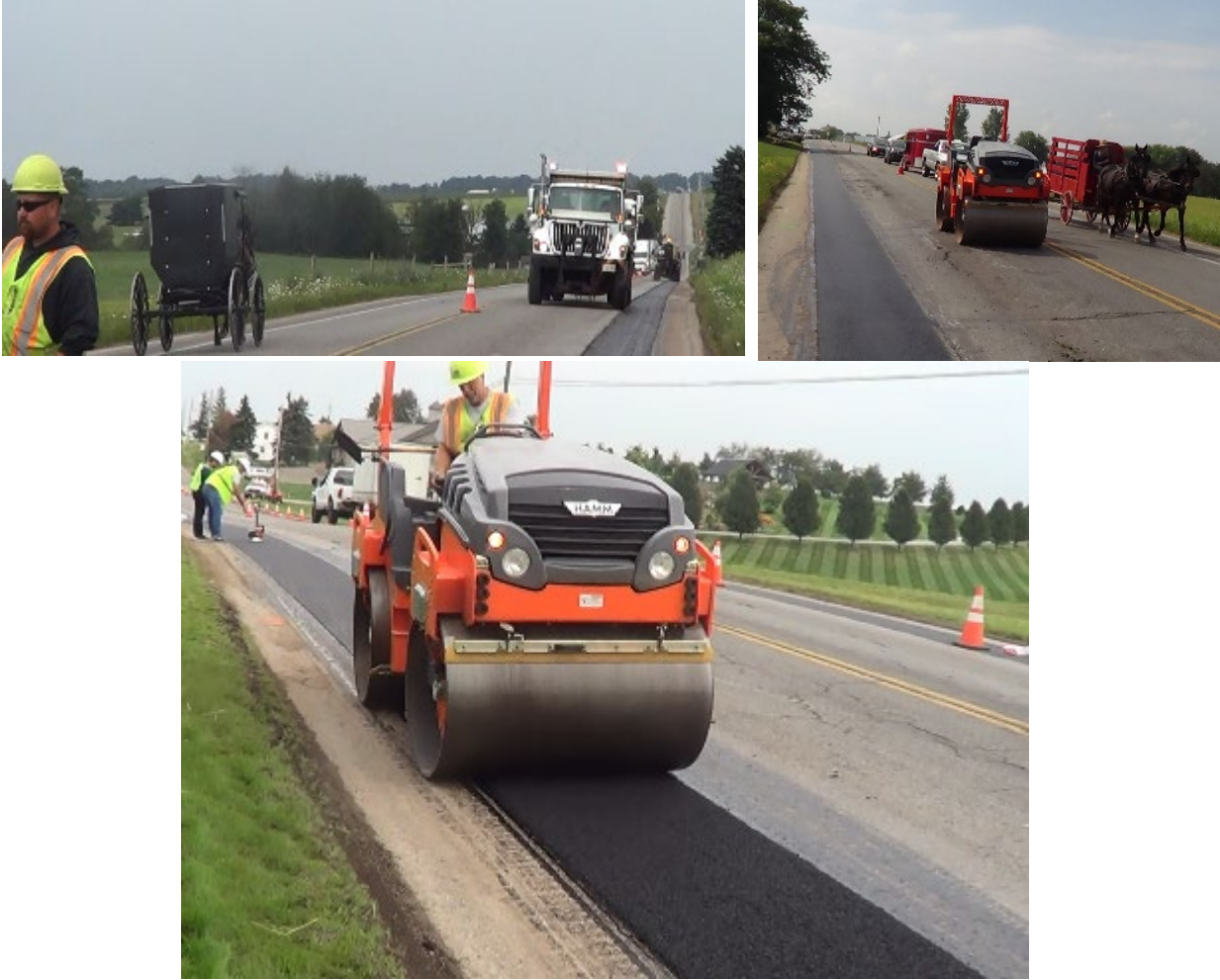
Figure A.3 Pictures taken during construction of test sections on SR 241
