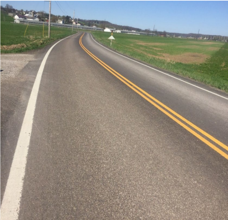
Figure A.13 Pictures of GTR-Mix test sections after 7 months of construction
