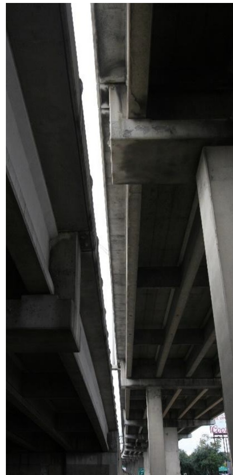
(c) Thruway bent adjacent to main bent at different elevation
