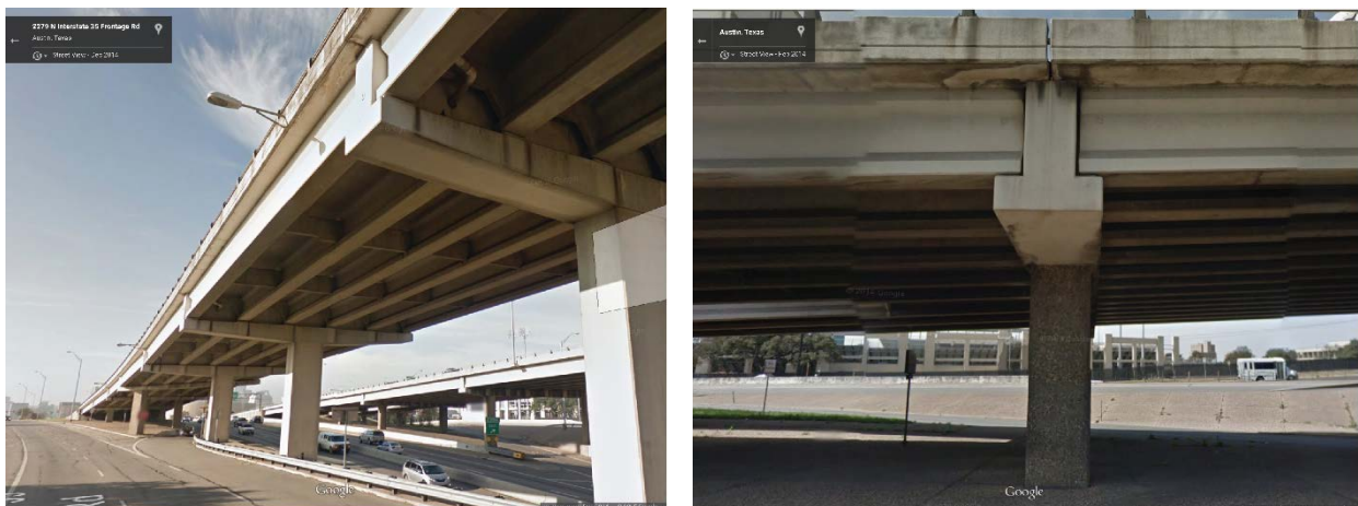
Figure 1.1. Inverted-T Bent Cap in Downtown Austin (Image from Google Maps).
