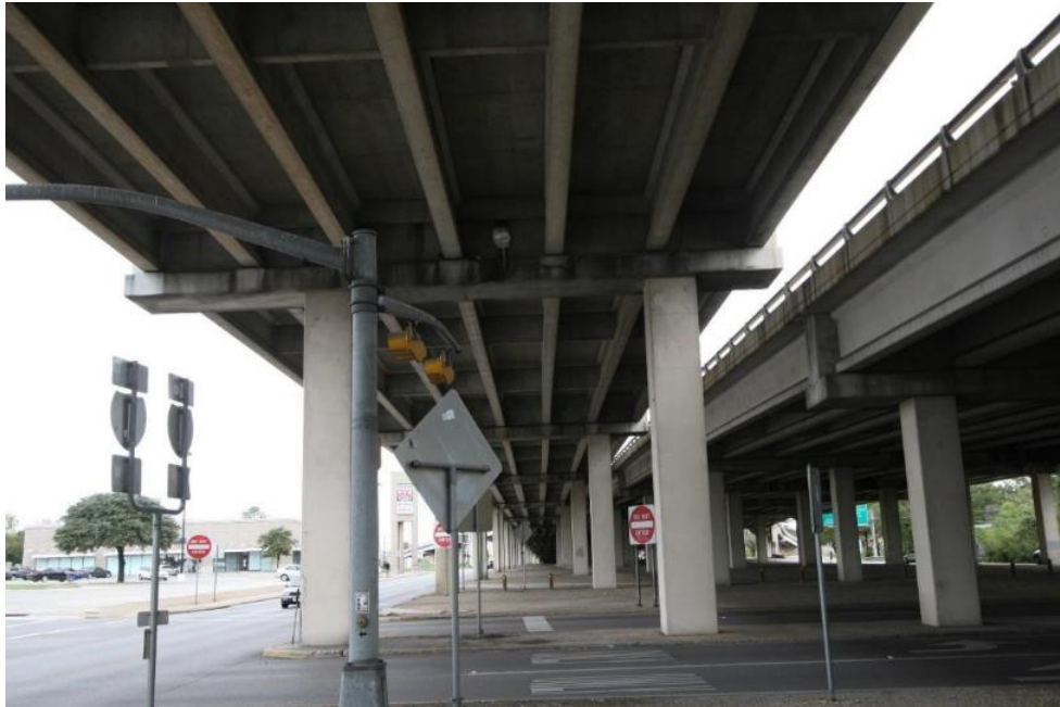
Figure 3.4. Unequal Overhang Lengths for Bent 16 of Northbound Thruway Lanes.
