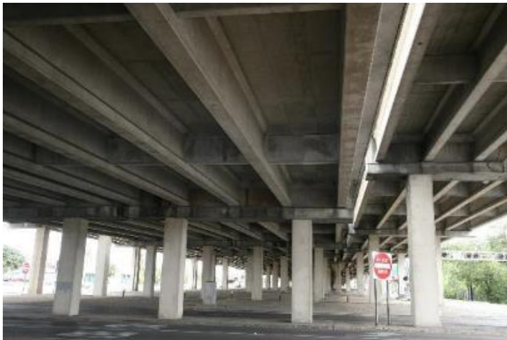
(b) Thruway bent adjacent to main bent at same elevation
