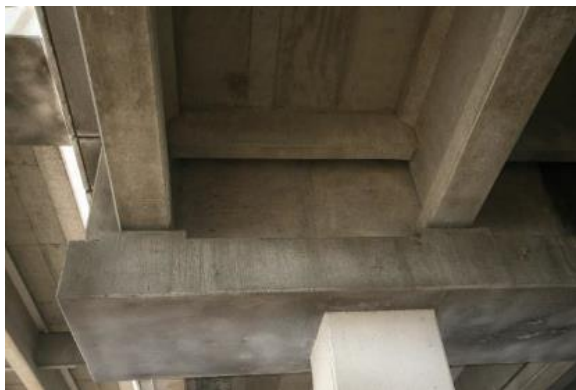
(a) Looking at face of bent cap
