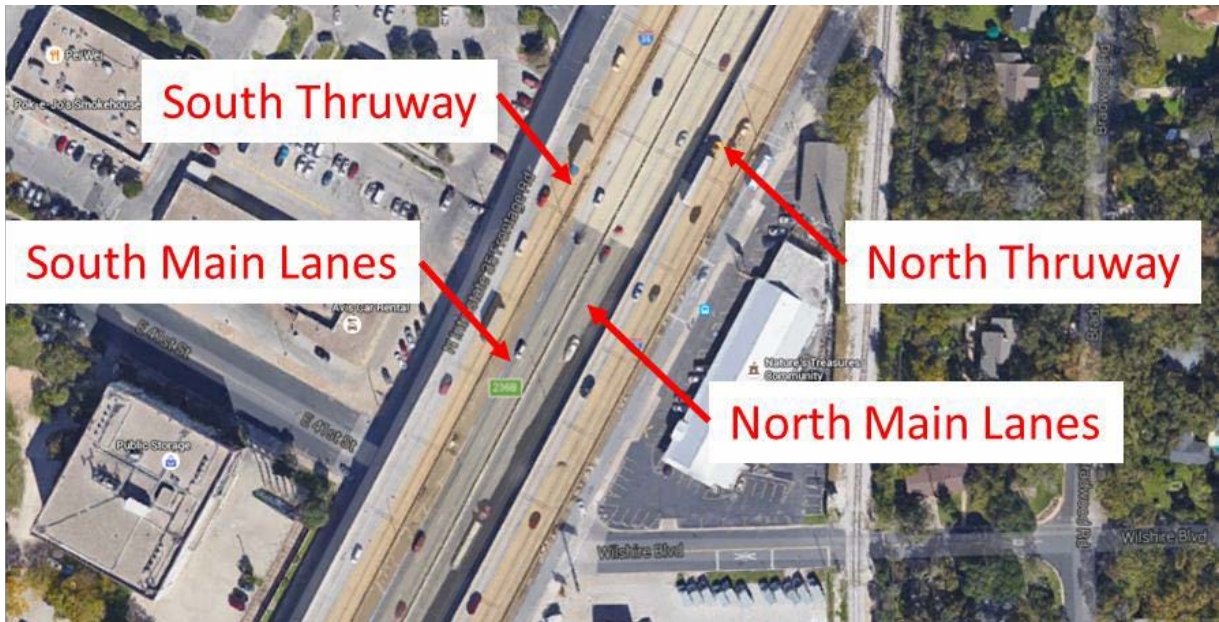
Figure 3.2. Plan View of Structures Observed during the First Field Visit (Image from Google Earth).
