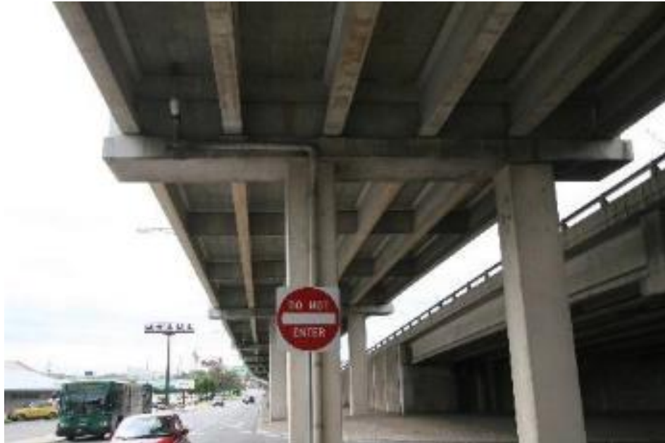
Figure 3.11. Drainage Pipes Attached to Ledge of Multi-Column Bent.
