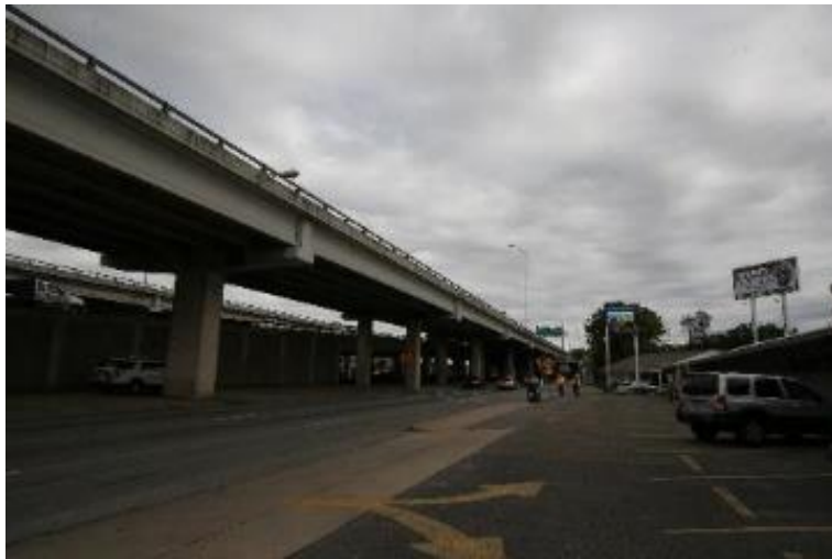
Figure 3.10. Frontage Road Adjacent to Thruway Lanes.
