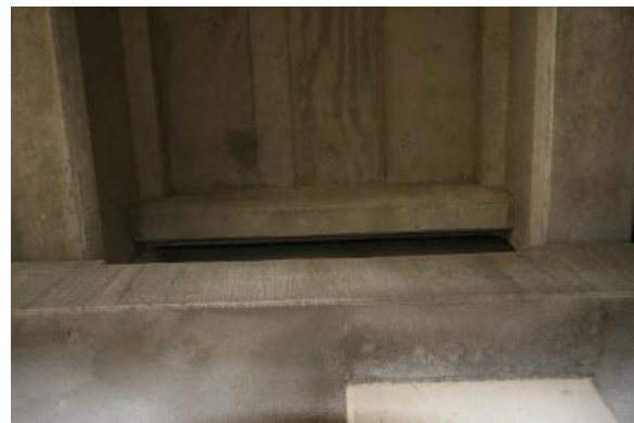
(b) Looking up toward bottom of deck
