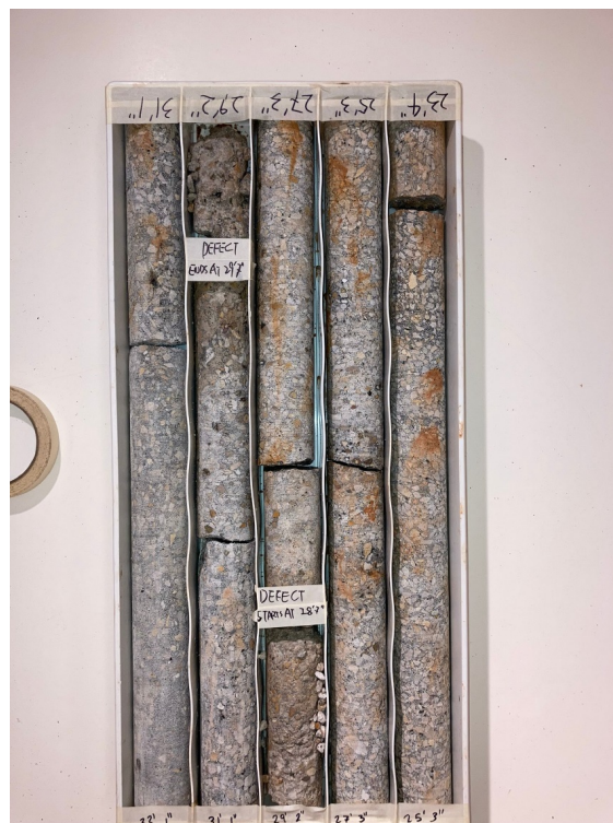
Figure 157. Photo. Photograph showing a core obtained from core #2 of test drilled shaft #3 showing the start and end of an observed defect between depths of 28 ft 7 in. and 29 ft 1 in.
