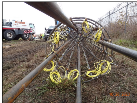
Figure 29. Photo. Photograph showing 3 ft diameter rebar cage with four CSL tubes and eight TIP wires installed.
