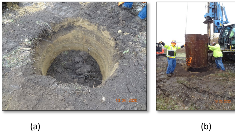
Figure 28. Photo. Photographs showing (a) start of excavation for test drilled shaft #3 and (b) installation of 4.5 ft diameter temporary casing.
