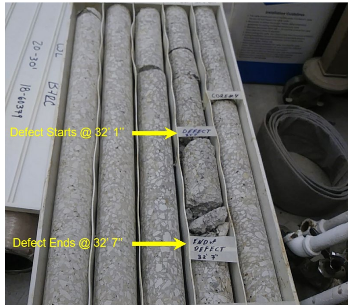
Figure 16. Photo. Cores obtained from coring test drilled shaft #1 showing the start and end of the observed defect between 32 ft 1 in. and 32 ft 7 in. depth.
