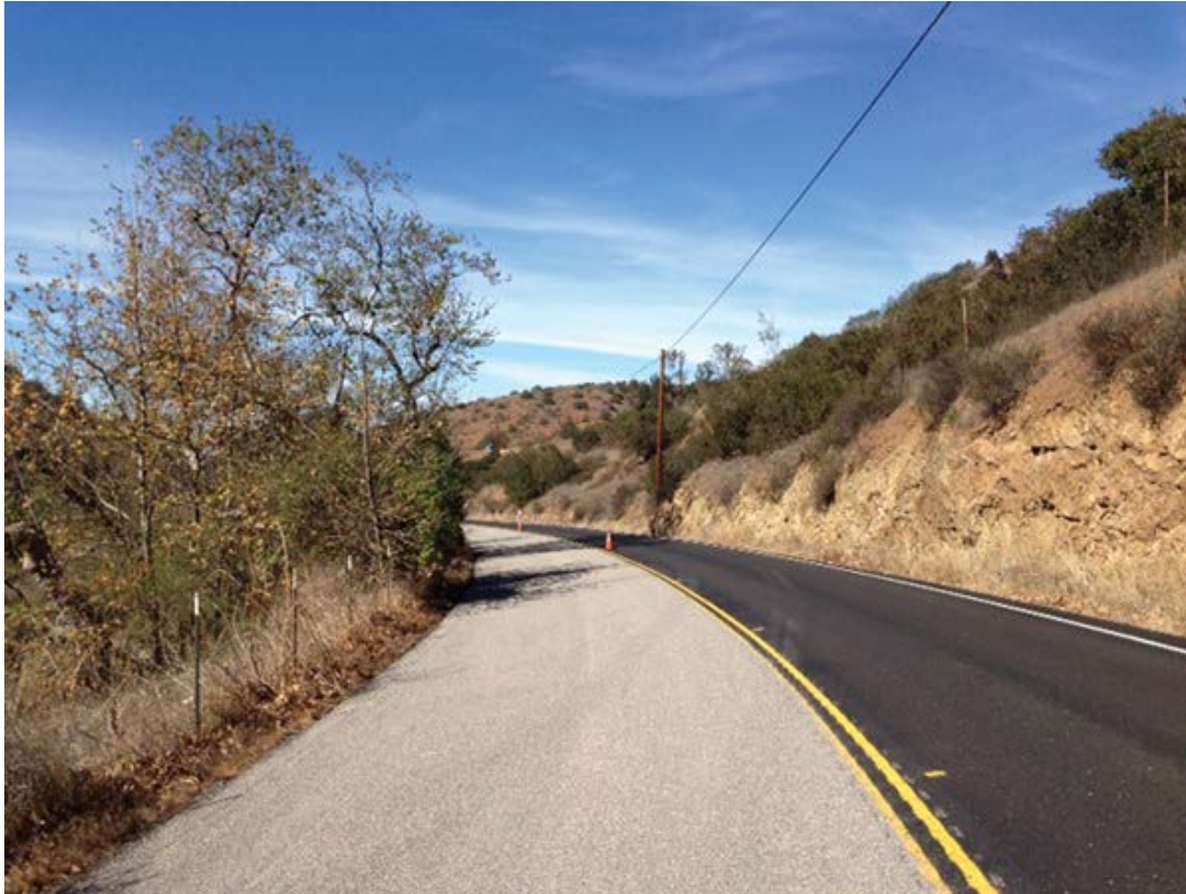
Figure 17. High-Friction Surface Treatment on a Horizontal Curve (53).
