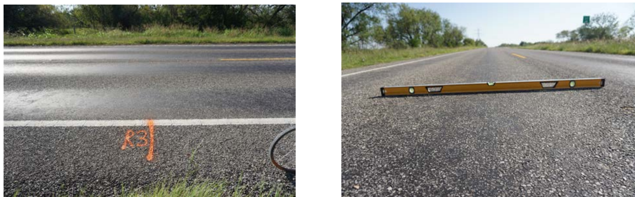
Figure 38. Pictures of Pavement Surface and Rutting: (a) No Cracking and (b) Rutting.
