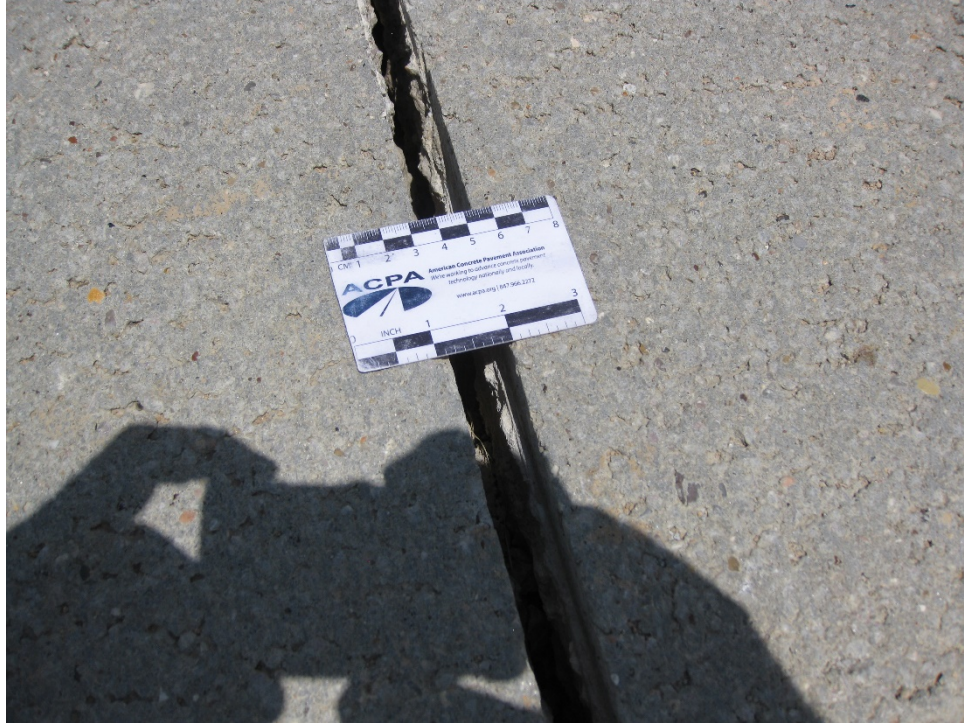
Figure 154. Bella Vista Longitudinal Joint Separation (July 2015).
