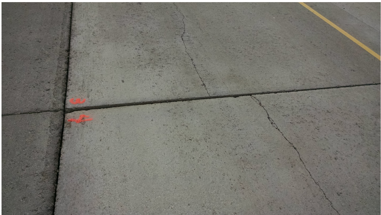
Figure 145. Location 3 and 4 (Joint Separation and Faulting).
