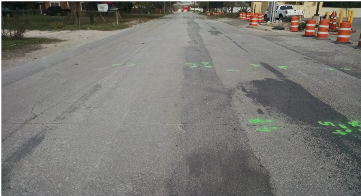
Figure 166. Solms Rd. Longitudinal Joint Spalling and Repair (along with Repair Material Failure).
