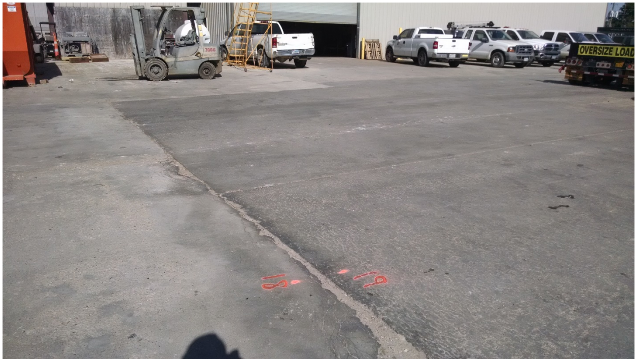
Figure 152. Construction Joint from Transverse to Longitudinal (December 2015).
