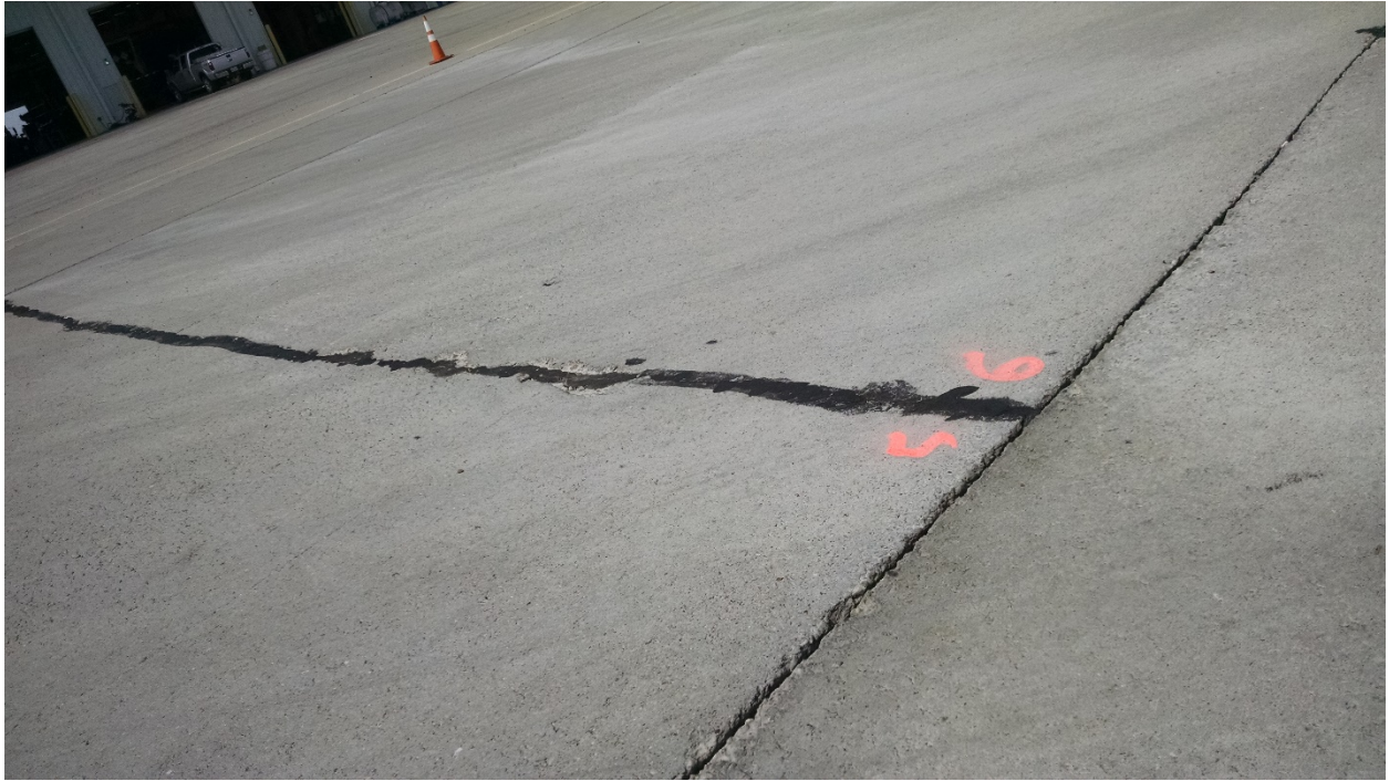
Figure 146. Pioneer Cracked Slab (Repair/Sealed with Asphalt).
