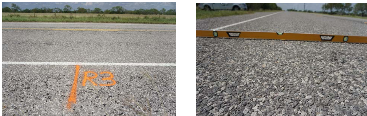
Figure 45. Pictures of Pavement Surface and Rutting: (a) No Cracking and (b) Rutting.
