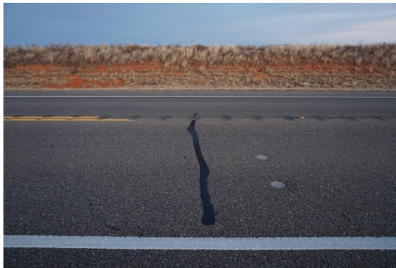
Transverse Cracking: 01/10/2018
