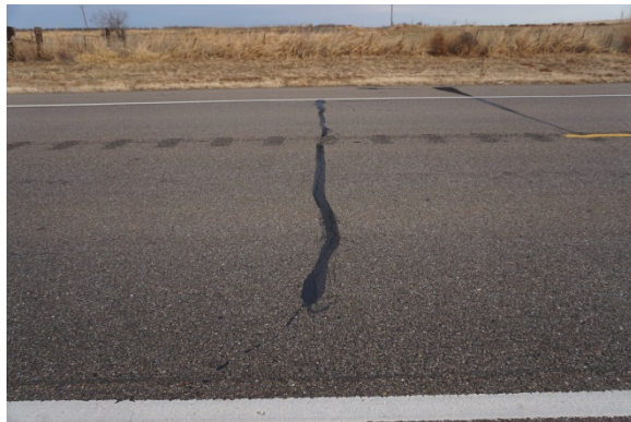
Transverse Cracking: 01/10/2018
