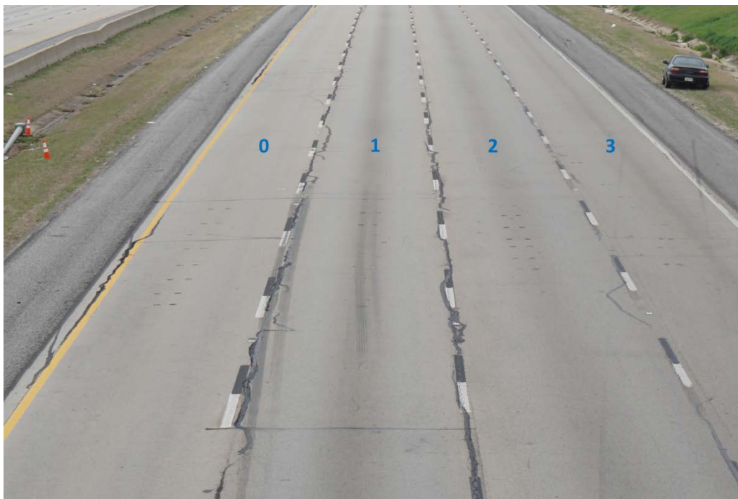
Sections 0 to 3: View from Quebec Bridge on 03/26/2018
