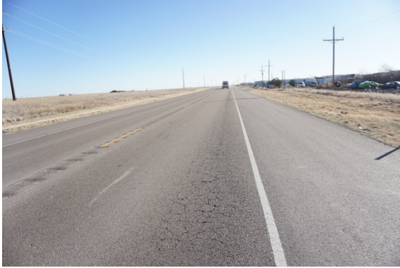
Alligator Cracking: 03/07/2017
