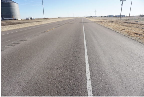
Alligator Cracking: 03/07/2017
