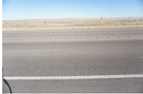
Transverse Cracking: 03/07/2017
