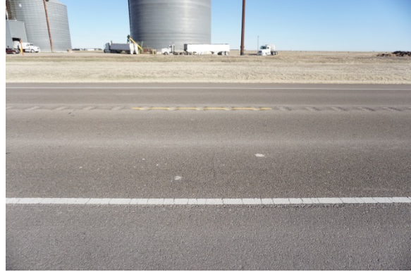
Transverse Cracking: 03/07/2017
