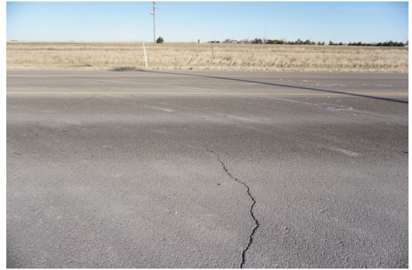
Transverse Cracking: 03/07/2017
