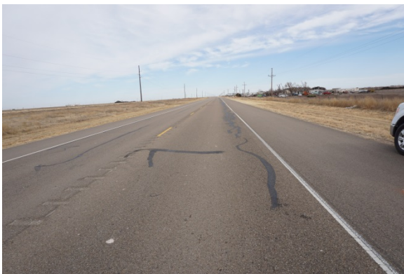
Overall Cracking: 01/10/2018
