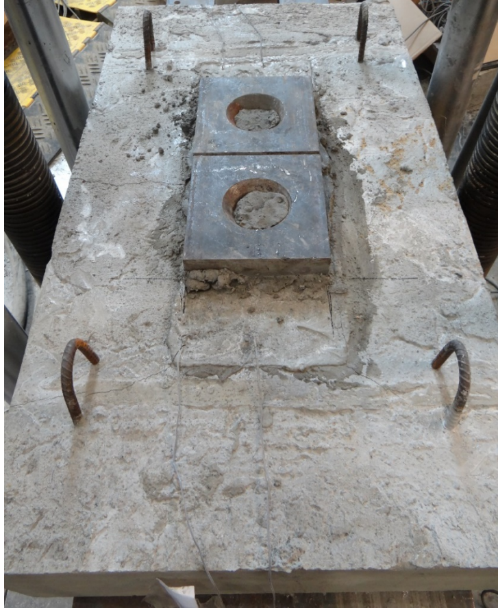
Figure 60. Cracks seen in the outer slab initiating from the interface with the loading plates.
