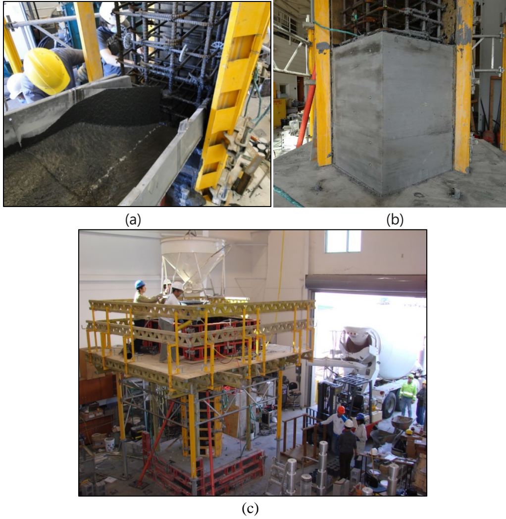
Figure 6. UHP-FRC (a) pouring, (b) completed section, and (c) final casting.
