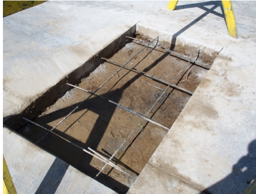
Figure 22. Conventional concrete repair.
