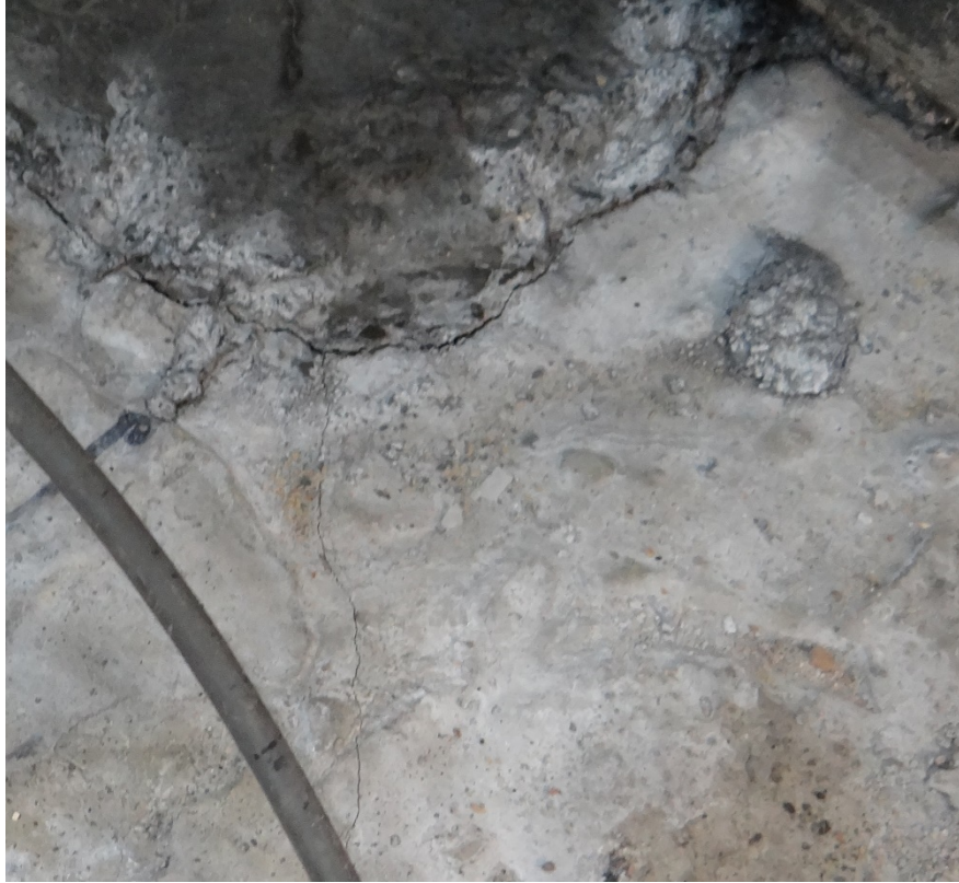
Figure 65. Interface cracks observed in the UHP-FRC punch test specimen after peak.
