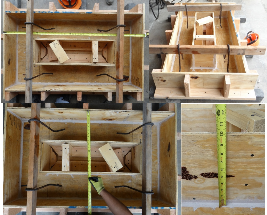
Figure 27. Formwork for the outer hollow slab.
