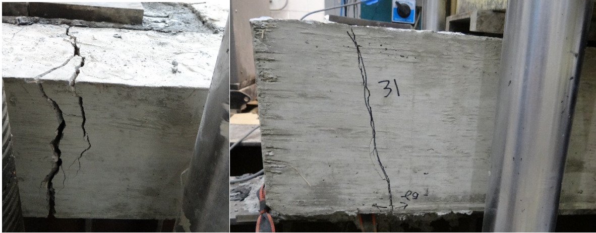
Figure 69. Cracks at the mid-span and the edge of the support outer slab.
