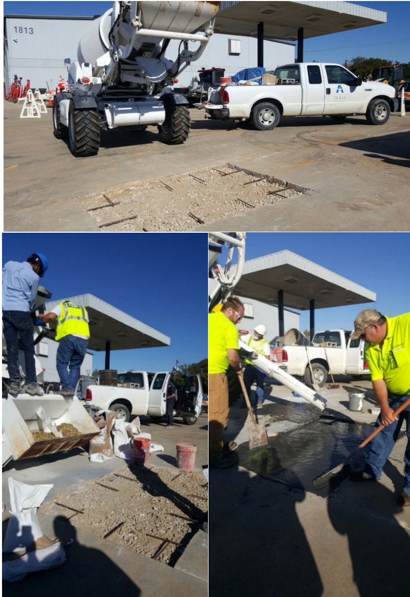
Figure 71. Field installation in the City of Bedford, TX.
