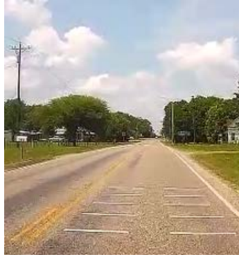
Figure 30. Transverse rumble strips and new reflective striping.
