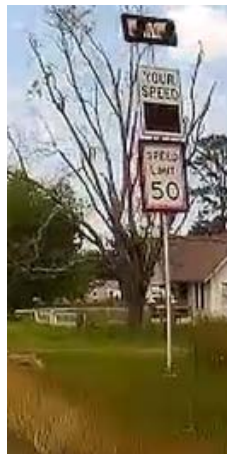
Figure 29. Permanent radar speed detector with active display and speed limit pavement marking.
