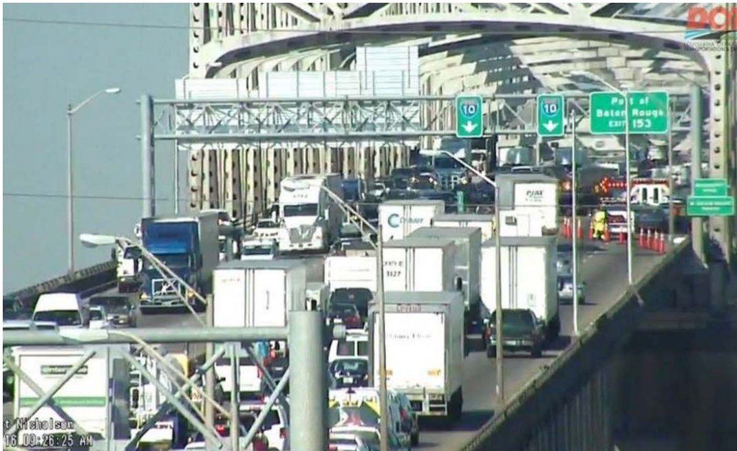
Figure 2. I-10 Mississippi River Bridge.
