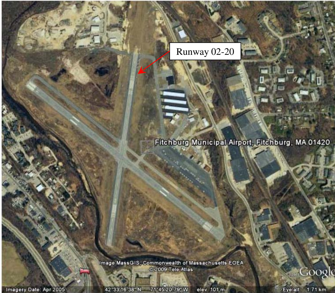
Figure 9. Aerial View of FIT
