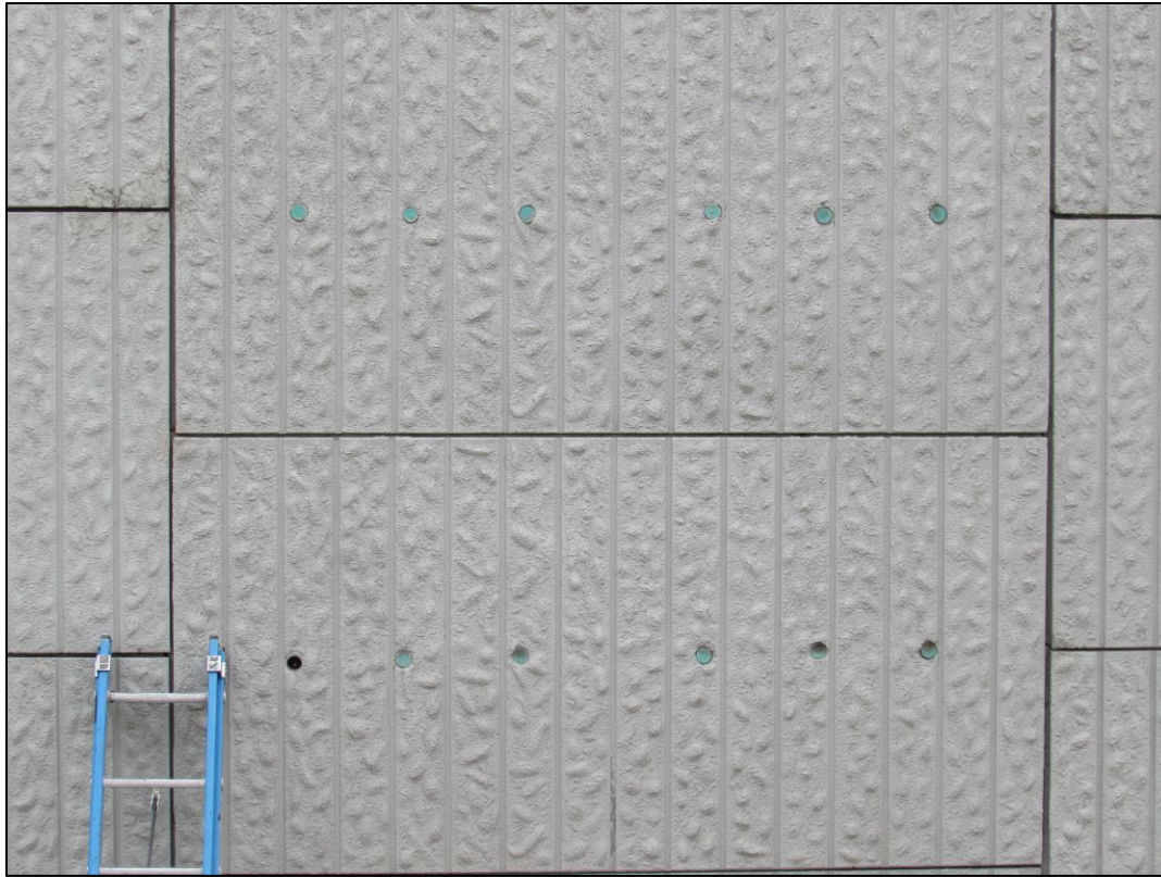
Figure 3-1: Typical MSE Wall Panels with Test Coupons
