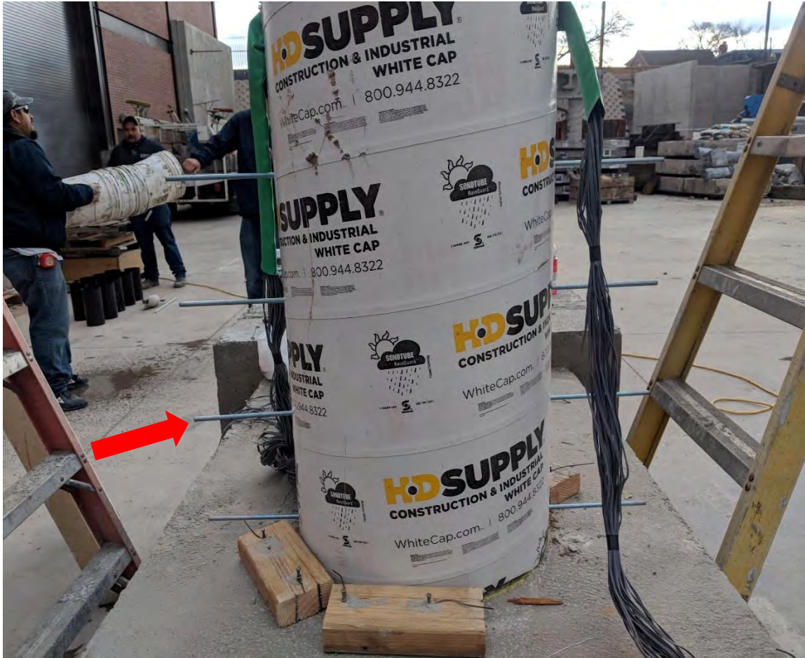
Figure 2.32 Threaded rods for the placement of Novatechniks
