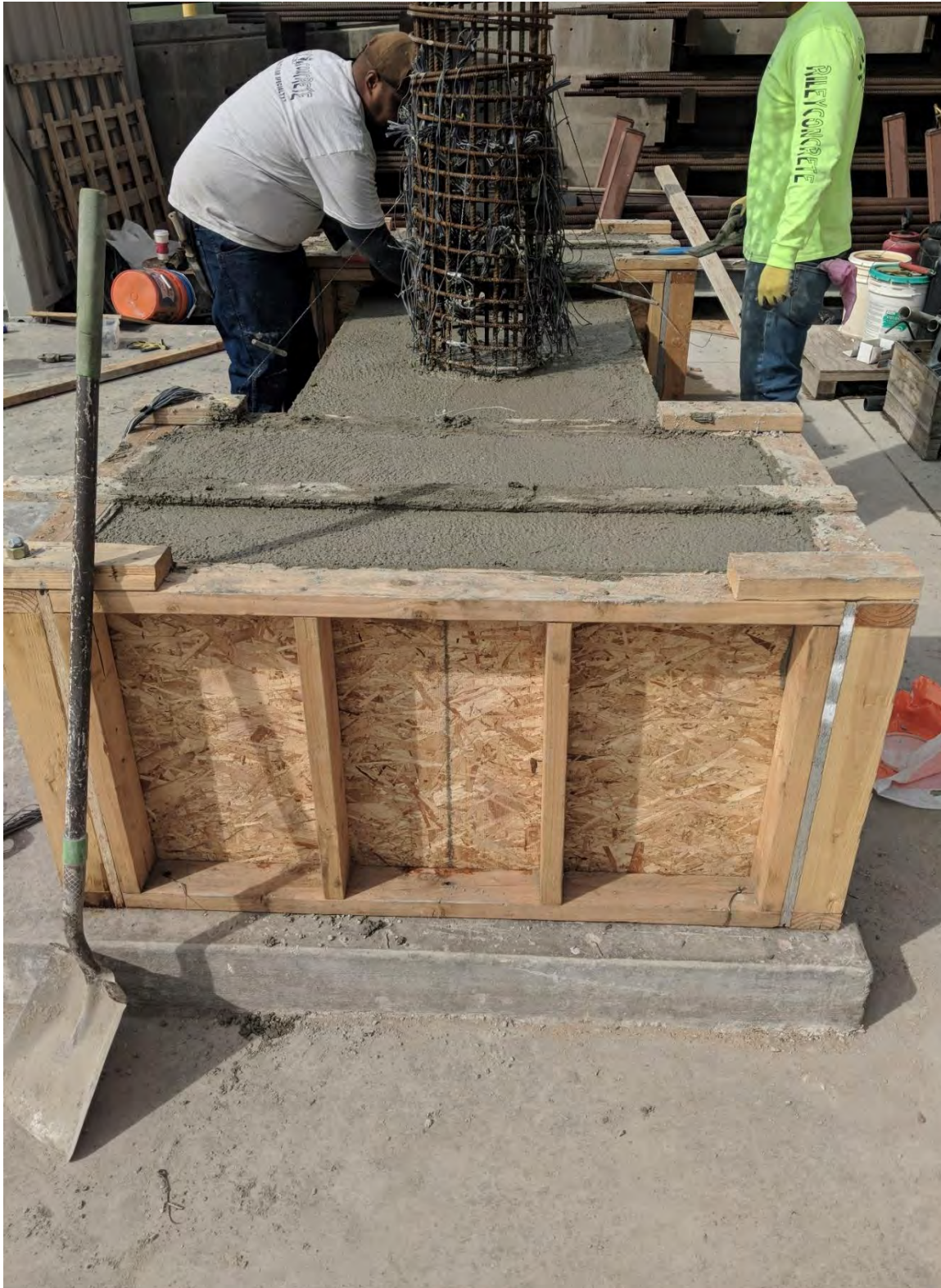
Figure 2.28 Finishing concrete for the cap beam and end blocks
