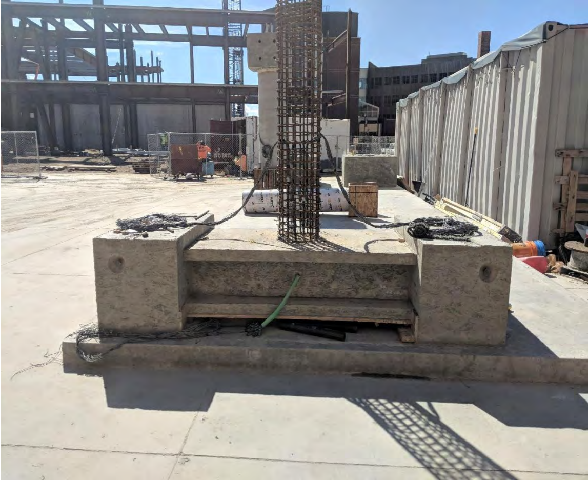
Figure 2.30 Cap beam and end blocks after stripping of formwork
