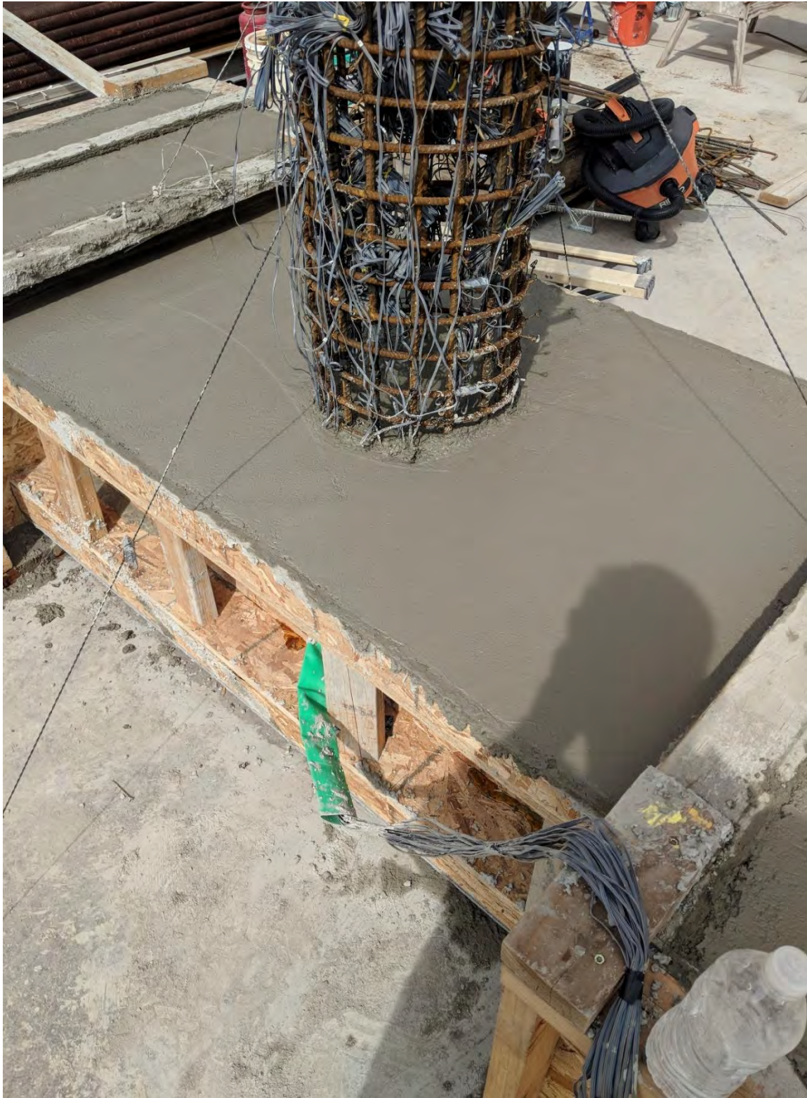
Figure 2.29 Finished concrete surface of the cap beam and end blocks
