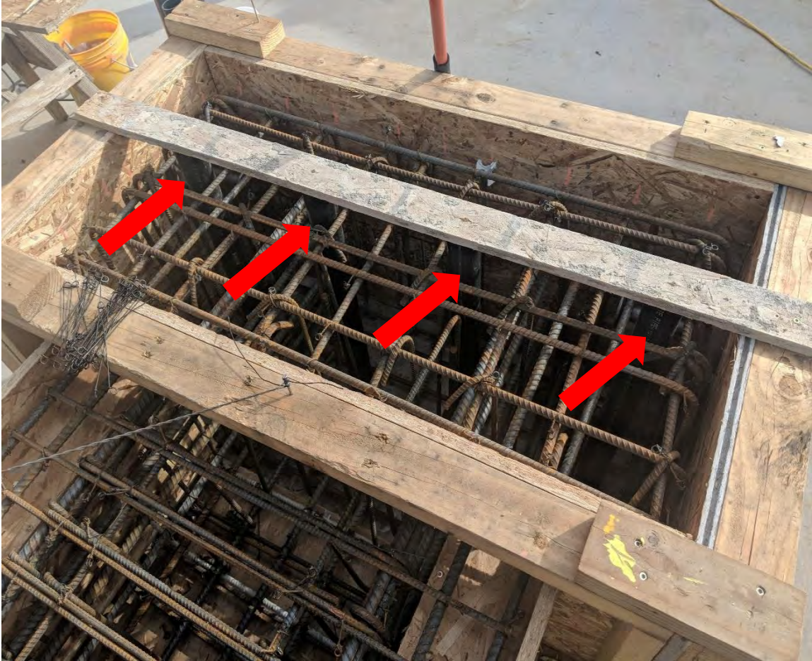
Figure 2.24 PVC pipes placed in an end block
