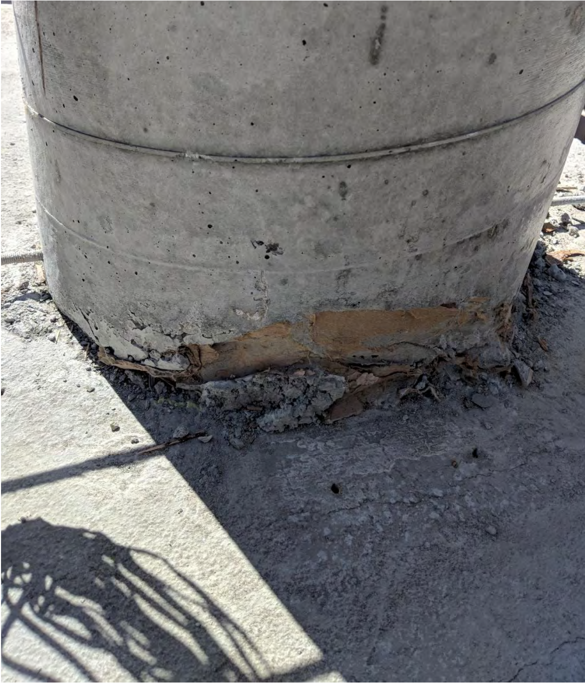
Figure 2.38 Deformed section of column due to Sonotube warping
