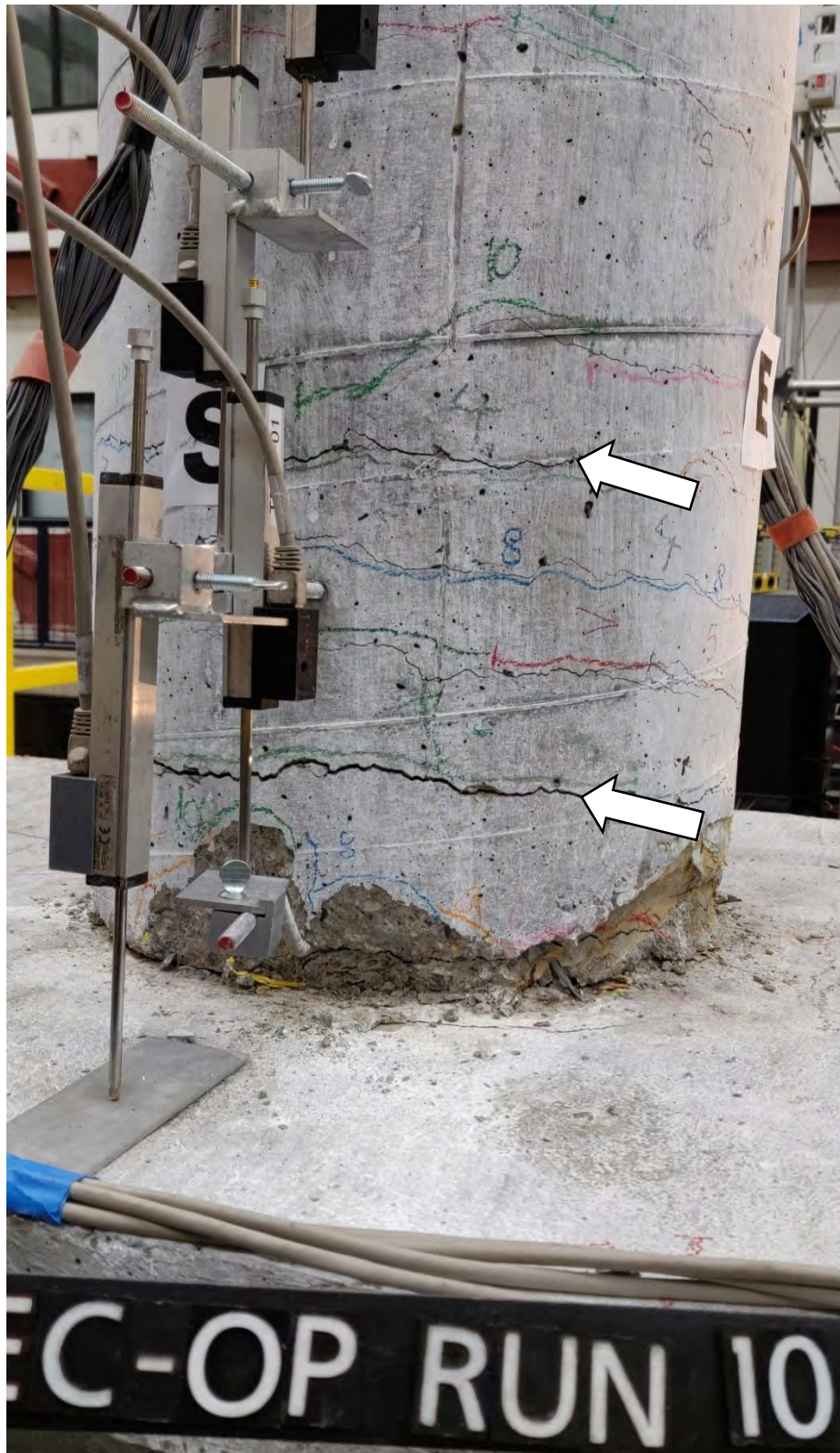
Figure 5.13 Flexural cracks widening after run 10
