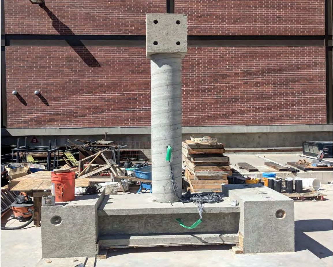
Figure 2.36 Specimen after the removal of all formwork
