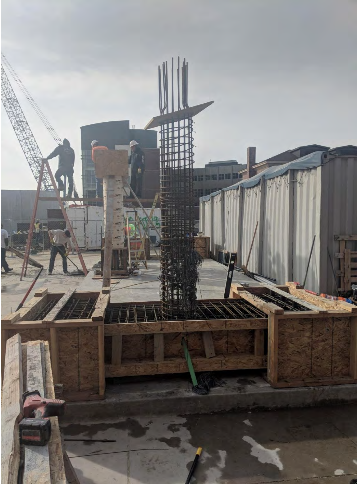
Figure 2.21 Column reinforcement cage placed in pocket
