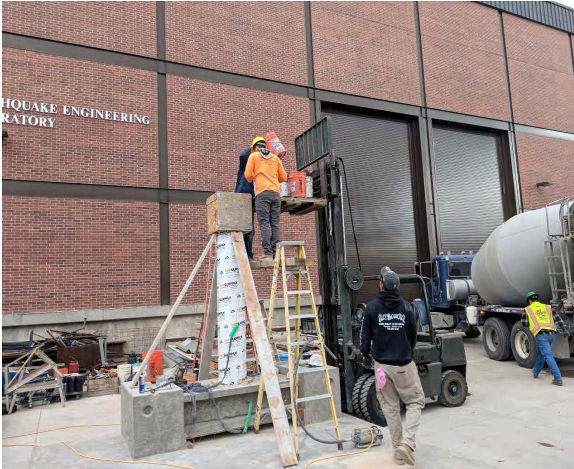
Figure 2.33 Pouring concrete for the column and loading head
