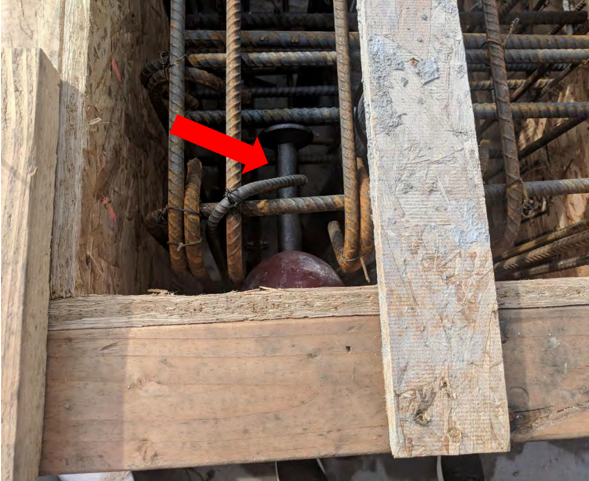
Figure 2.23 One of two lifting anchors placed in each end block
