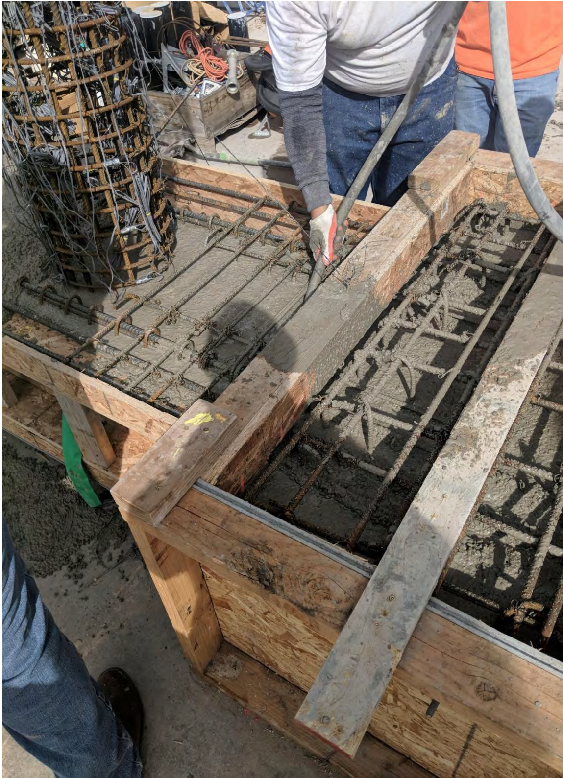
Figure 2.26 Vibrating cap beam concrete
