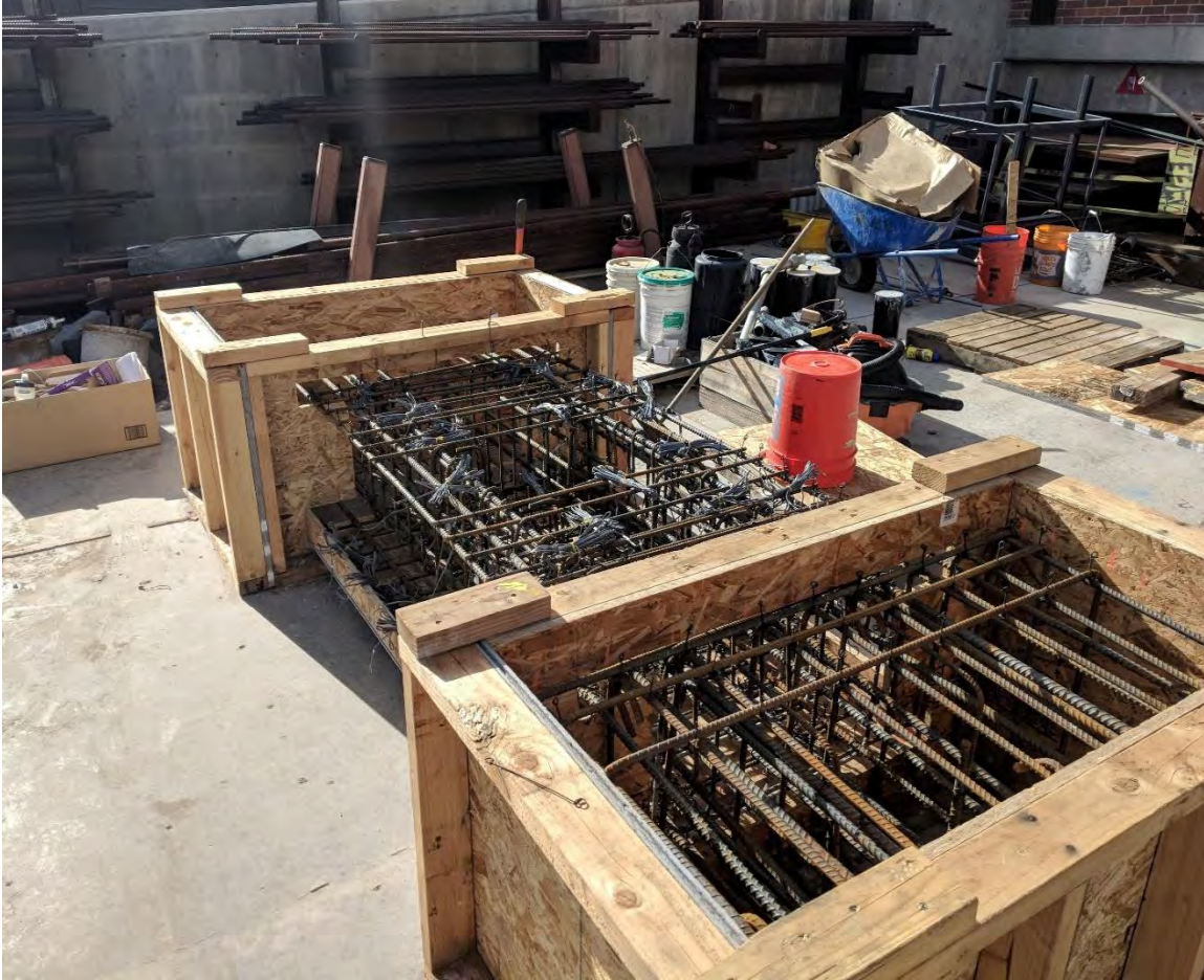
Figure 2.19 Cap beam and end blocks reinforcement cages and forms
