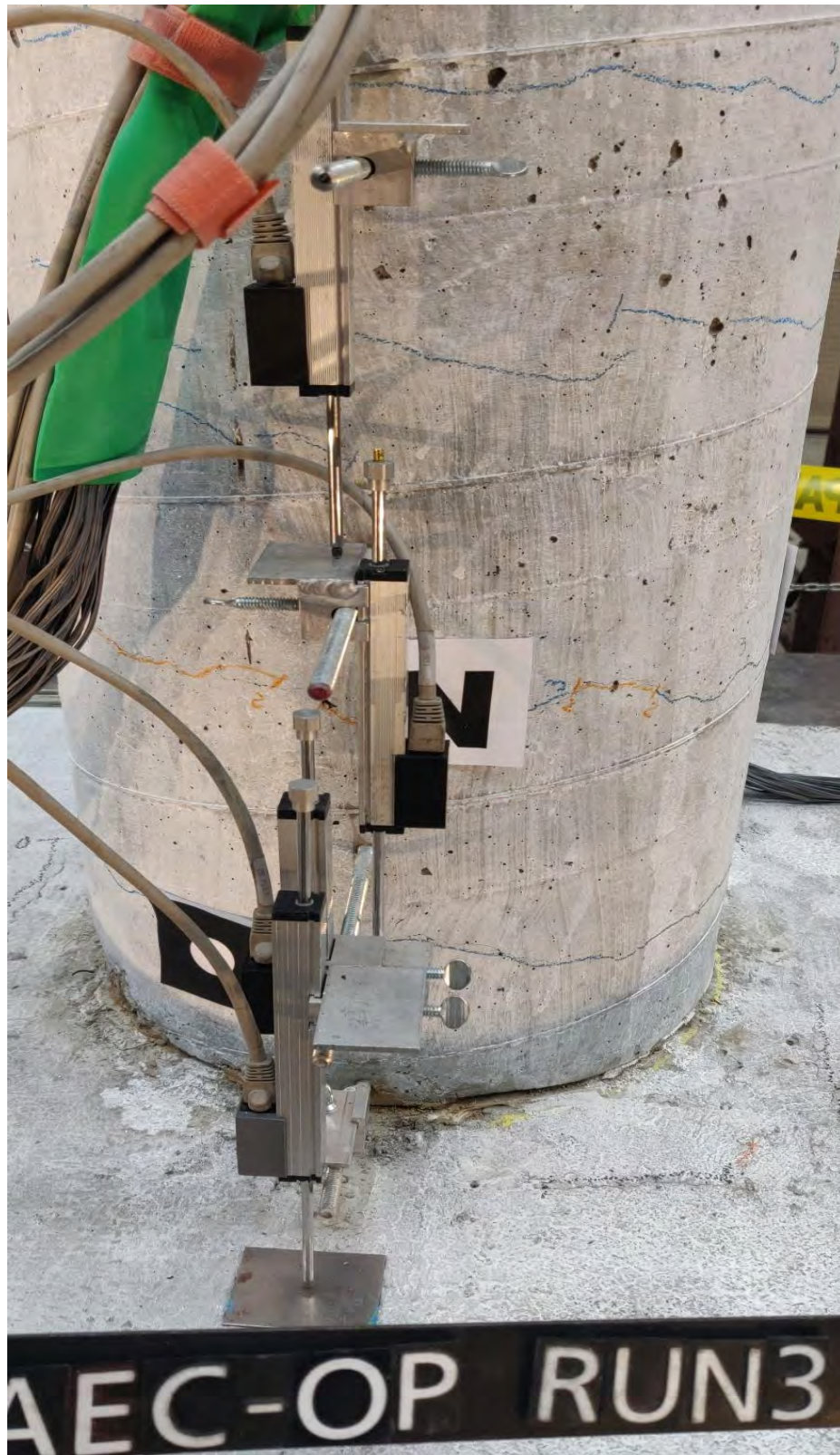
Figure 5.3 Flexural cracks on column north side after run 3
