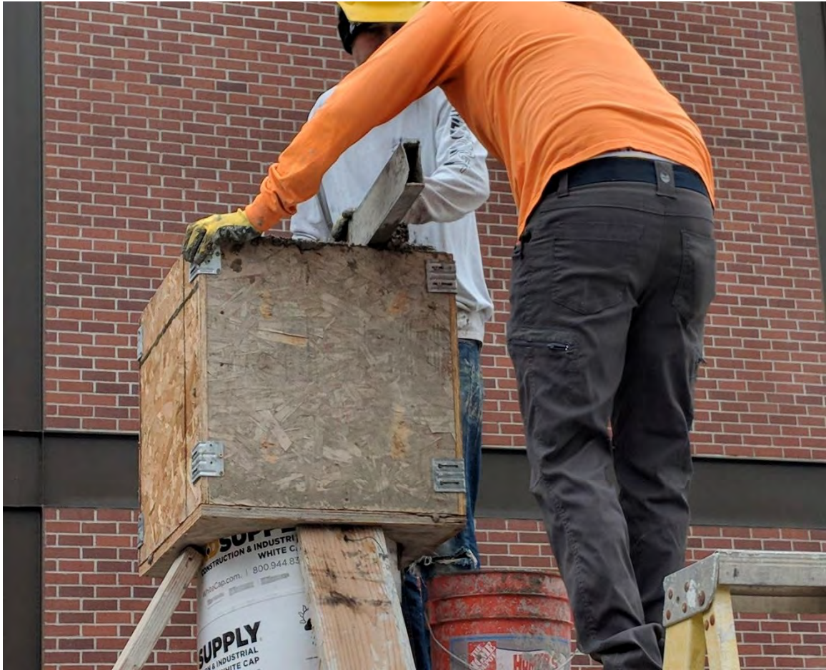
Figure 2.35 Finishing the surface of the loading head
