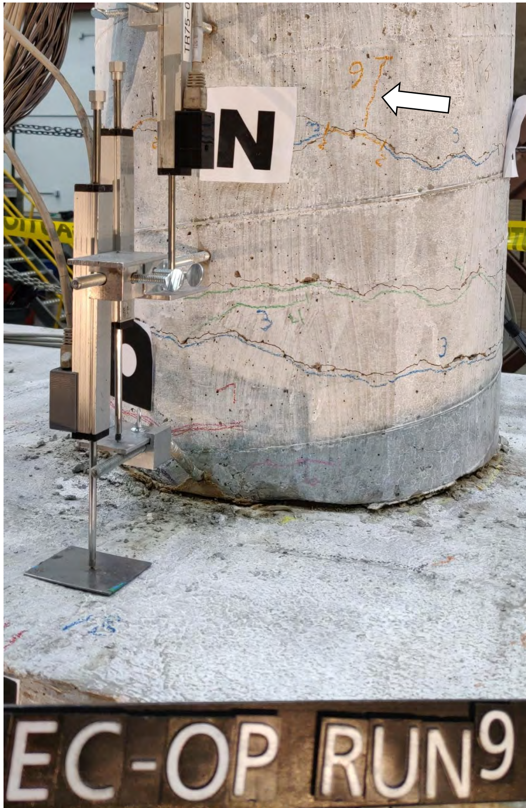
Figure 5.11 Shear crack on column north side after run 9
