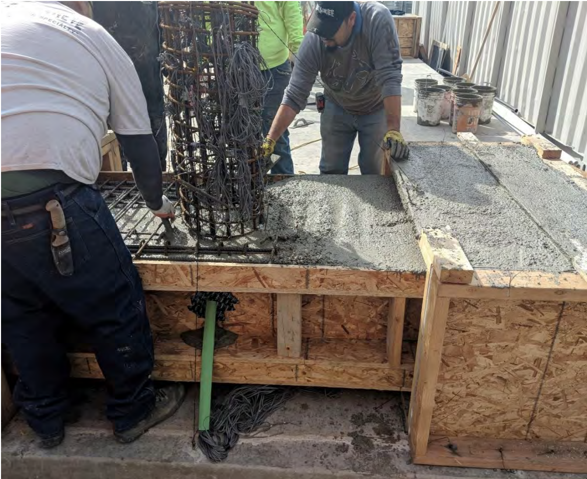
Figure 2.27 Vibrating concrete around column to cap beam joint
