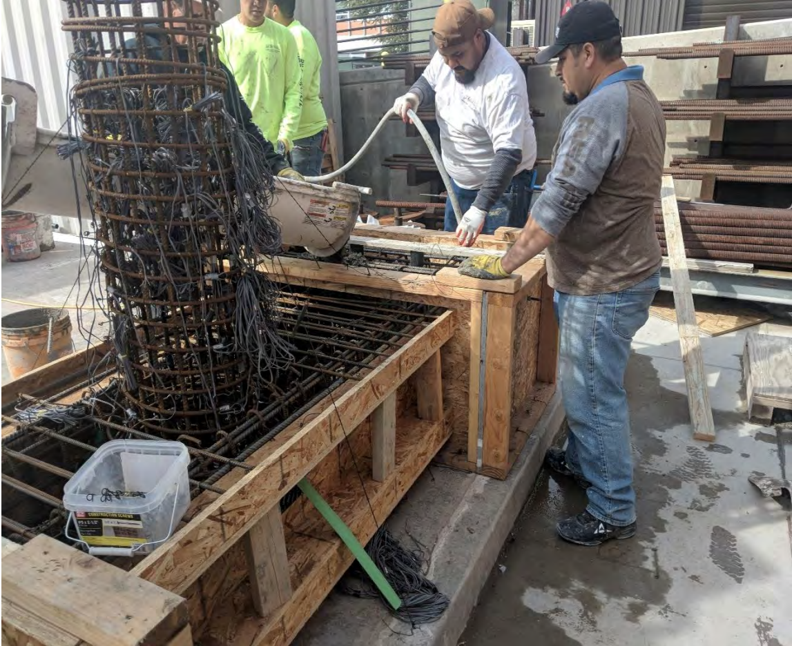
Figure 2.25 Pouring and vibrating concrete in an end block
