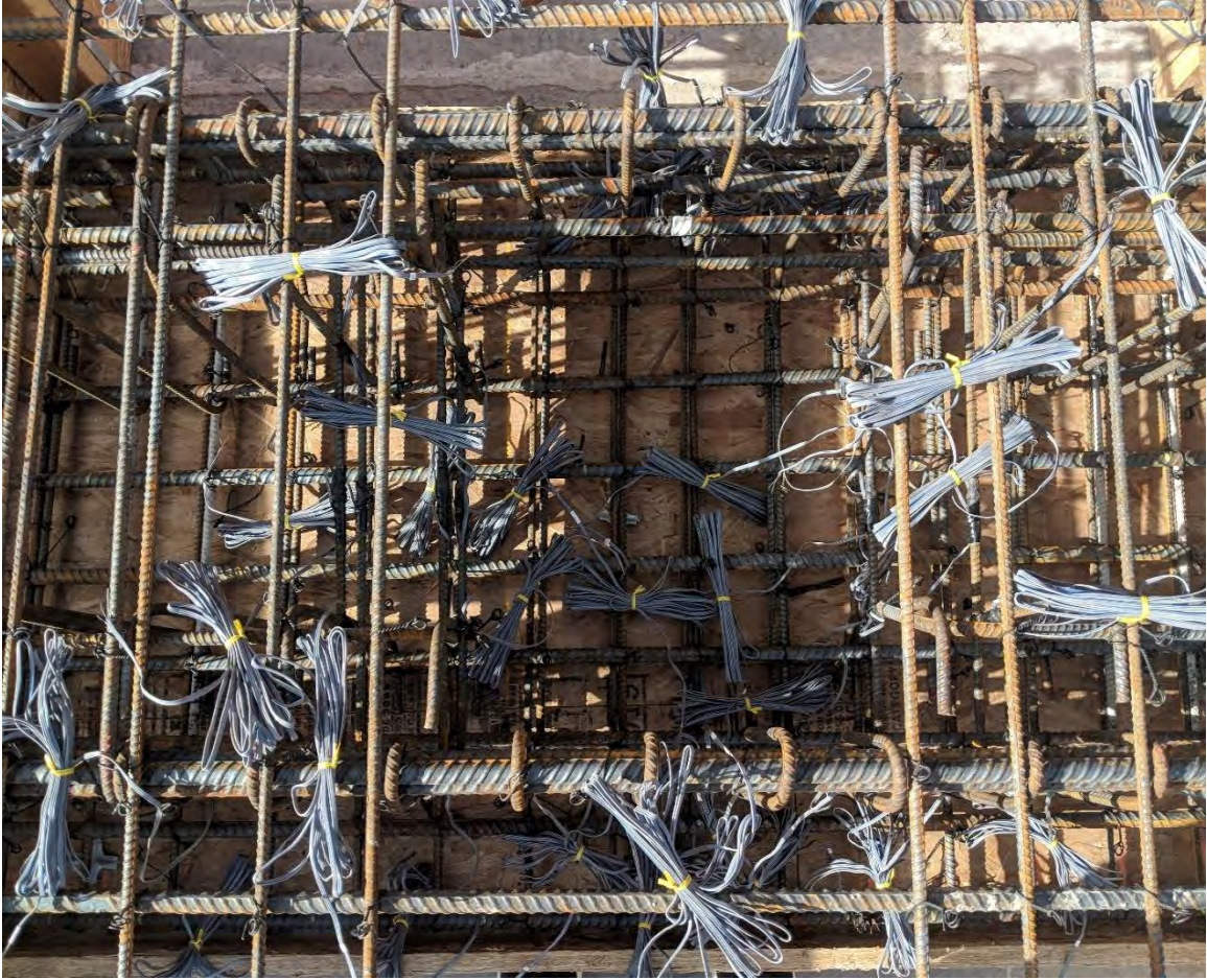
Figure 2.20 Joint reinforcement creating cast-in-place pocket
