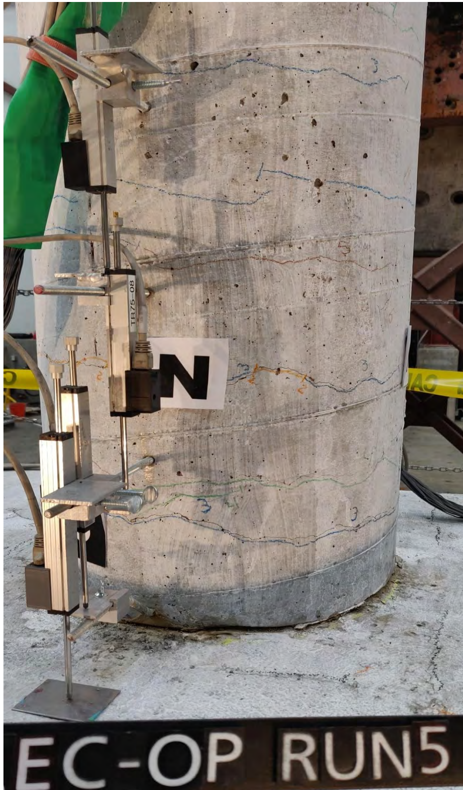
Figure 5.5 Flexural cracks on column north side after run 5
