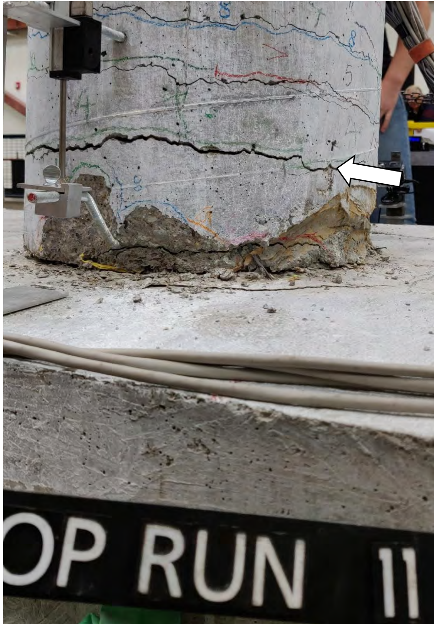
Figure 5.16 Widened flexural crack on column south side after run 11 (final run)
