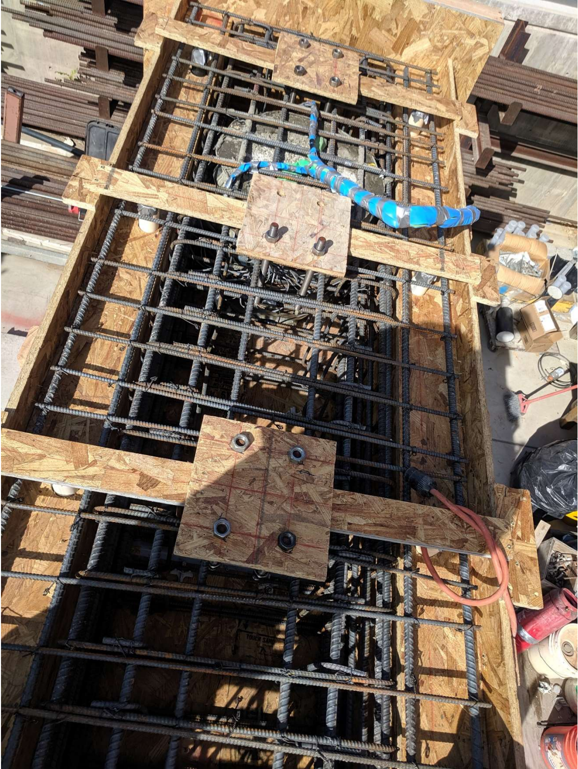
Figure 2.49 Completed cap beam reinforcement
