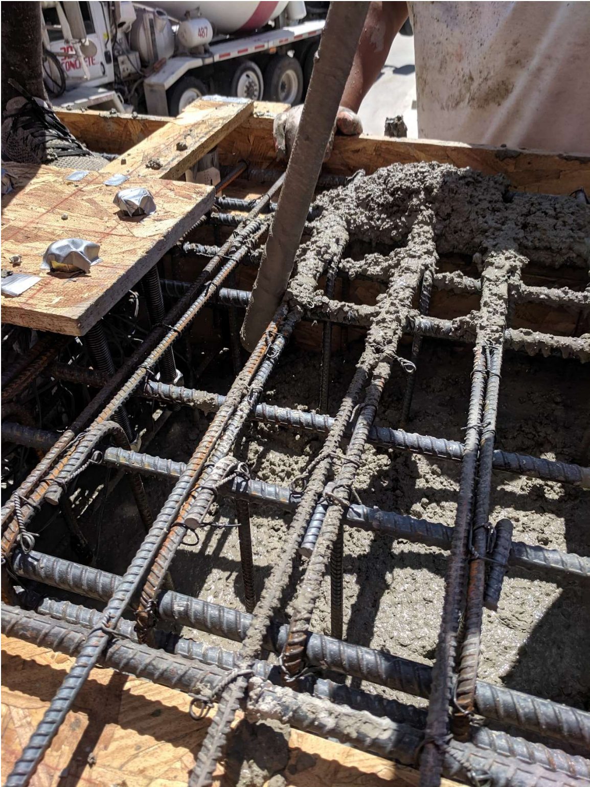
Figure 2.52 Vibrating of cap beam concrete
