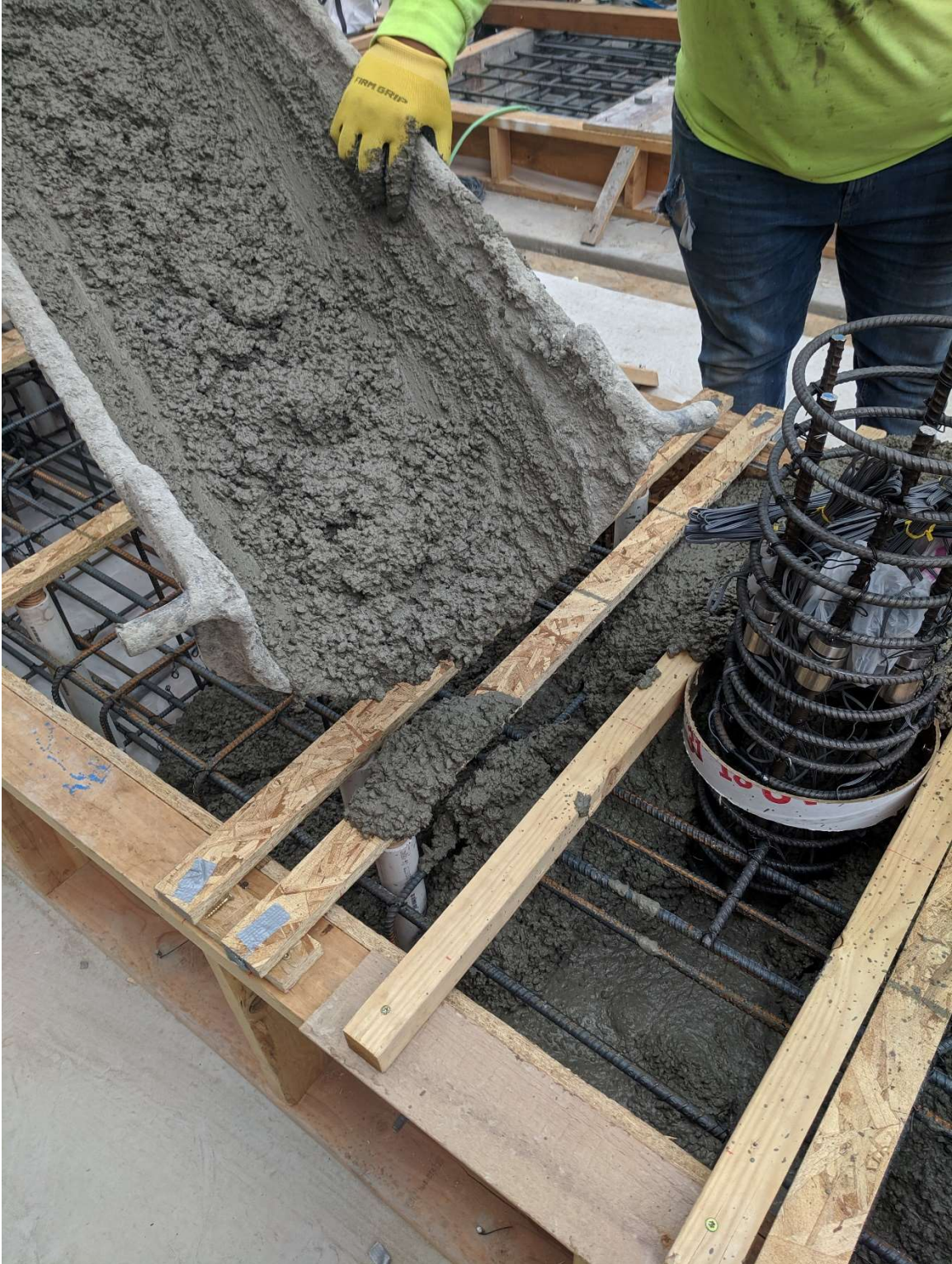
Figure 2.35 Pouring of footing concrete
