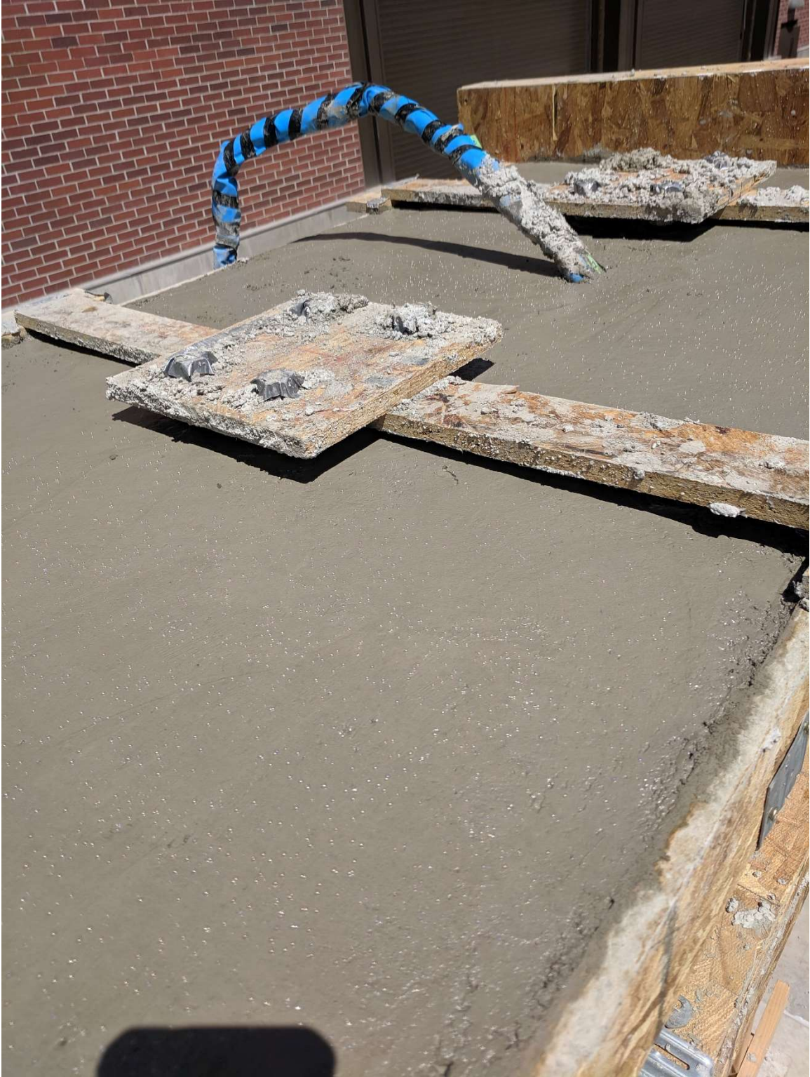
Figure 2.53 Finished cap beam concrete
