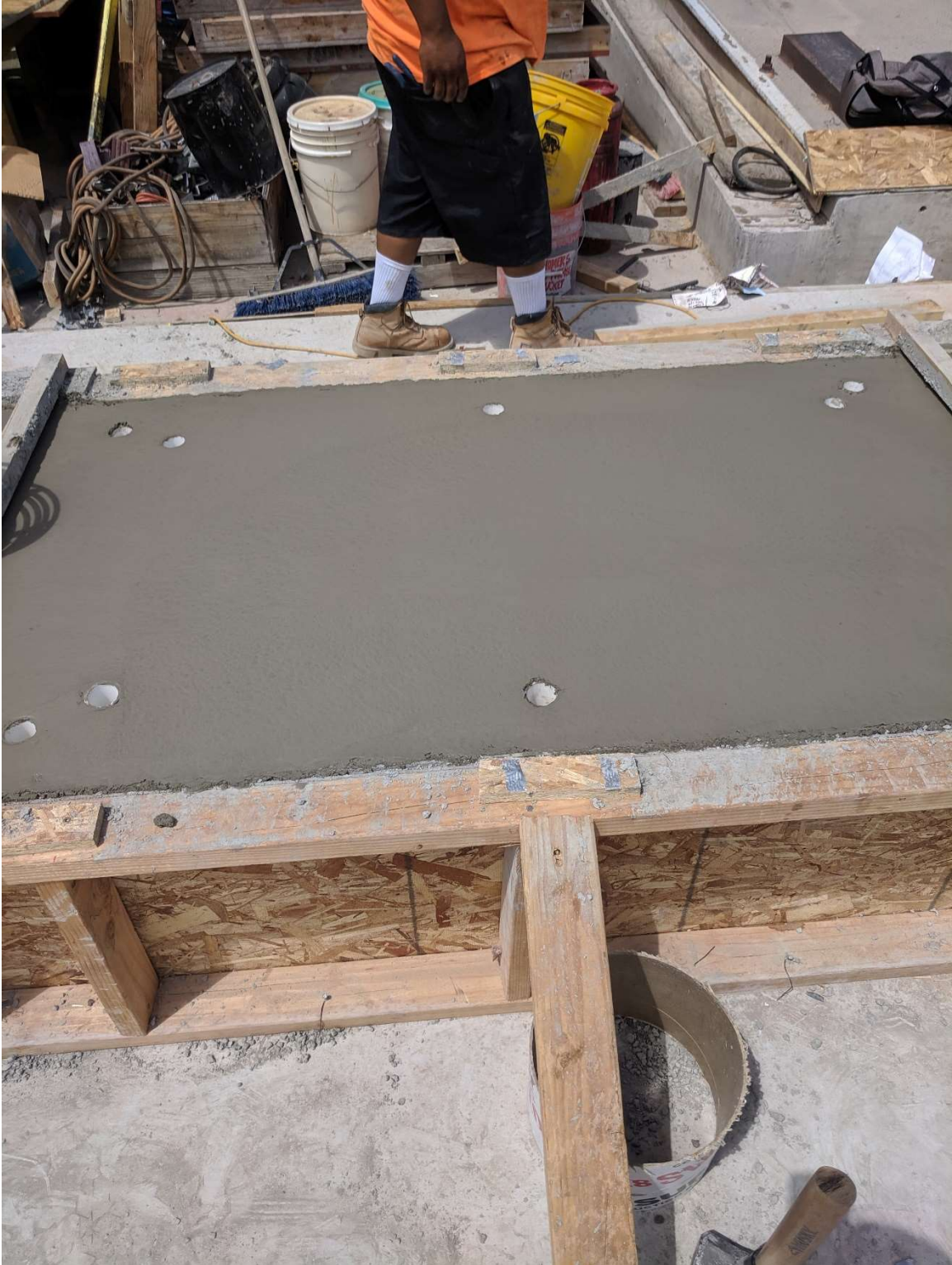
Figure 2.37 Finished footing concrete
