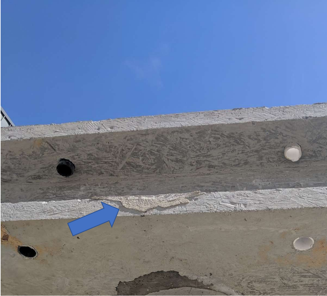
Figure 2.56 Repaired cap beam flange rebar exposure
