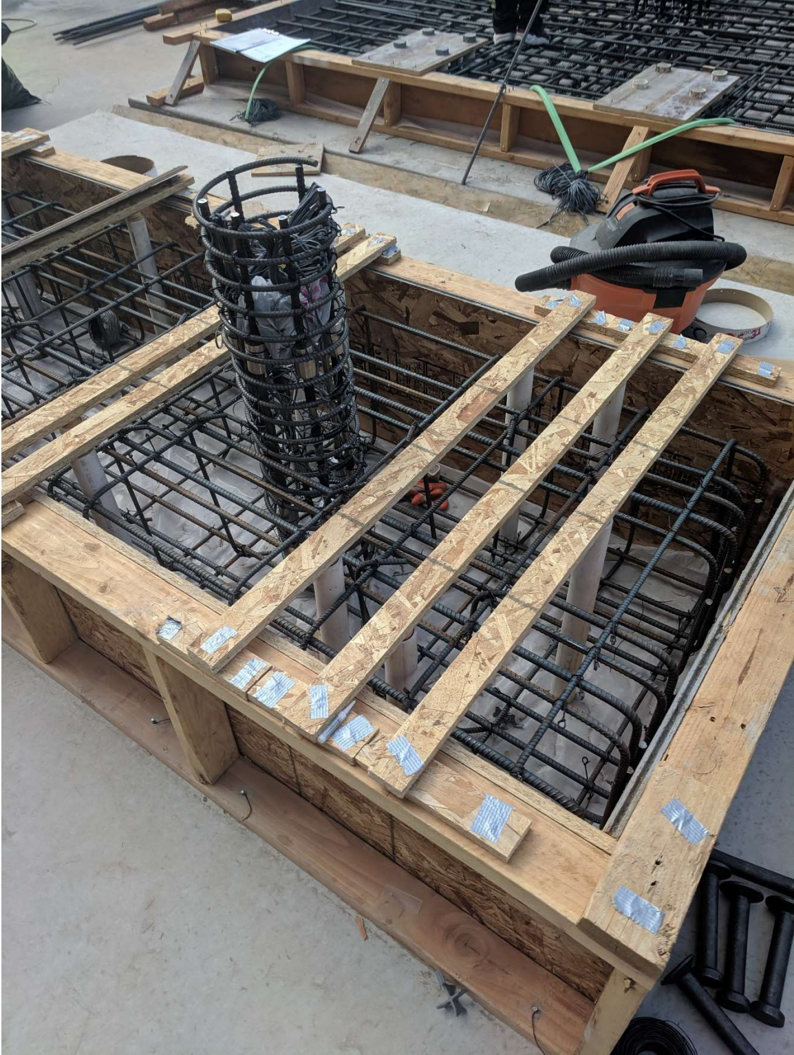
Figure 2.29 Hinge reinforcement cage residing in footing reinforcement
