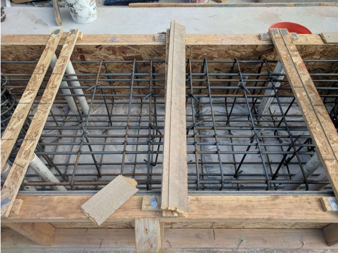
Figure 2.28 Footing reinforcement
