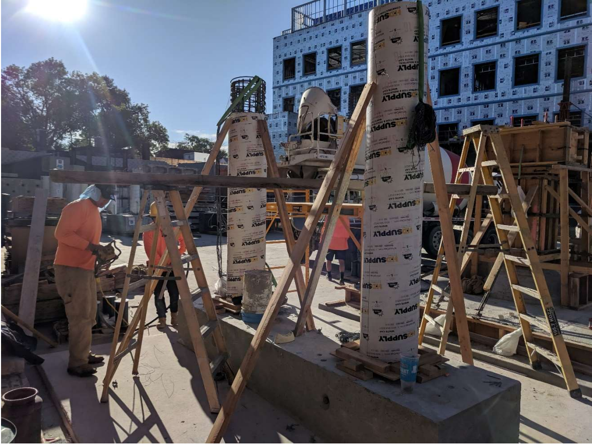
Figure 2.41 Erected column cages and Sonotube
