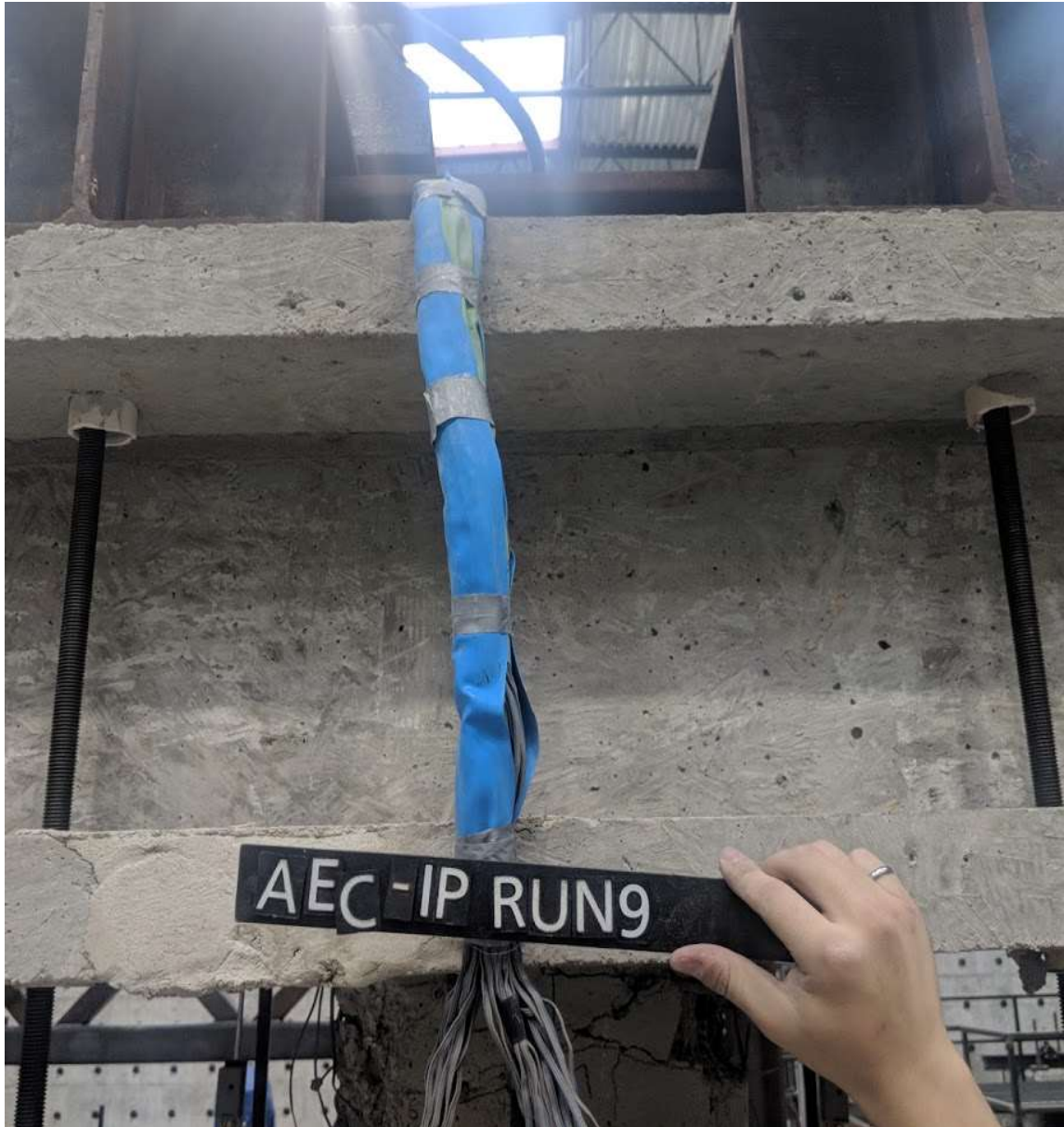
Figure 5.22 Run 9 – Absence of cracks on south column-cap joint (ABC – W face)
