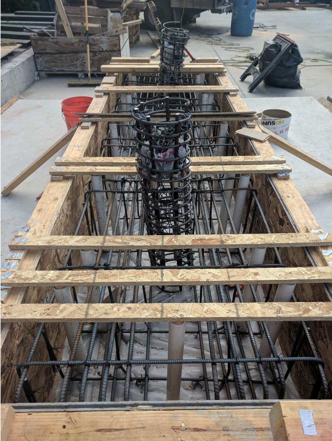
Figure 2.34 PVC pipes within footing
