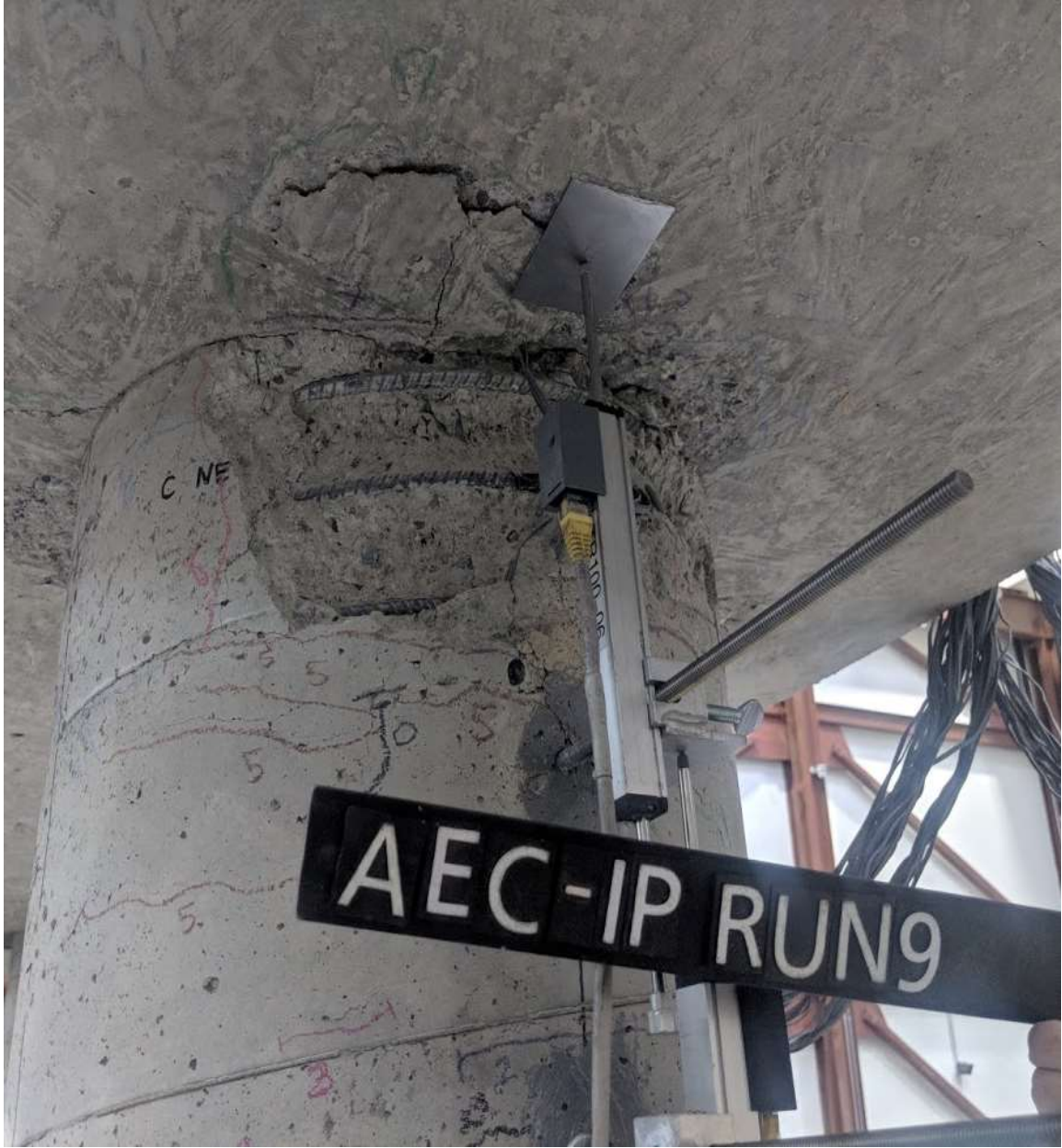
Figure 5.41 Run 9 – Progression of column and cap beam spalling (CIP – N face)
