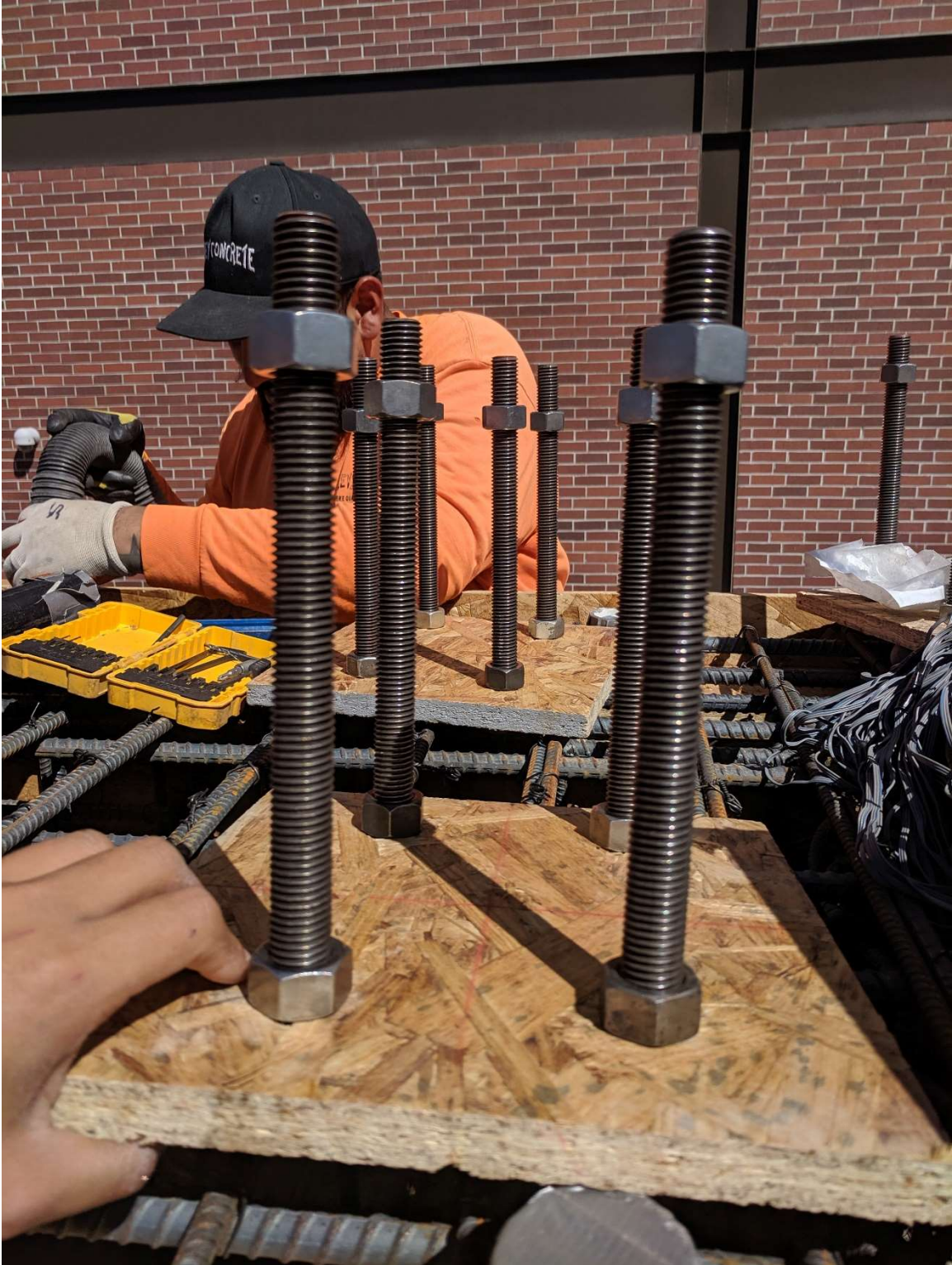
Figure 2.50 Group of \frac{3}{4} " (19 mm) steel studs.
