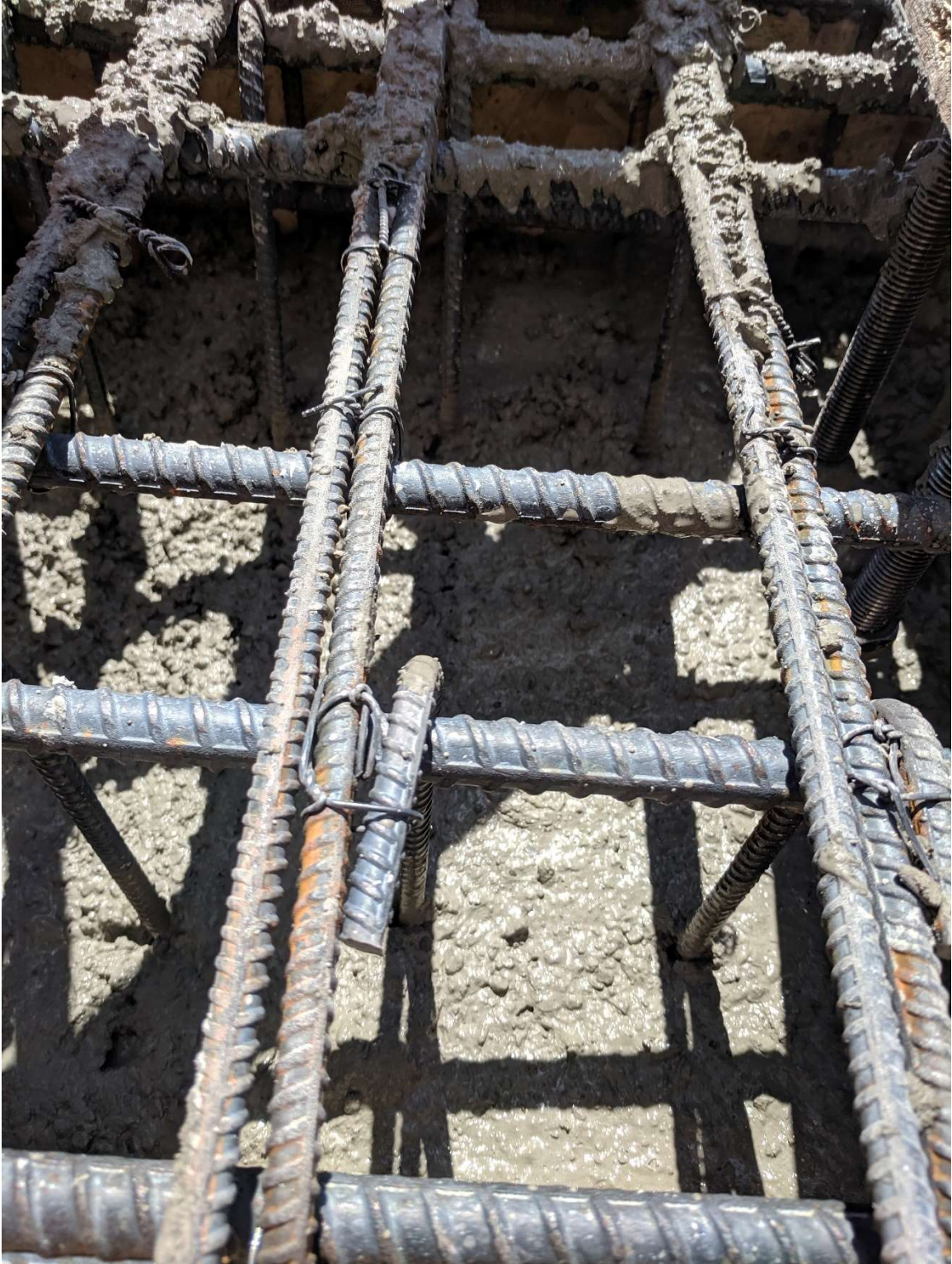
Figure 2.51 Pouring of cap beam concrete
