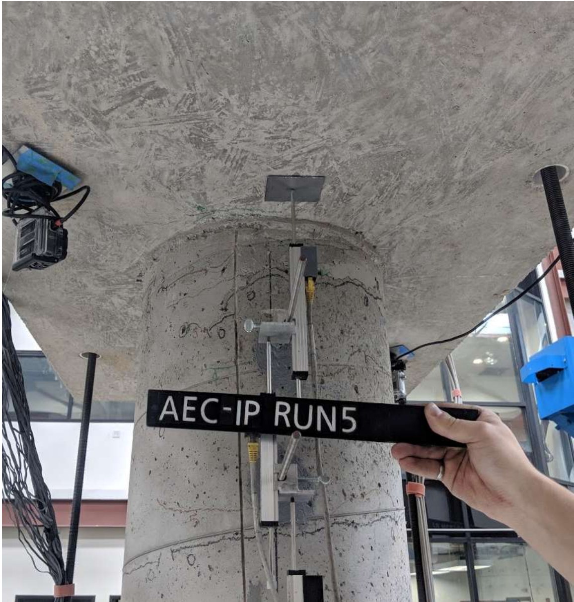
Figure 5.32 Run 5 – Appearance of several flexural cracks (CIP – S face)
