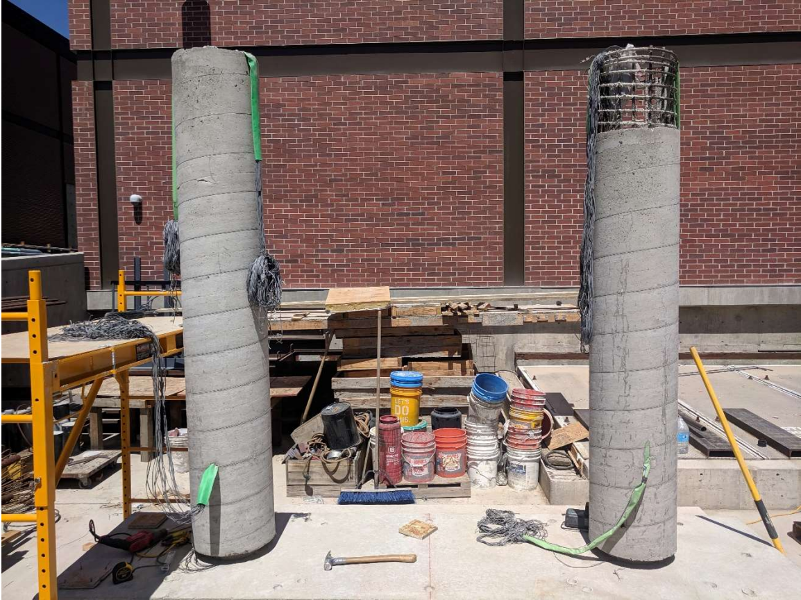
Figure 2.43 Columns stripped of their formwork
