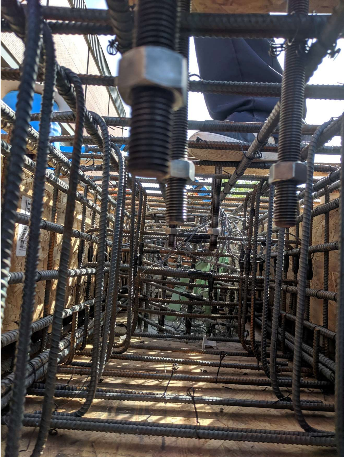
Figure 2.46 CIP column reinforcement cage passing into cap beam pocket unobstructed
