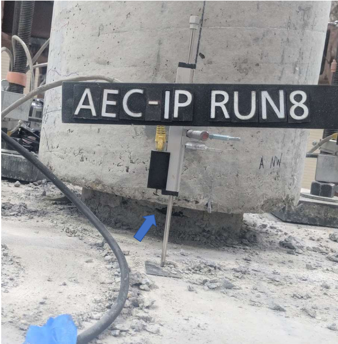
Figure 5.13 Run 8 – Exposure of two-way hinge reinforcement (ABC - N face)
