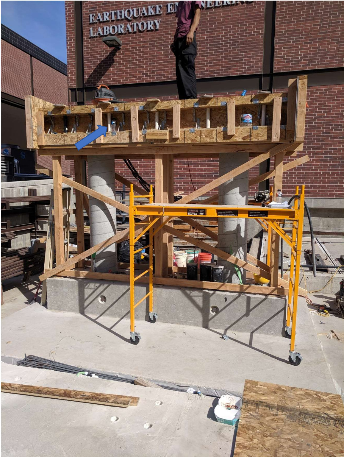
Figure 2.48 Completed cap beam formwork and PVC pipes
