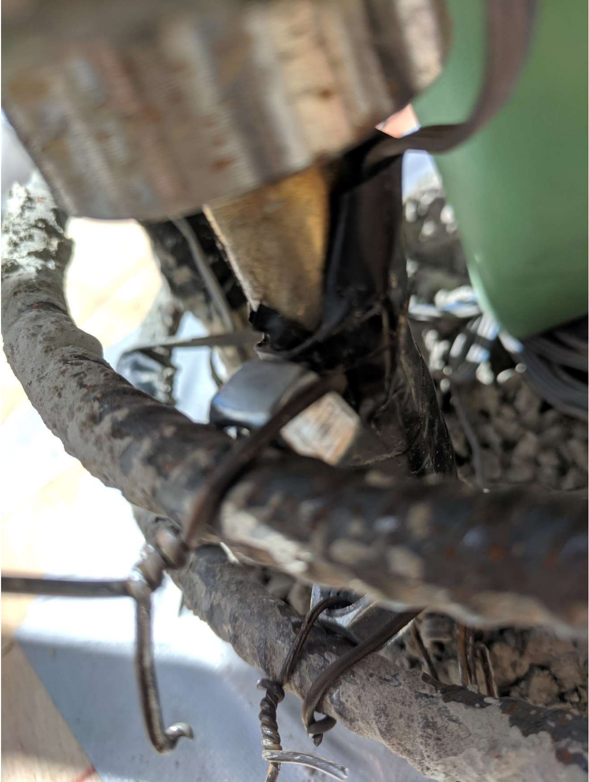
Figure 2.32 High strength steel nut placed in gap between CAM bar and hinge spiral
