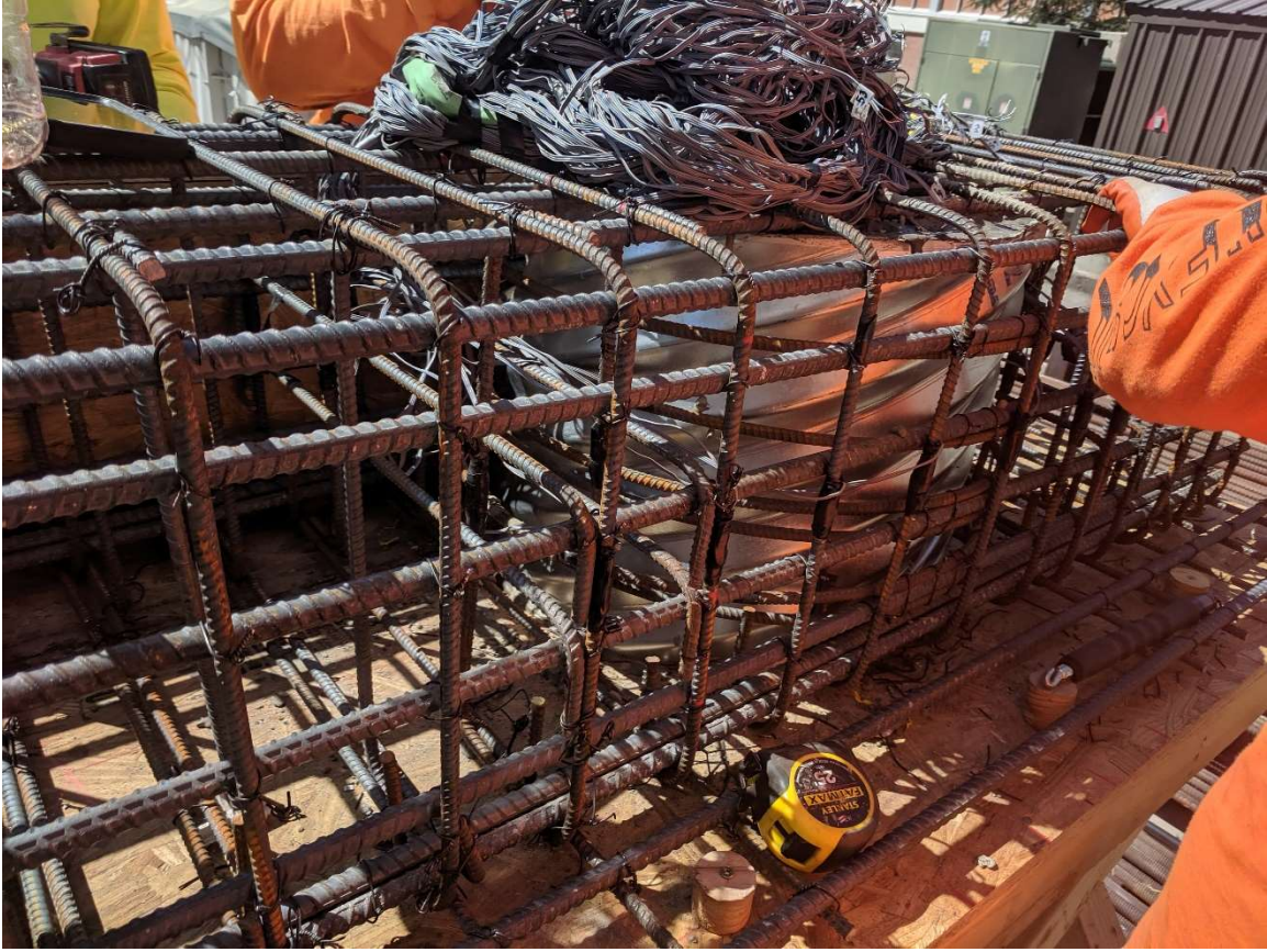
Figure 2.45 Tying of bottom and middle cap beam reinforcement
