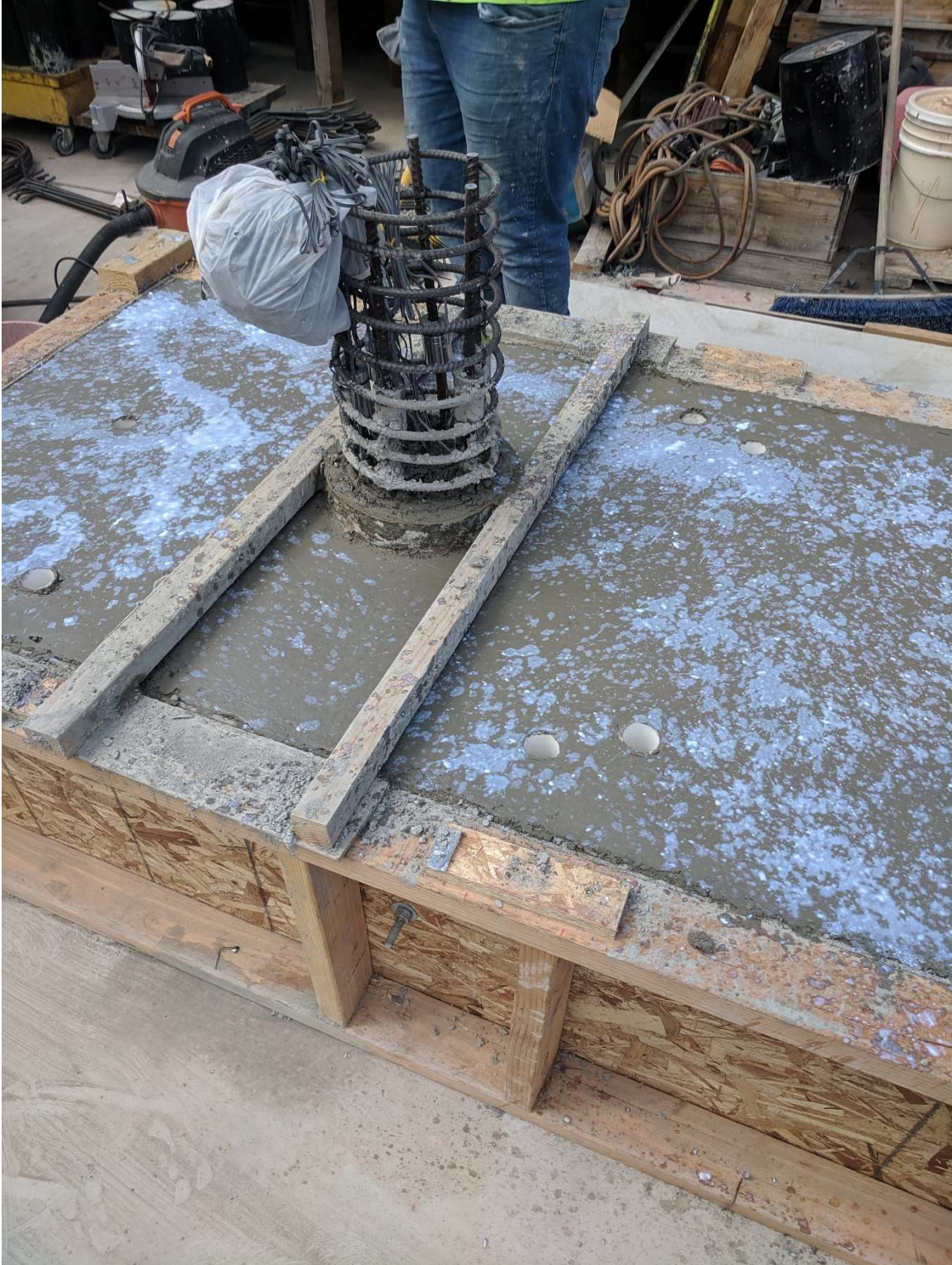
Figure 2.38 Water based cure spread on finished concrete
