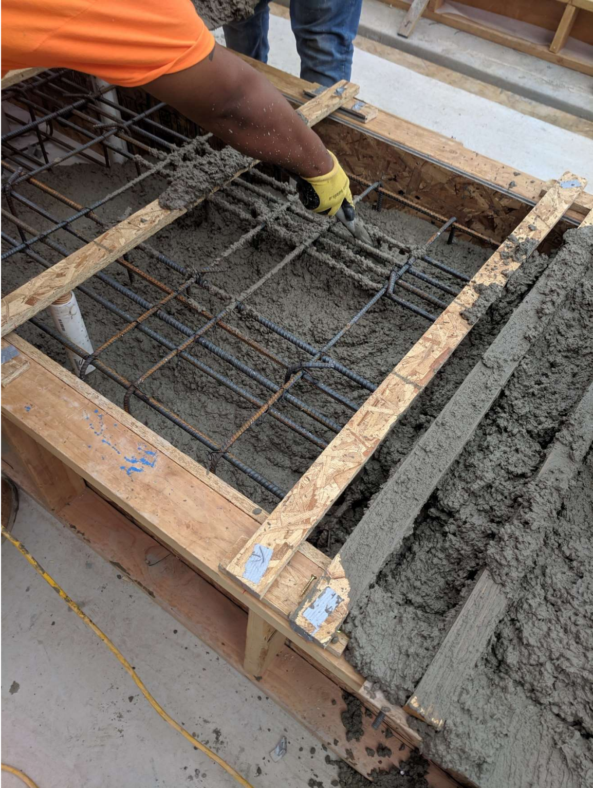
Figure 2.36 Vibrating of footing concrete
