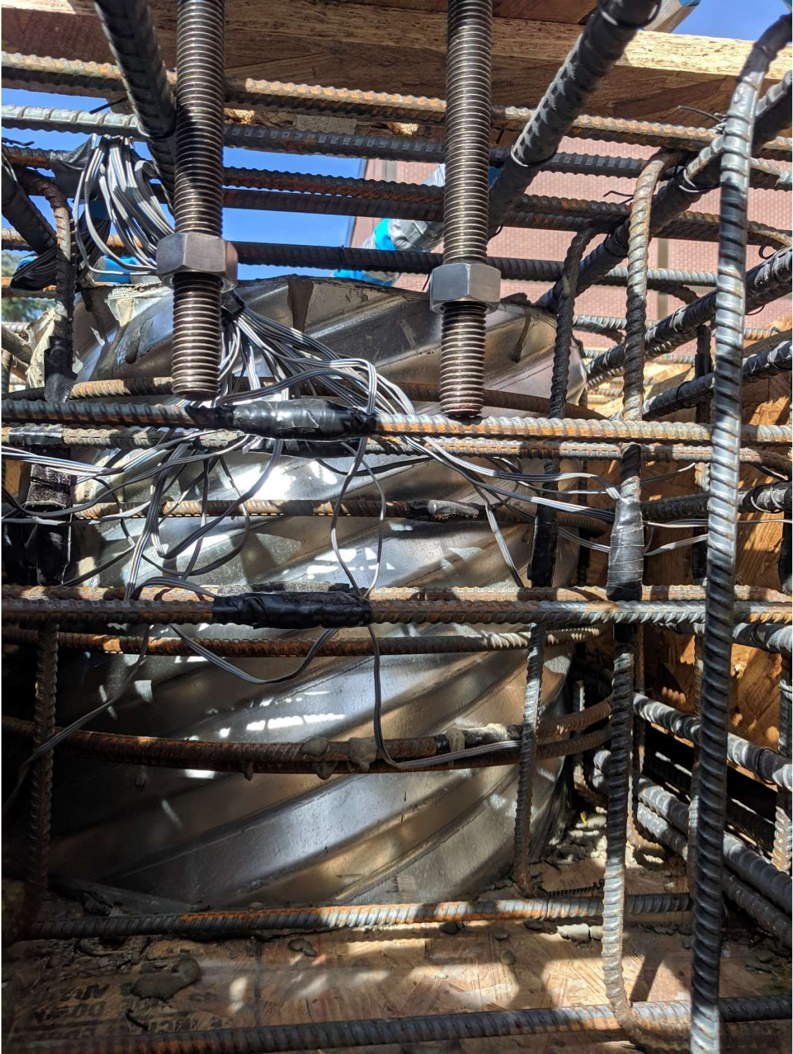
Figure 2.47 ABC column and CMP passing into cap beam pocket unobstructed.
