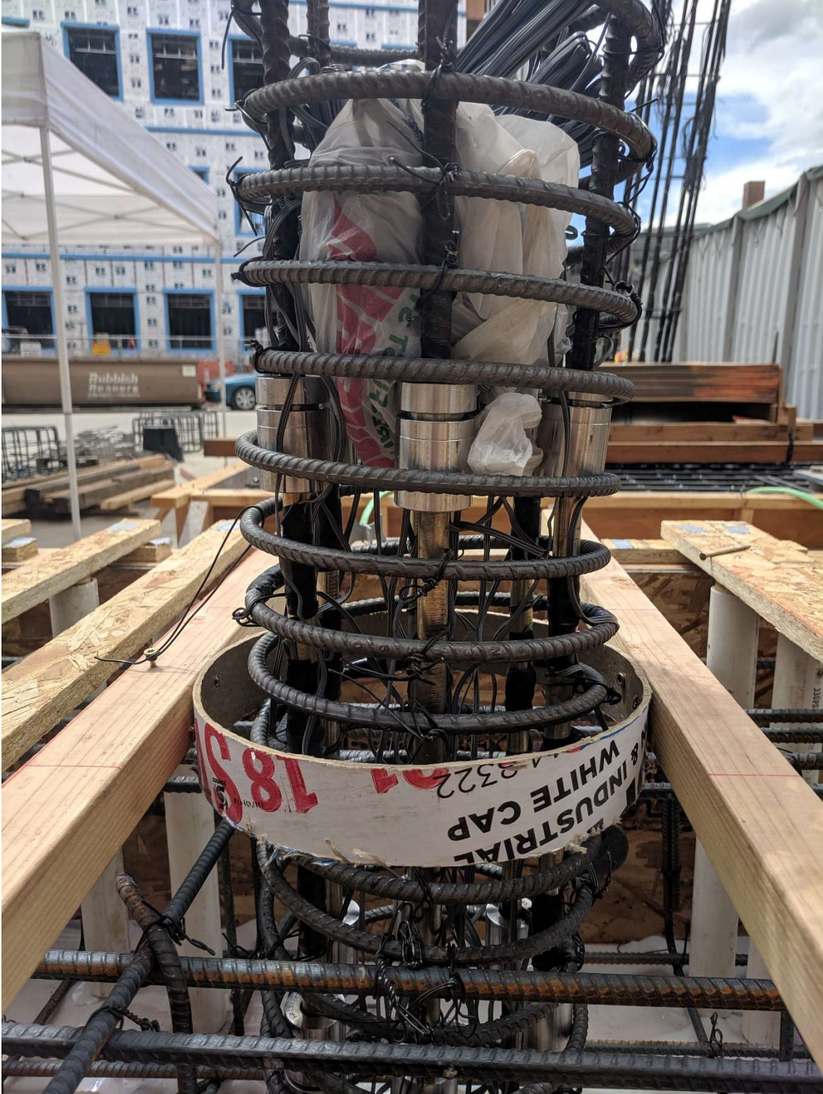
Figure 2.31 CAM bars HRC coupled to #4 rebar within hinge spiral
