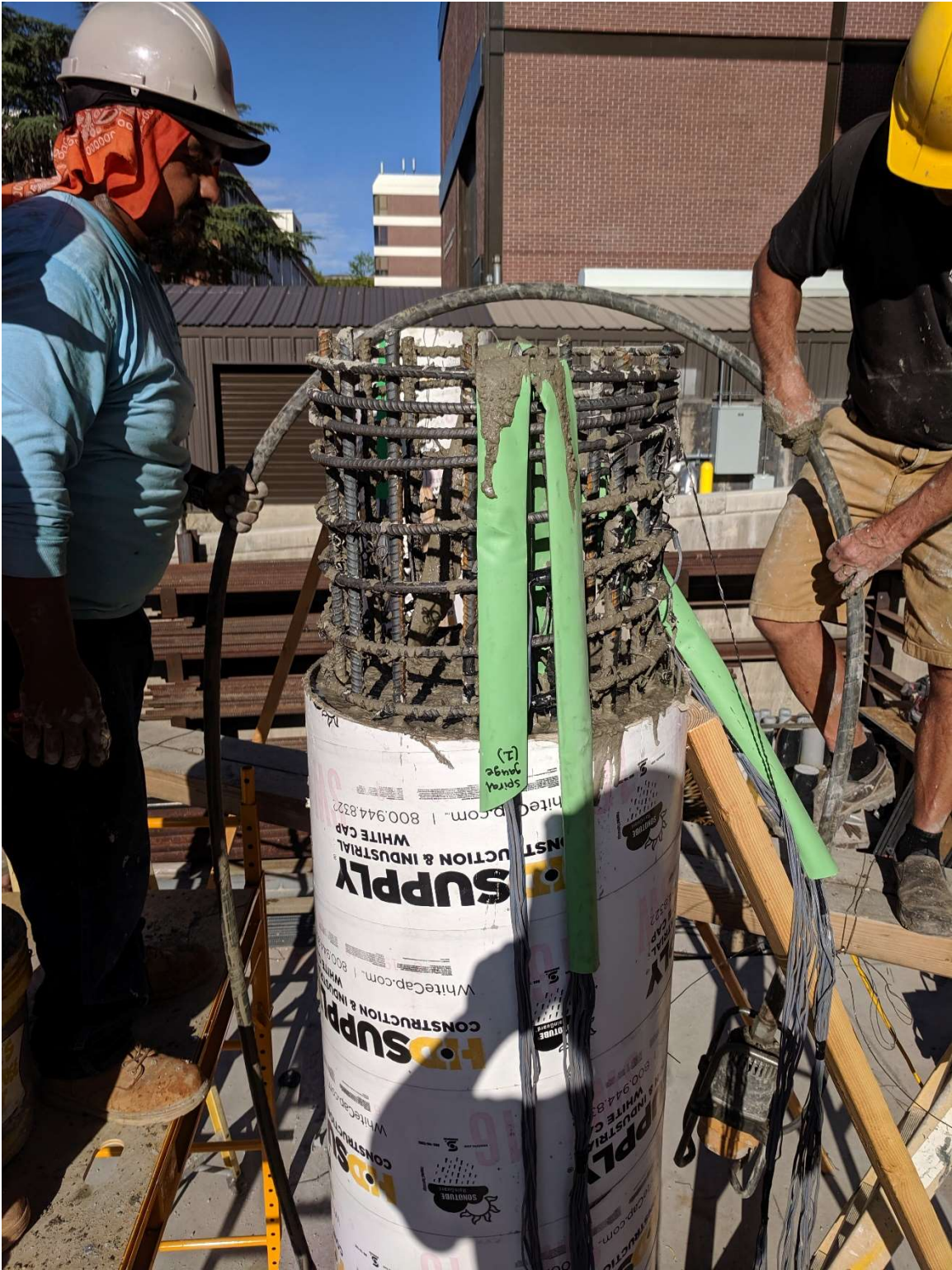
Figure 2.42 Pouring and vibrating of column concrete
