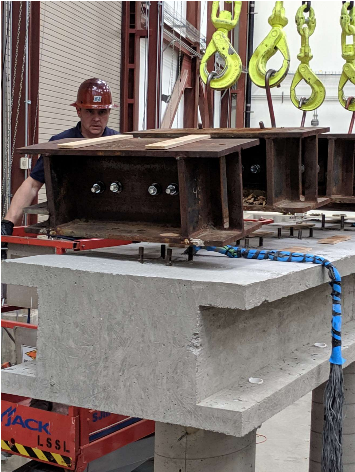
Figure 4.12 Placement of load transfer beam onto specimen cap beam
