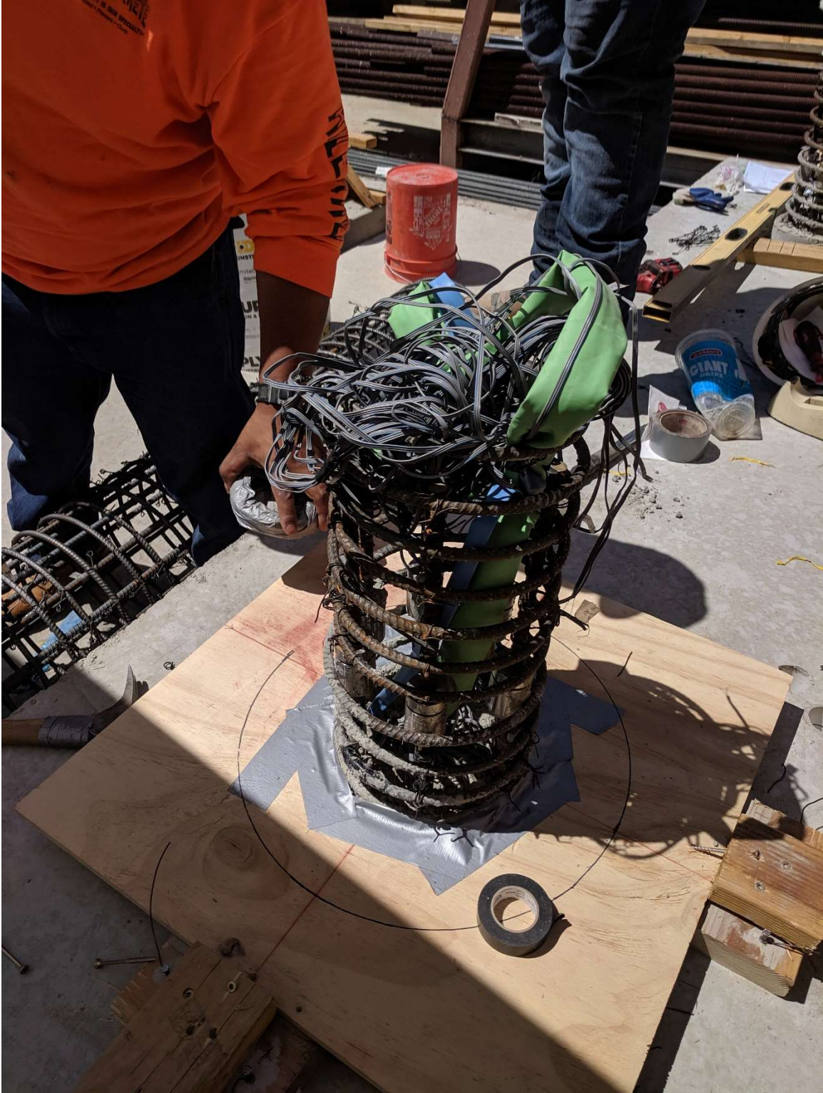
Figure 2.39 Wooden platform to elevate column
