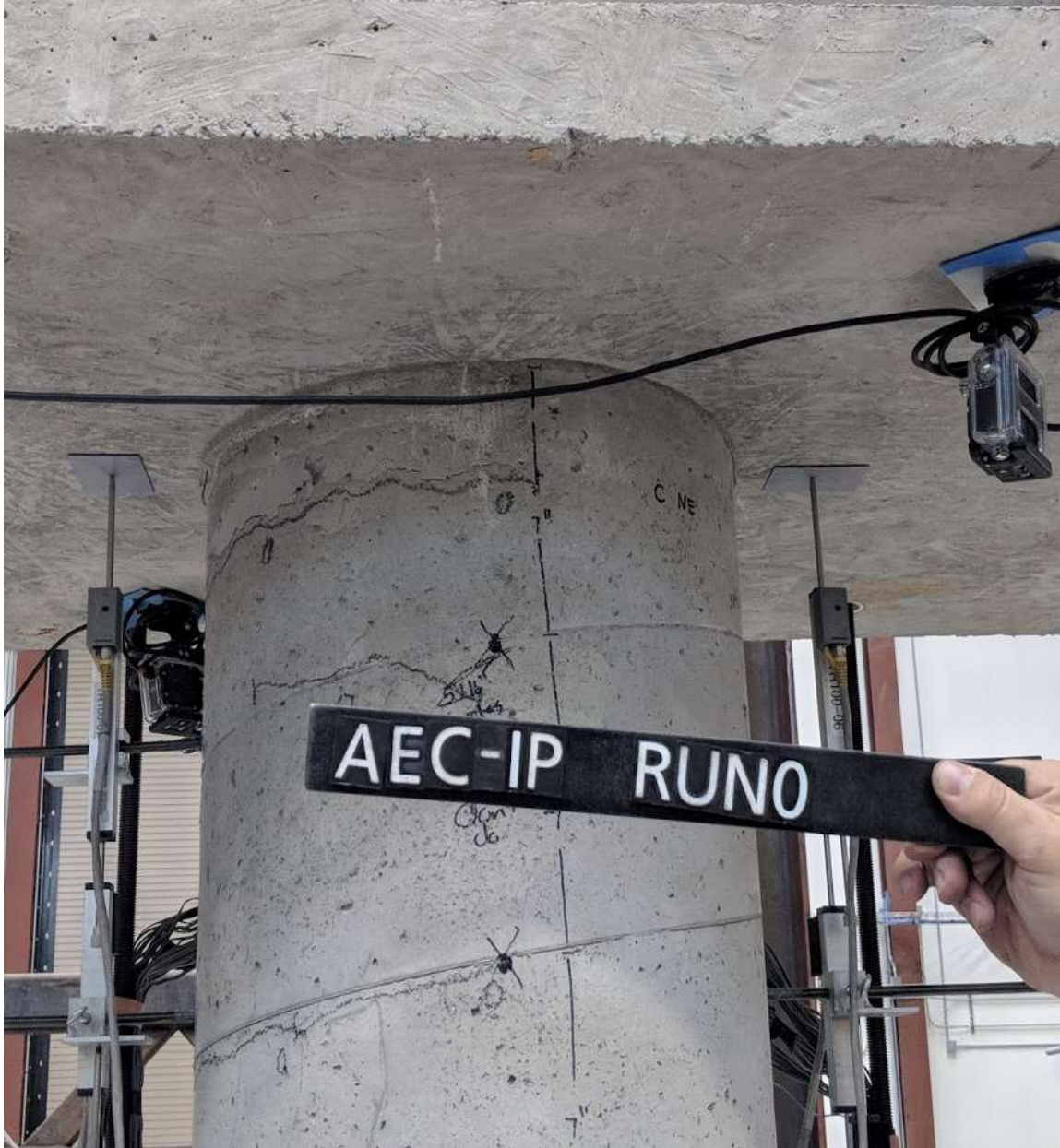
Figure 5.24 Run 0 – Cracks marked before testing (CIP – E face)
