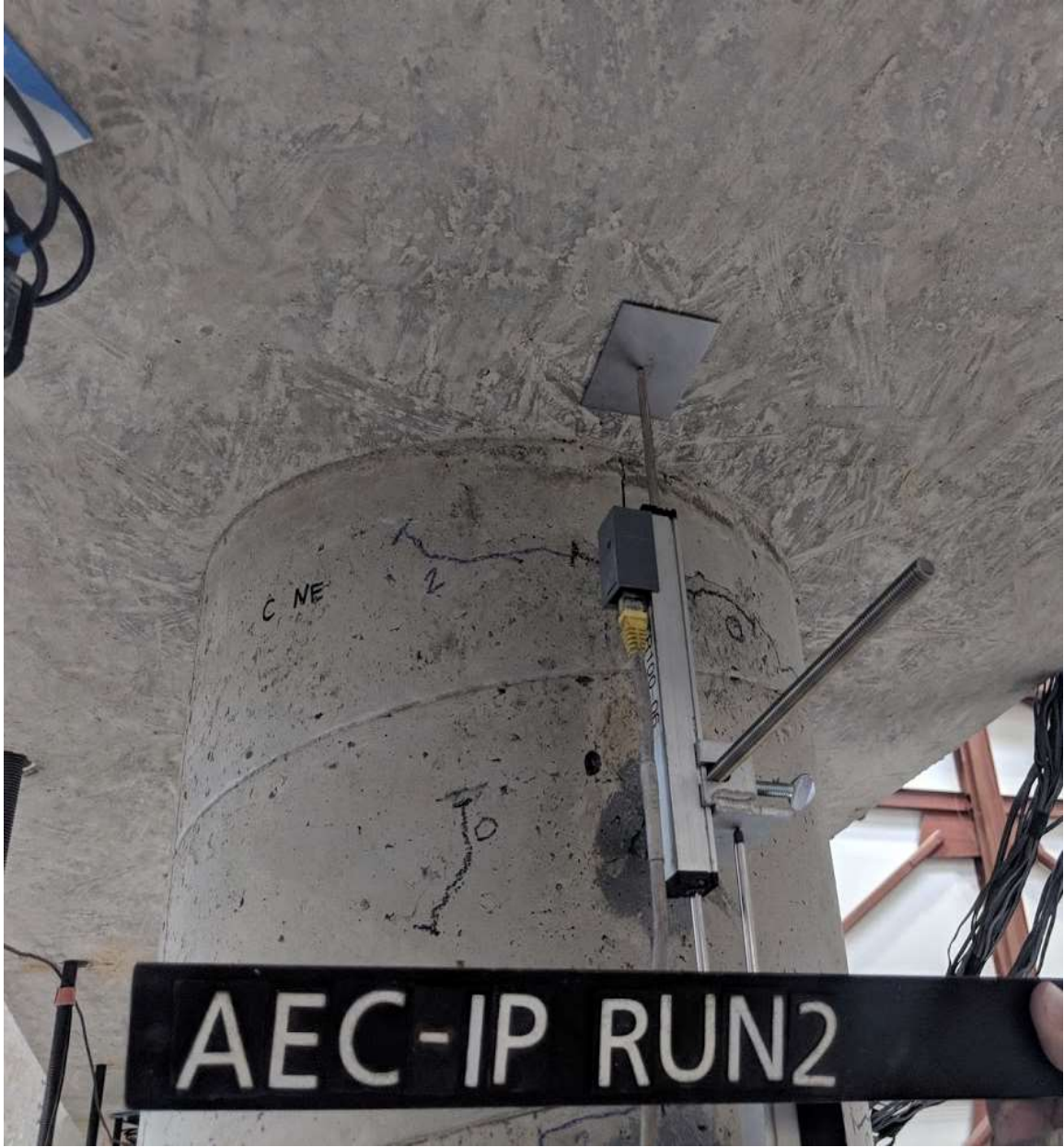
Figure 5.27 Run 2 – Extension of pre-existing cracks (CIP – N face)
