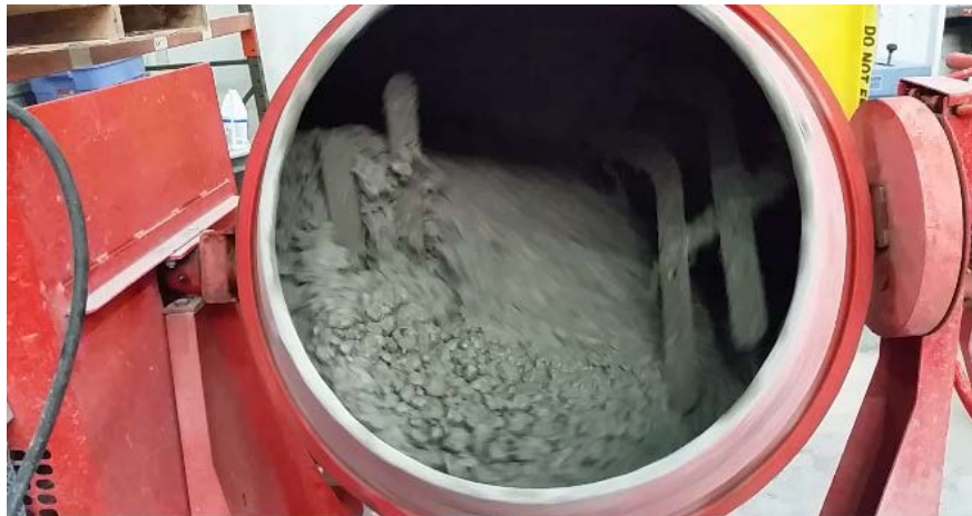
Figure 15. Photo. Concrete Mixing From (Shalan 2016)
