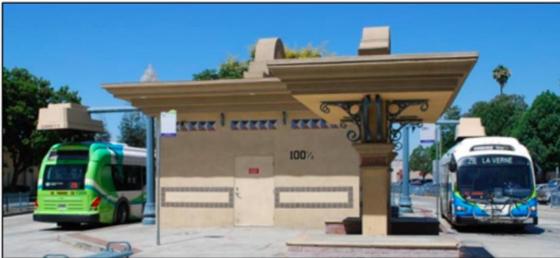
Figure 12. Charging station for the Proterra Bus [20]
