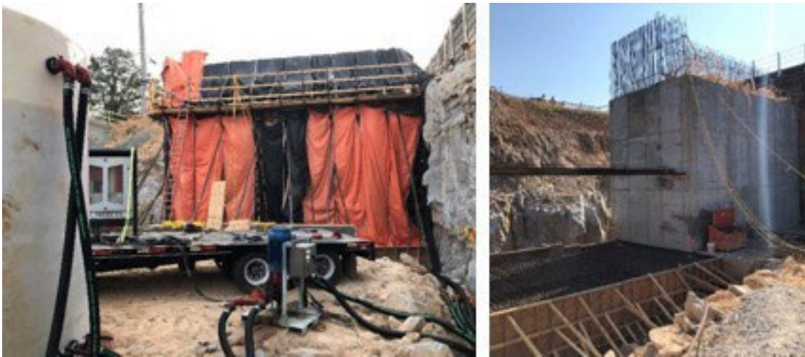
Figure 51. Photo. SR-92 abutment wall and footing.
