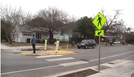
Figure 3.3 Concrete refuge island with flexposts at North Loop & Chesterfield
