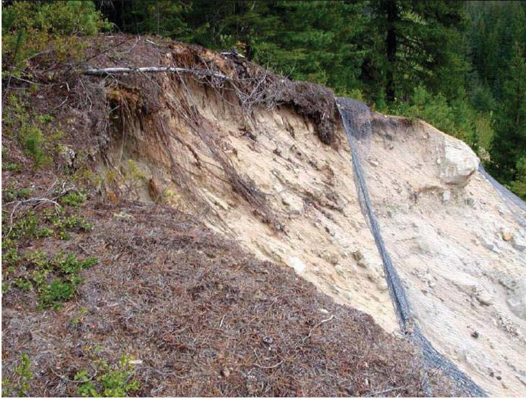
Figure 59. Photo. Erosion can lead to failure in a drapery system if the mesh is not secured sufficiently beyond the area of slope degradation at the top of the slope.
