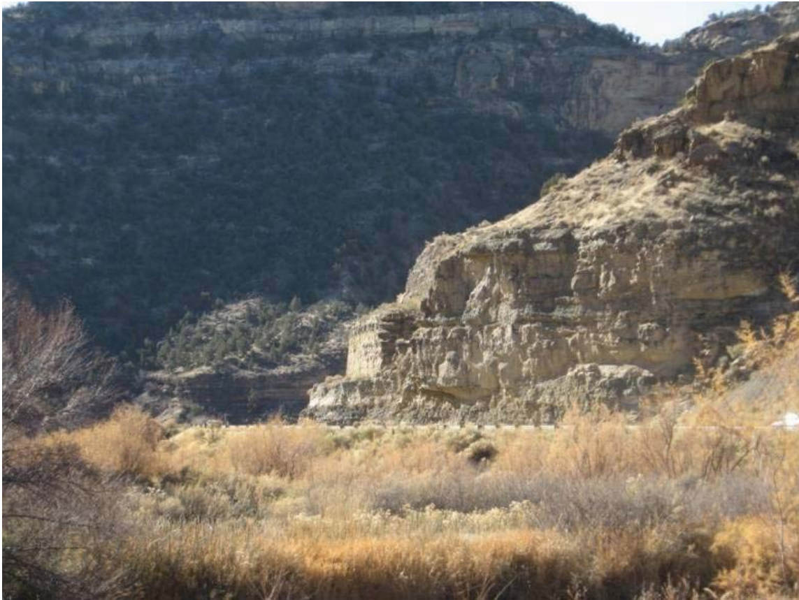
Figure 33. Photo. Slope angle variation helps match the natural topography of the surrounding area. The lower three tiers in the slope were excavated to simulate the natural benches in sedimentary units.
