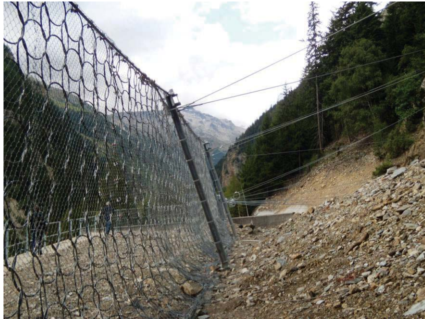
Figure 68. Photo. Example of a ring-net flexible barrier.
