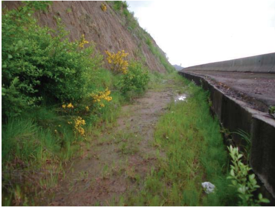
Figure 72. Photo. A hybrid ditch design.
