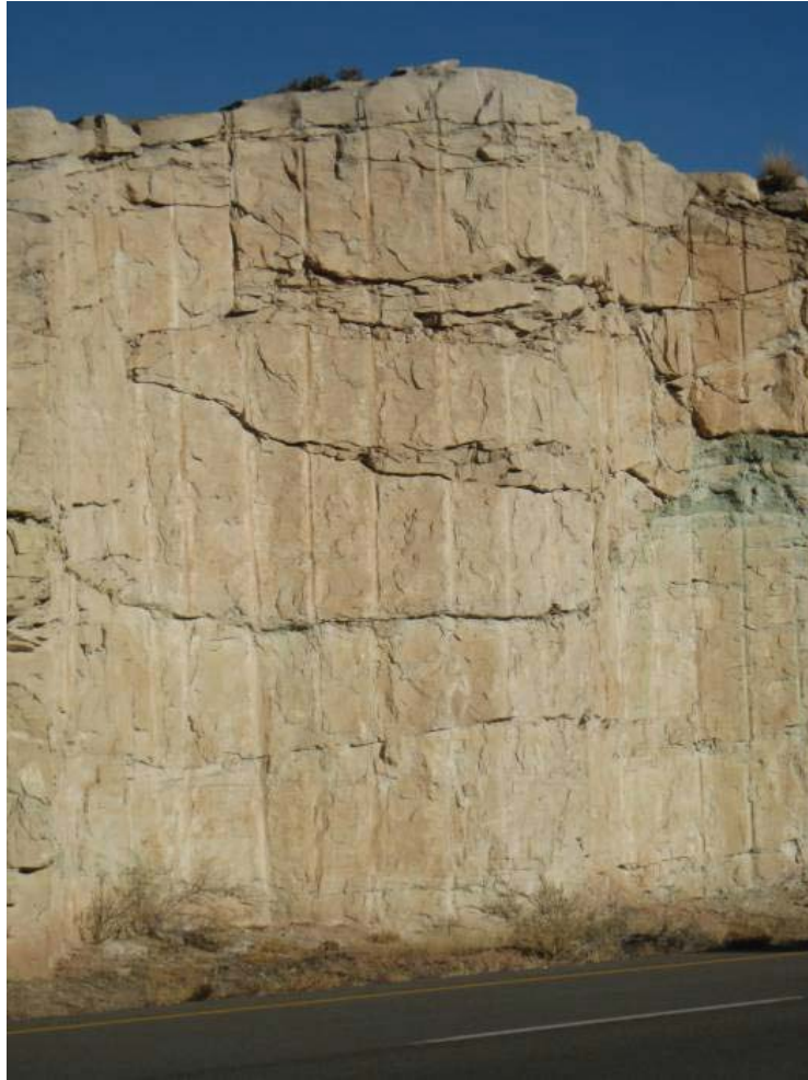
Figure 12. Photo. Example of a presplit slope in massive sandstone. Note the abundant drill hole traces (half casts).
