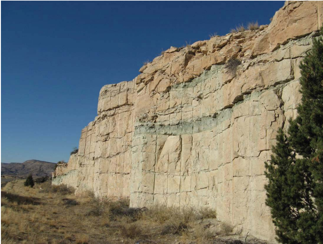
Figure 32. Photo. Ditch width variation can camouflage blast scars and drill traces.
