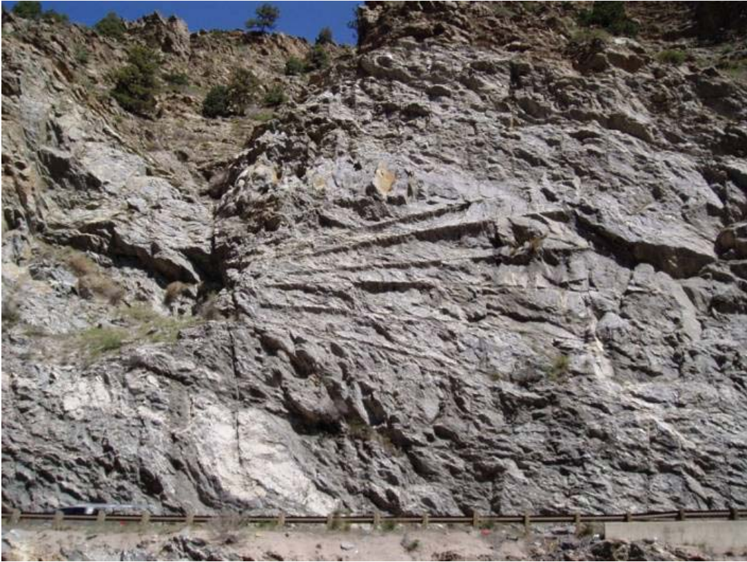
Figure 17. Photo. Drill hole traces left by horizontal drilling parallel to the rock face (fan drilling).
