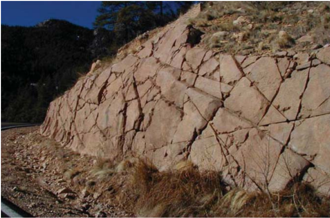
Figure 51. Photo. Shotcrete can be used to protect a slope from erosion—and sculpted to mimic the natural rock face (Ada County Highway District 2003).
