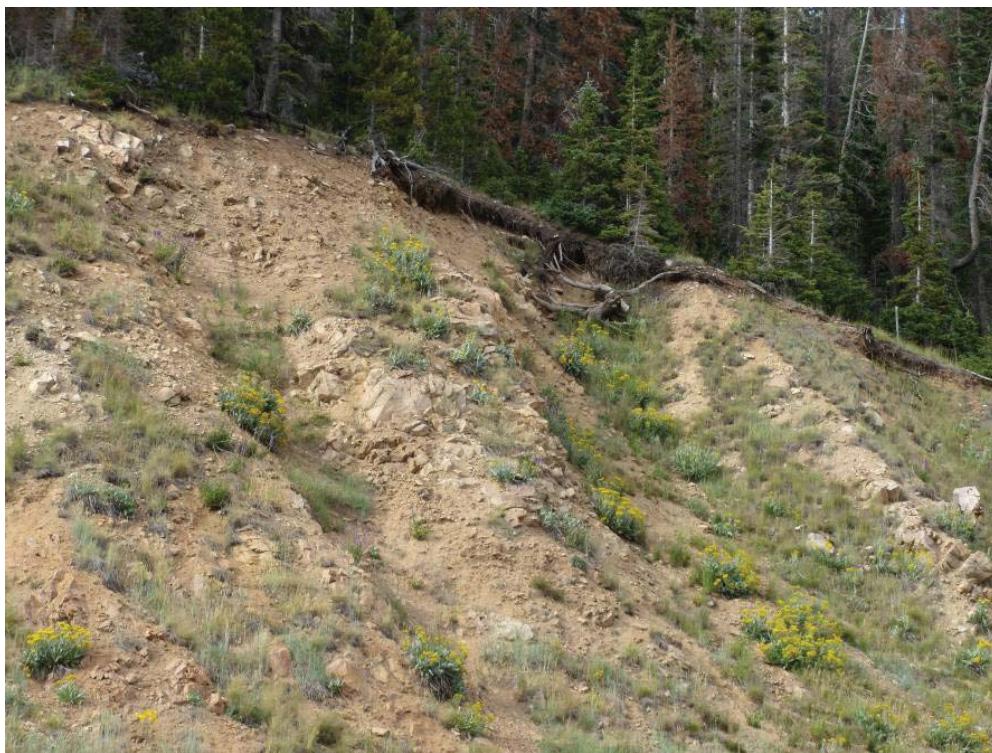
Figure 29. Photo. Expanded slope rounding can prevent this type of erosion and overhang.
