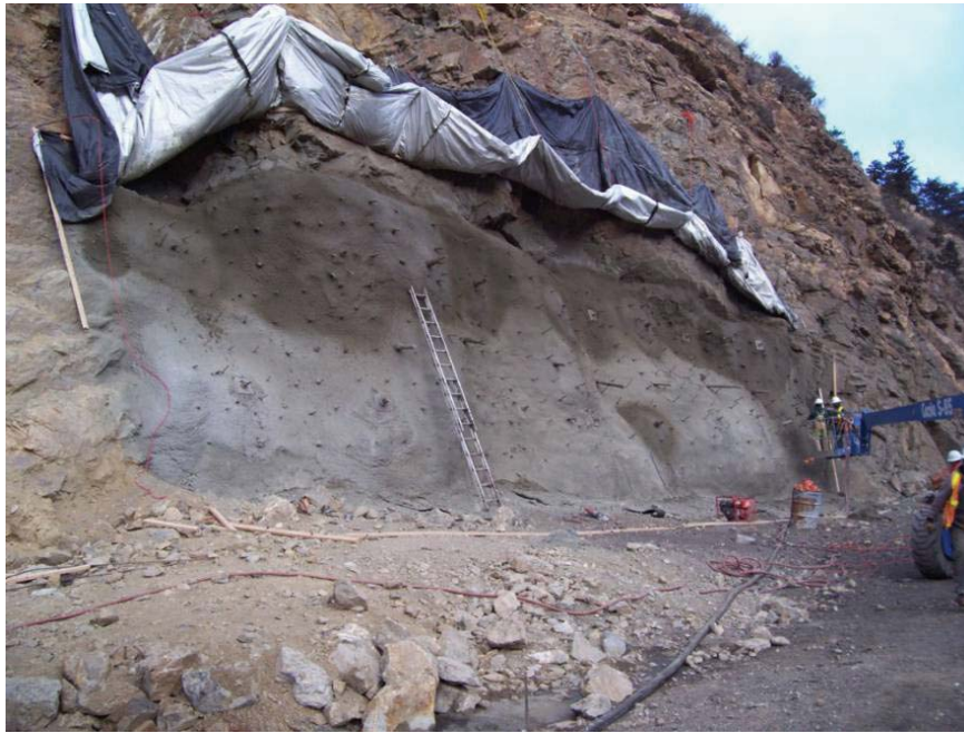
Figure 54. Photo. Installation of the first layer of structural shotcrete.
