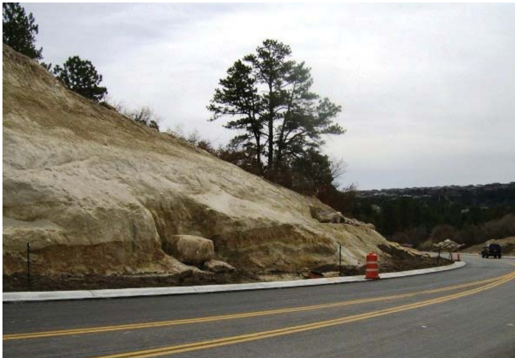
Figure 26. Photo. Completed rock slope prior to placement of topsoil and a native seed mix.
