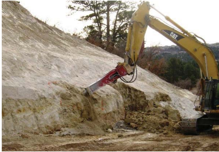
Figure 25. Photo. A hydraulic hammer expanding a sculpted area, creating planting areas and more natural-looking slope variation.
