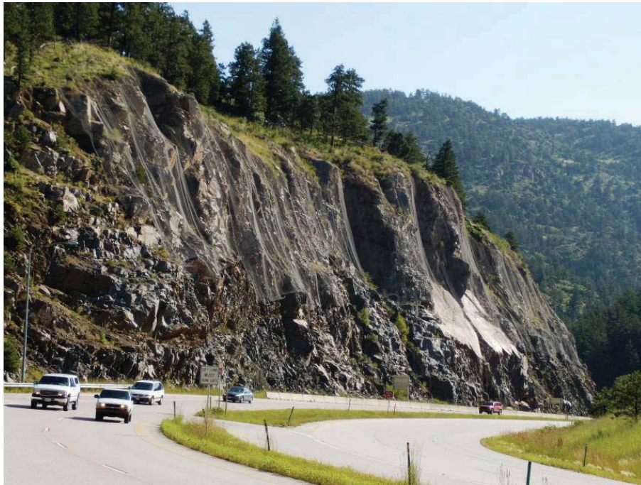
Figure 61. Photo. A drapery system that was not visually mitigated.
