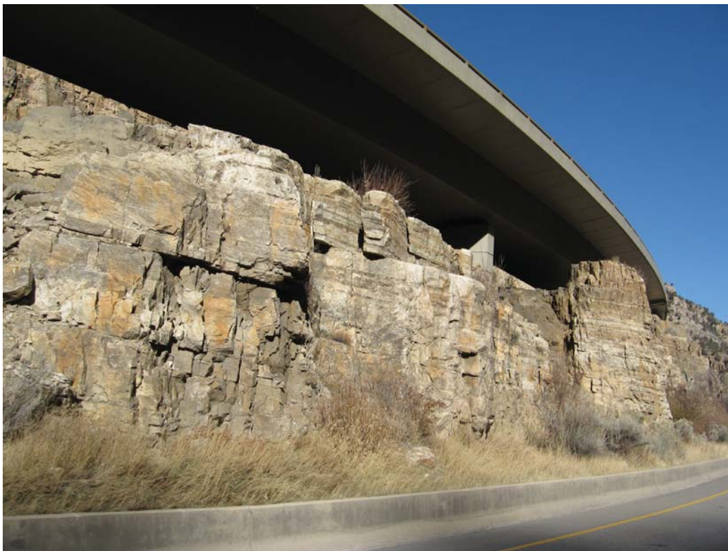
Figure 37. Photo. Staining on the completed cut slope used to create a natural-looking rock face. Glenwood Canyon, Colorado.
