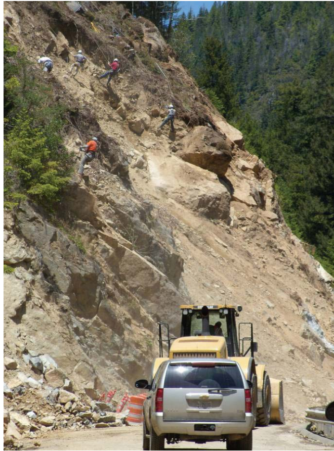
Figure 39. Photo. Hand scalers removing loose material from a cut slope South Fork Smith River Road, California.
