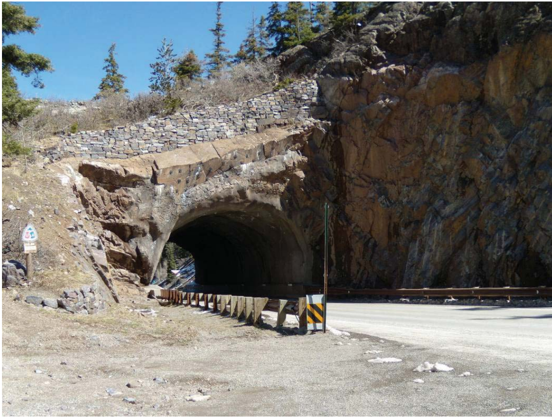
Figure 52. Photo. Sculpted shotcrete used to stabilize a tunnel portal (the area directly below the dry-stack wall is the sculpted shotcrete).
