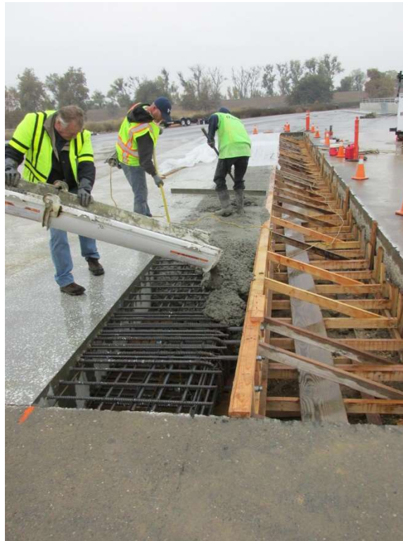
Figure 2-13. Concrete Deck Overhang Pour
