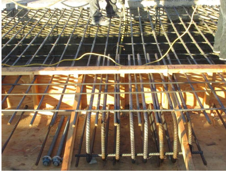
Figure 2-8. Rebar Configuration at Rail Post Location
