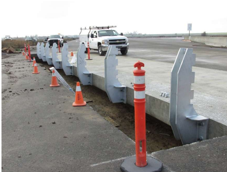
Figure 2-15. Installation of CA ST-70SM Side Mounted Bridge Rail Posts
