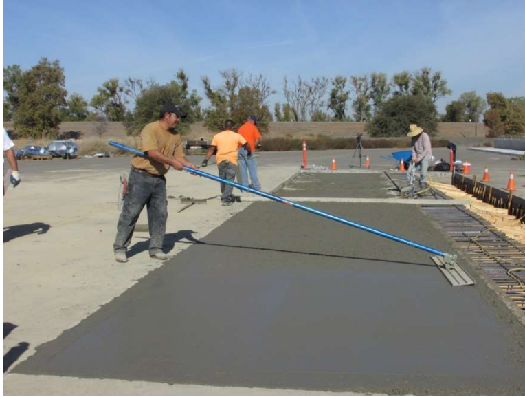
Figure 2-10. Surface Finishing on Anchor Block
