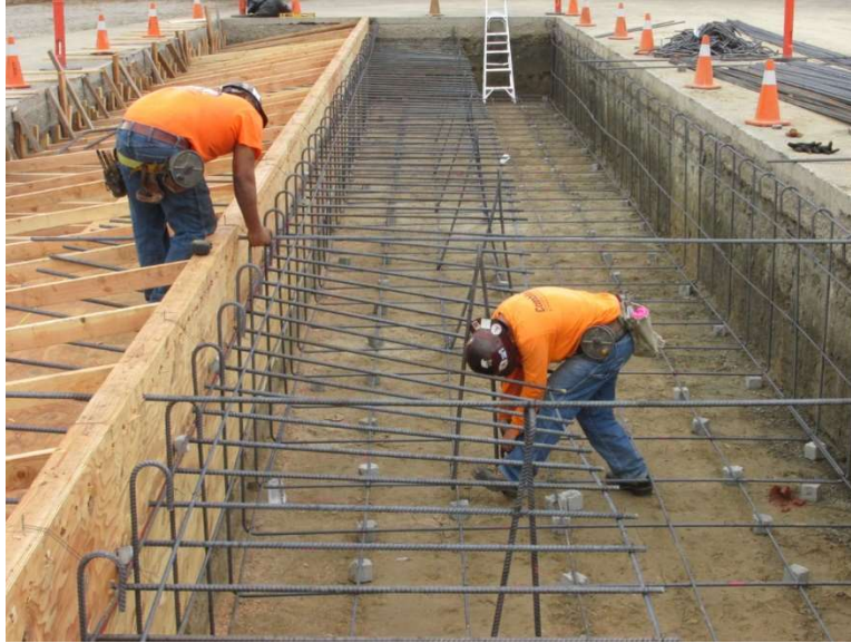
Figure 2-4. Anchor Block Rebar
