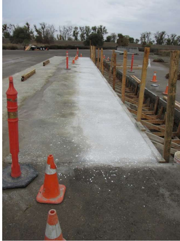
Figure 2-14. Concrete Deck Overhang Finish
