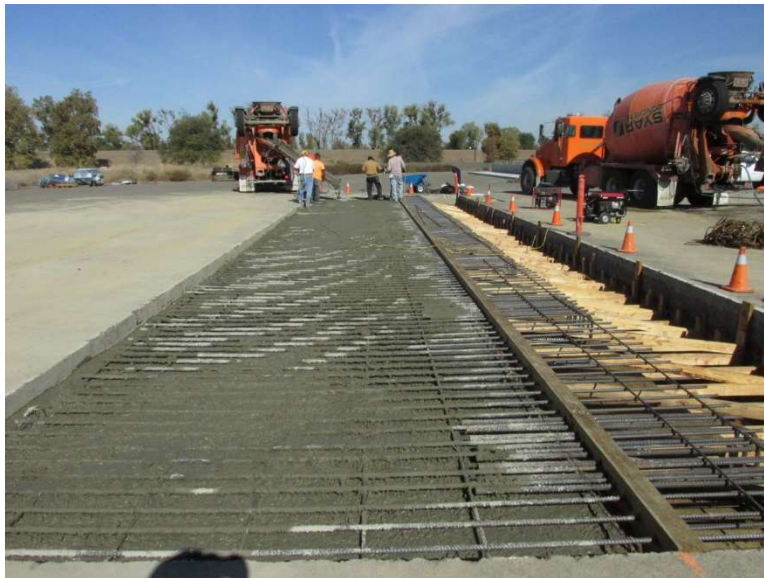
Figure 2-9. Pouring Anchor Block Concrete
