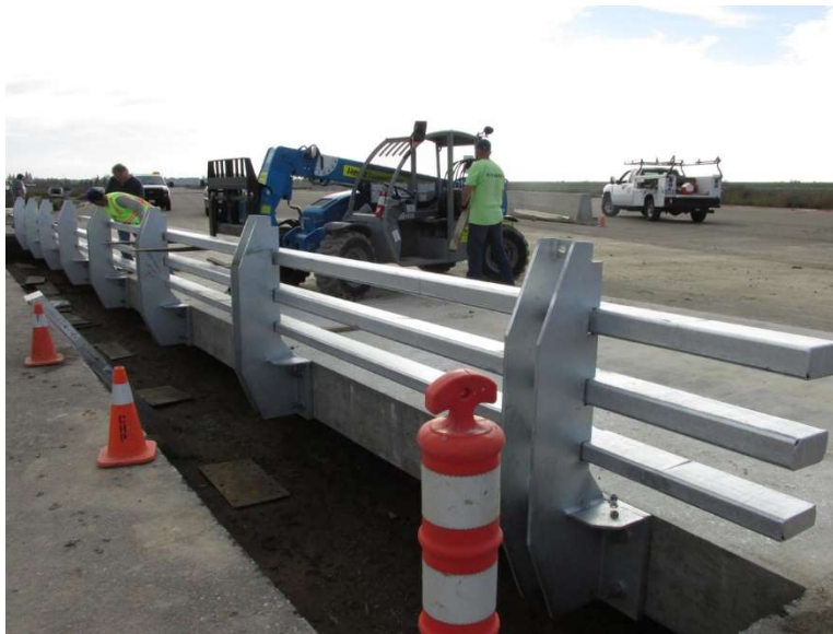
Figure 2-16. Installation of CA ST-70SM Side Mounted Bridge Rails
