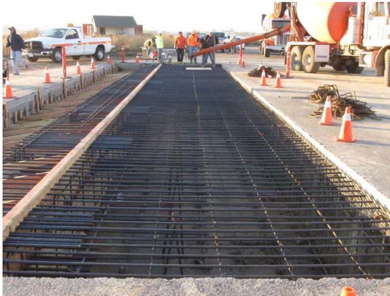
Figure 2-7. Anchor Block and Bridge Deck Rebar
