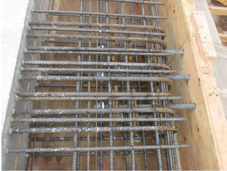
Figure 2-12. Anchor Rod Placement in Deck Overhang
