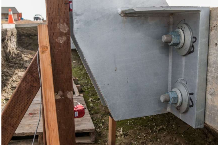
Figure 3-22. Disc Spring Installation
