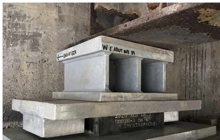
Figure 2.3: Bridge bearing in use (MassDOT)
