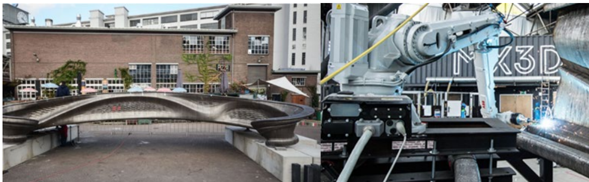
Figure 1.6: MX3D 3D-printed stainless steel bridge
