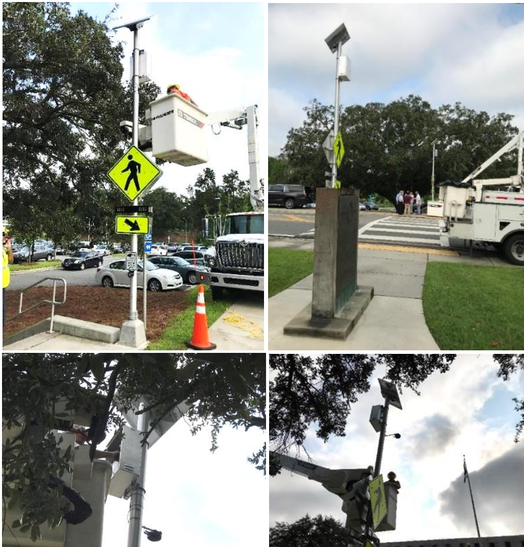
Figure 38. Installation of system at midblock crosswalk, Tallahassee
