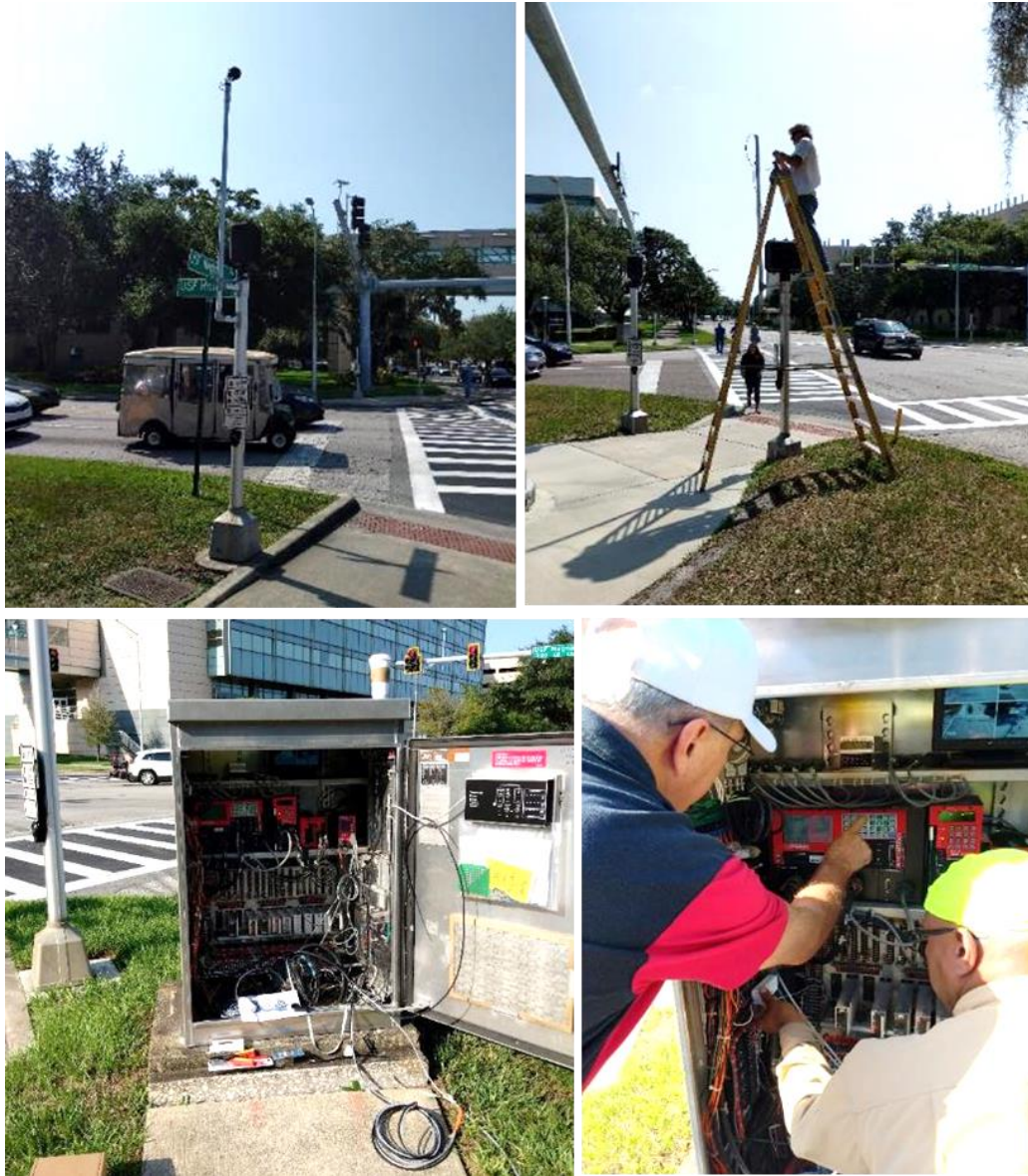
Figure 40. Installation of system at signalized intersection, Tampa
