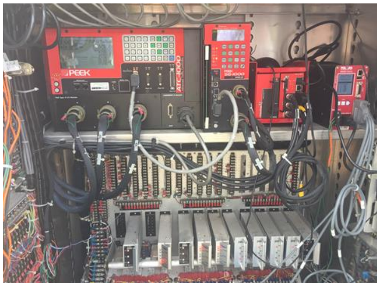
Figure 50. Integration of programming script into traffic signal controller
