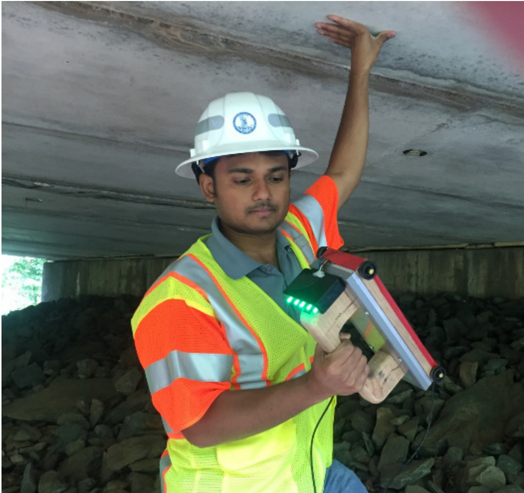
Figure 27. MFLIS Device Being Used by Inspector. MFLIS = magnetic flux leakage inspection system.
