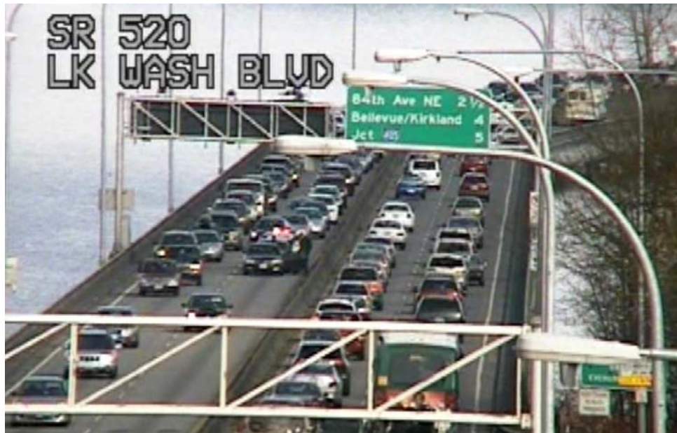
Figure 6-5. Apr. 9, 2010, Downstream of Incident
