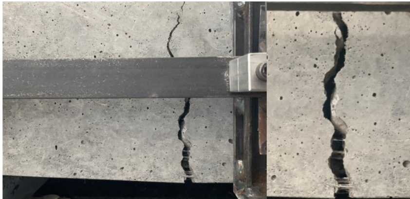
Figure 3-18. Fibers Bridging a Crack
