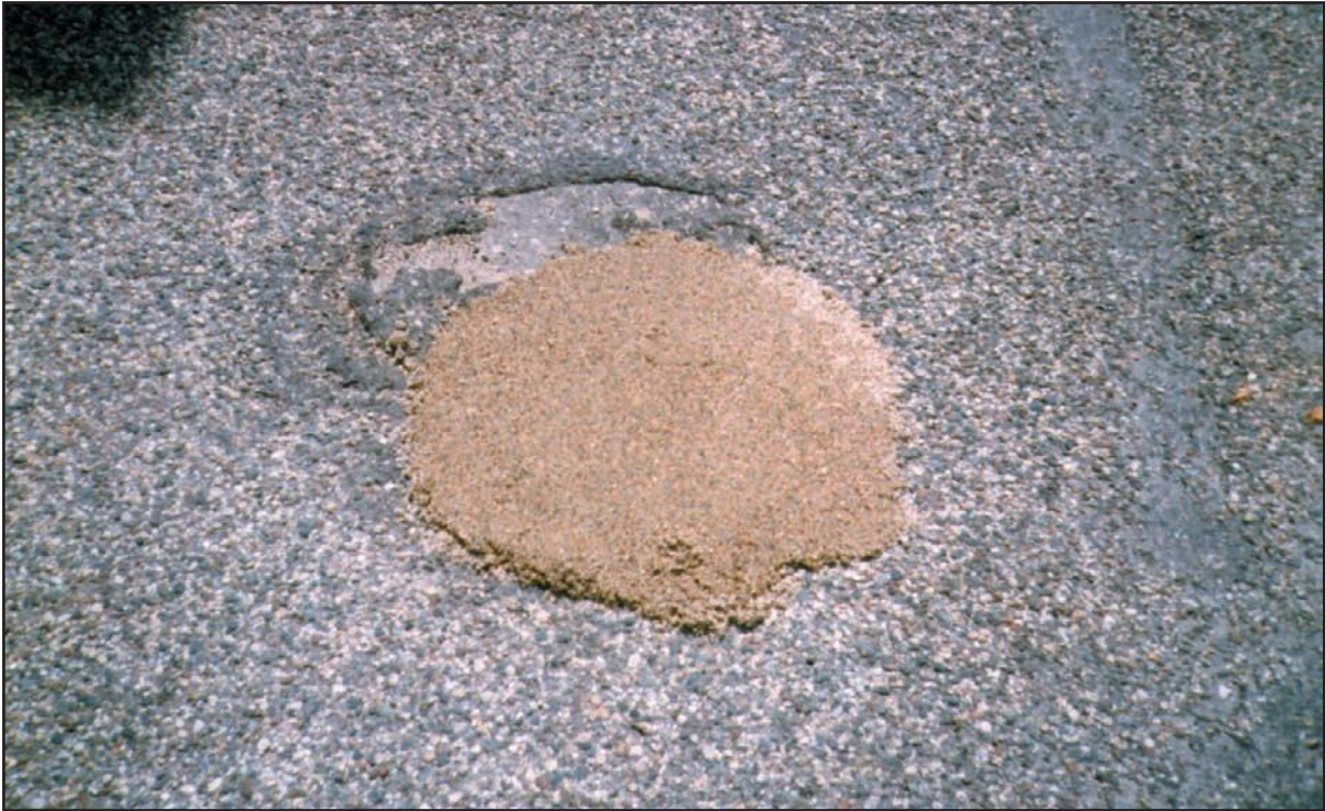
Figure 3.8.23. Sand cover on manholes
