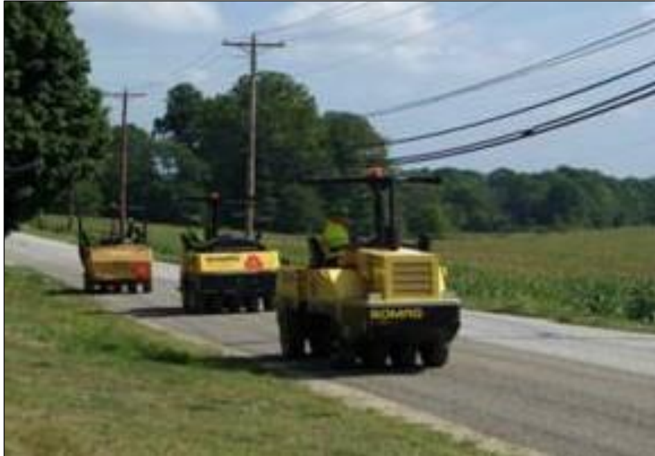
Figure 3.1.8. Pneumatic tired rollers (Ohio DOT)
