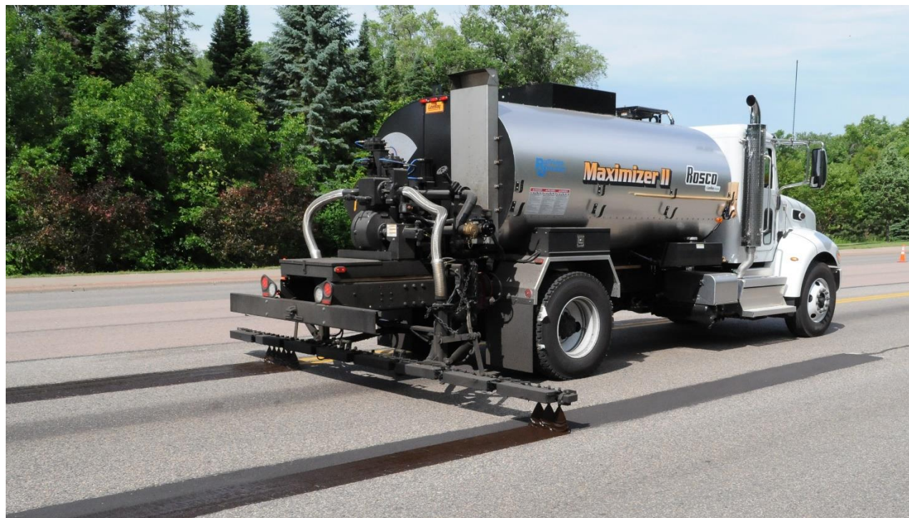
Figure 3.8.21. Pretreatment of pavement markings
