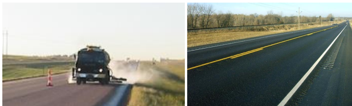
Figure 3.5.1. Fog sealing after chip sealing
