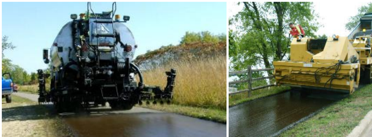
Figure 3.6.1. Chip sealing of recreational trail
