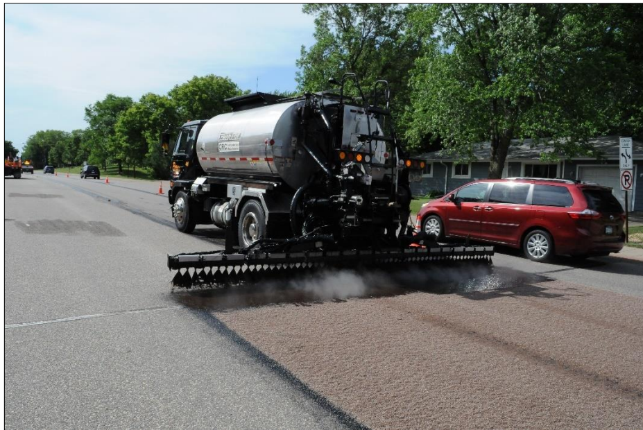
Figure 3.1.5. Computer controlled asphalt distributor
