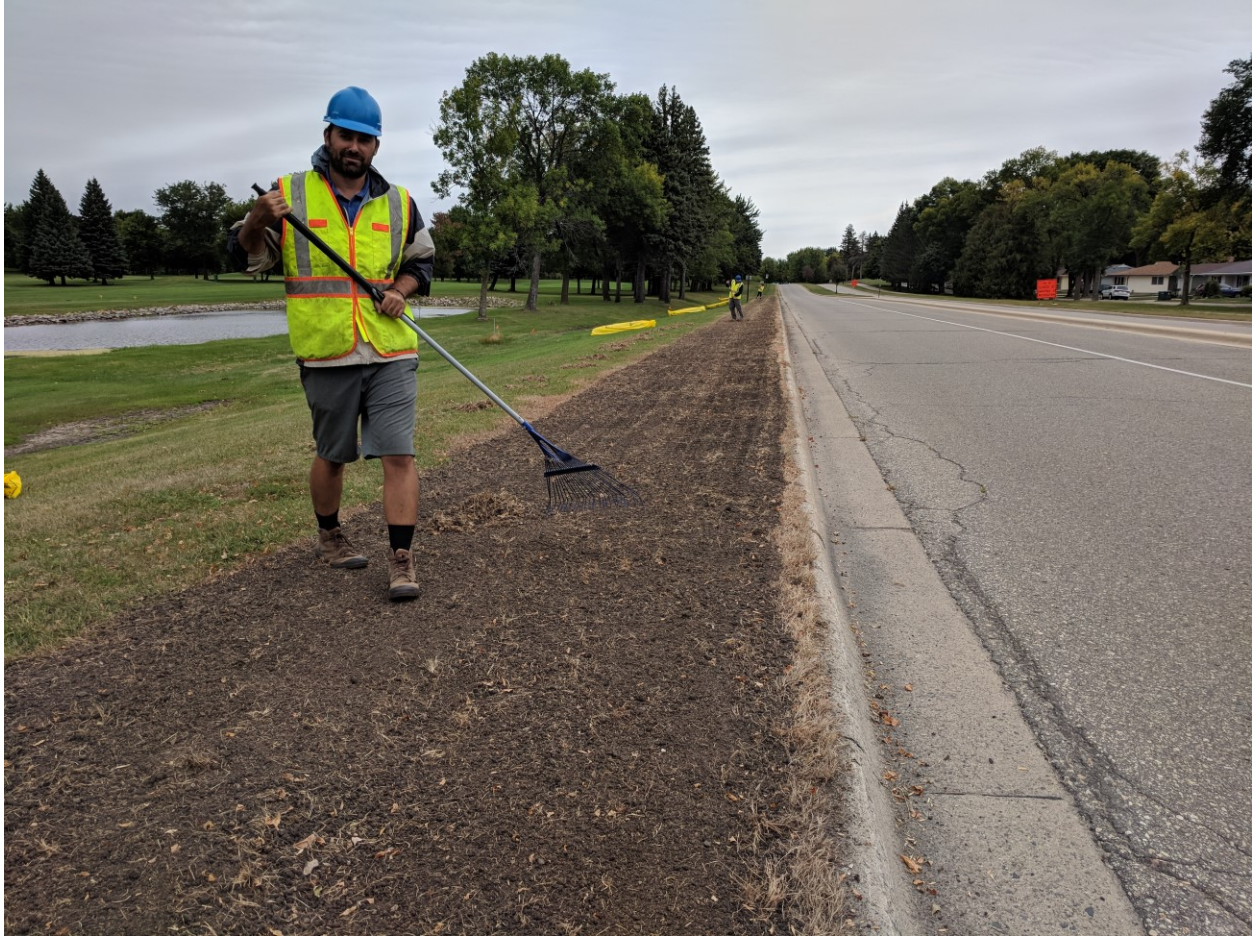
Figure 2.2 Dr. John Trappe preparing soil bed before seeding. This photo was taken at the Marshall, MN roadside research site on Sep. 17, 2018.
