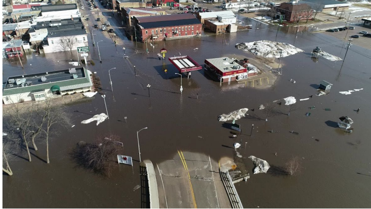
Figure 30. Photo. Flooded road – Library sample image. (35)
