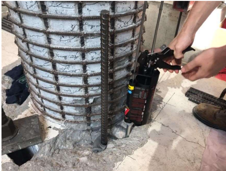
Figure 3.7: Anchorage of Repair Bars in Footing via Epoxy.
