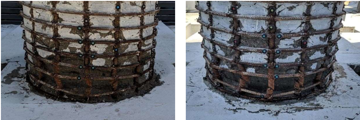
Figure 4.12: Damaged column for Repair #2 on the North (left) and South (right) sides.
