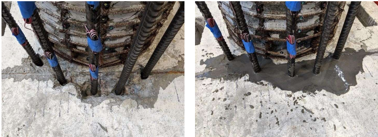
Figure 3.8: Use of Grout to Provide a Level Base for the Steel Sleeve.
