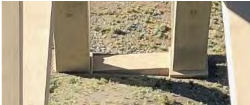
Figure 2-15: Link beam connecting the northbound and southbound superstructures
