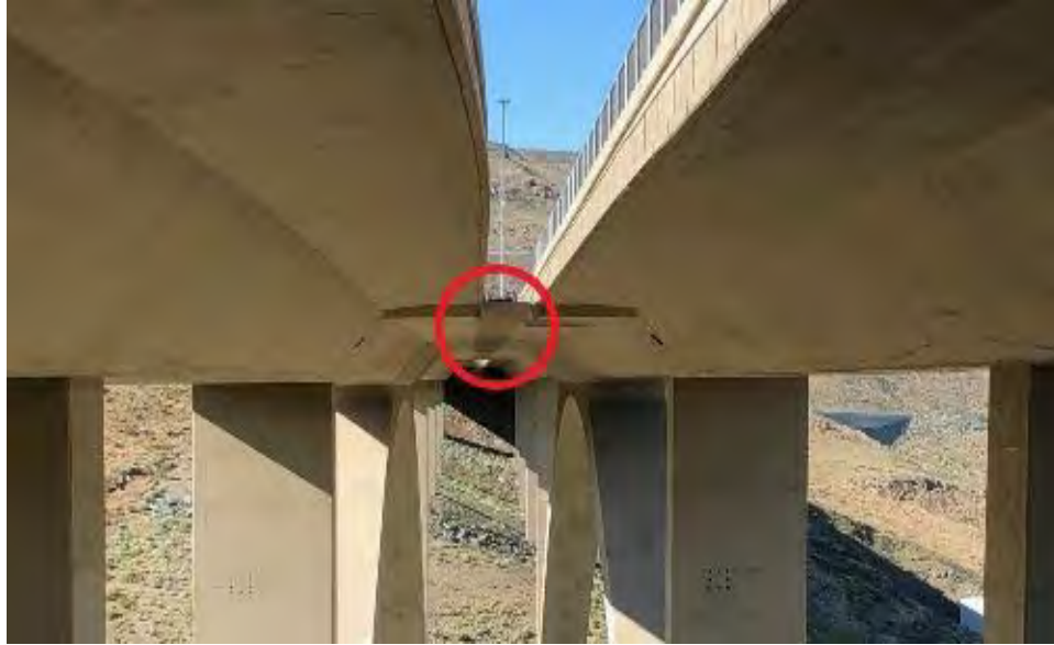
Figure 2-13: Hinge diaphragm elevation view (m)
