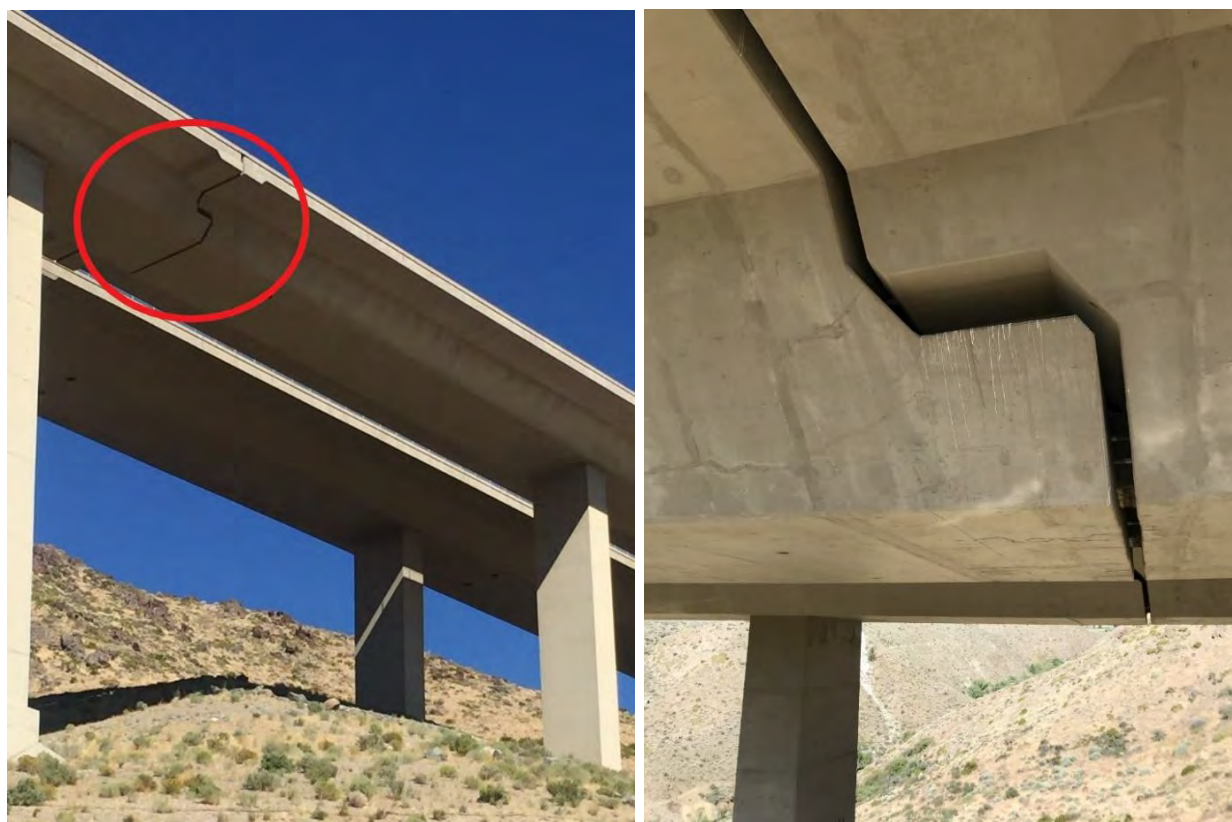
Figure 2-10: Photographs of Galena Creek Bridge expansion joint hinge
