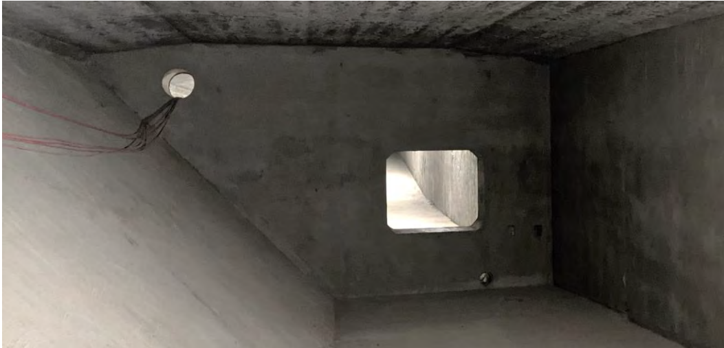
Figure 2-11: Example of Galena Creek Bridge diaphragm
