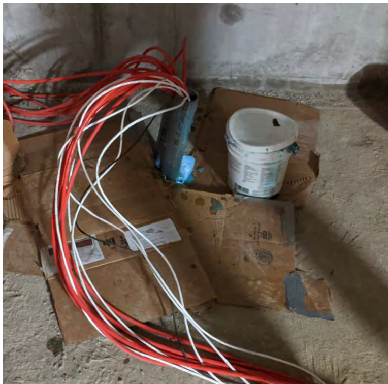
Figure 3-8: PVC conduit extruding through the bottom slab near Abutment 1
