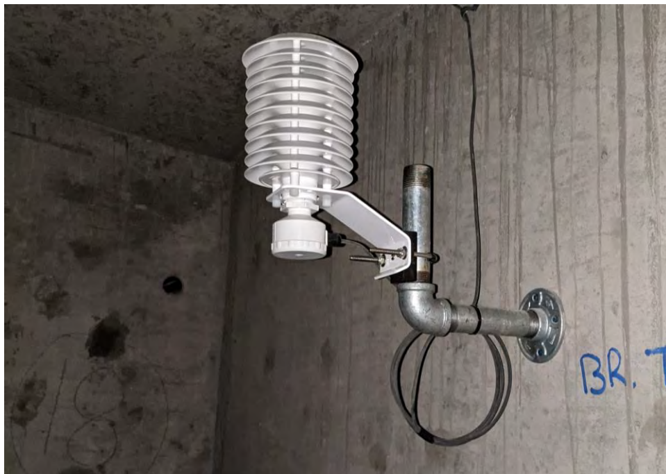
Figure 3-15: Temperature probe located in Galena Creek Bridge
